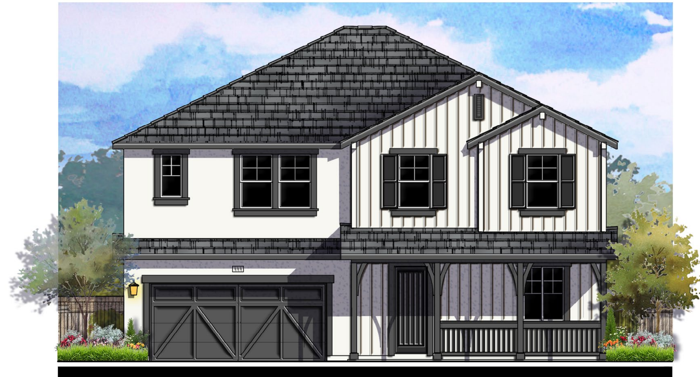
© 2020 Kevin L. Crook Architect, Inc. Refer to landscape drawings for wall, tree, and shrub locations
