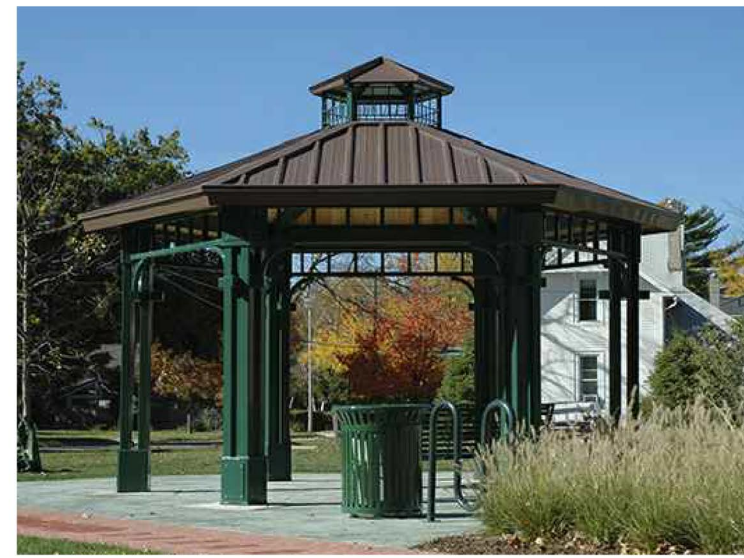
OVERHEAD SHADE STRUCTURE
