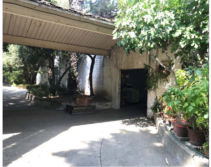
Image 14. View of west elevation of Warehouse A building (Resource No. 7) showing breezeway connection.
