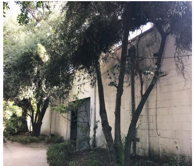
Image 16. View of west elevation of Warehouse C building (Resource No. 9).
