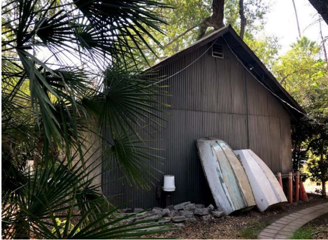
Image 17. View of north elevation of the Graber Barn building (Resource No.10).
