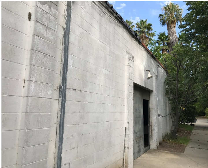
Image 15. View of east elevation of Warehouse B building (Resource No. 8).
