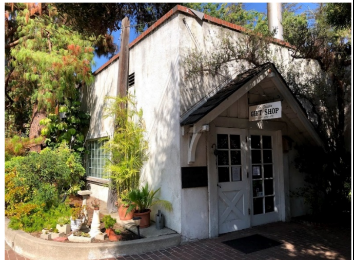
Image 12. View of the southwest corner of La Casita Gift Shop building (Resource No. 4).
