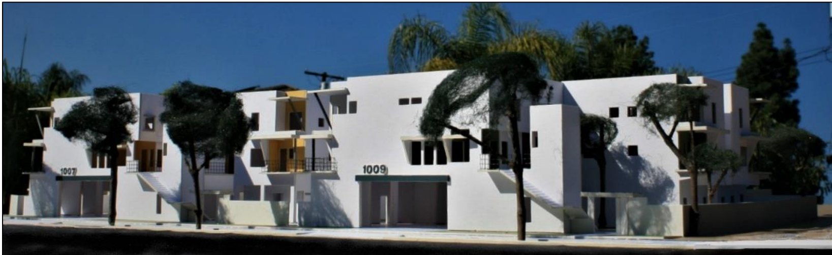
South Elevation (Facing Sixth Street – From Southeast Corner)
