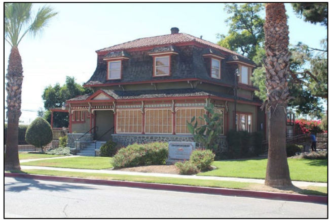
West Elevation (enclosed porch and mansard roof 2016)
