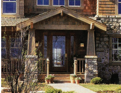
Front Porch with Battered Columns
