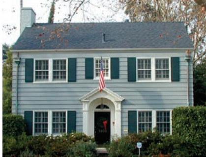
Vertical Multi-Pane Windows with Shutters
