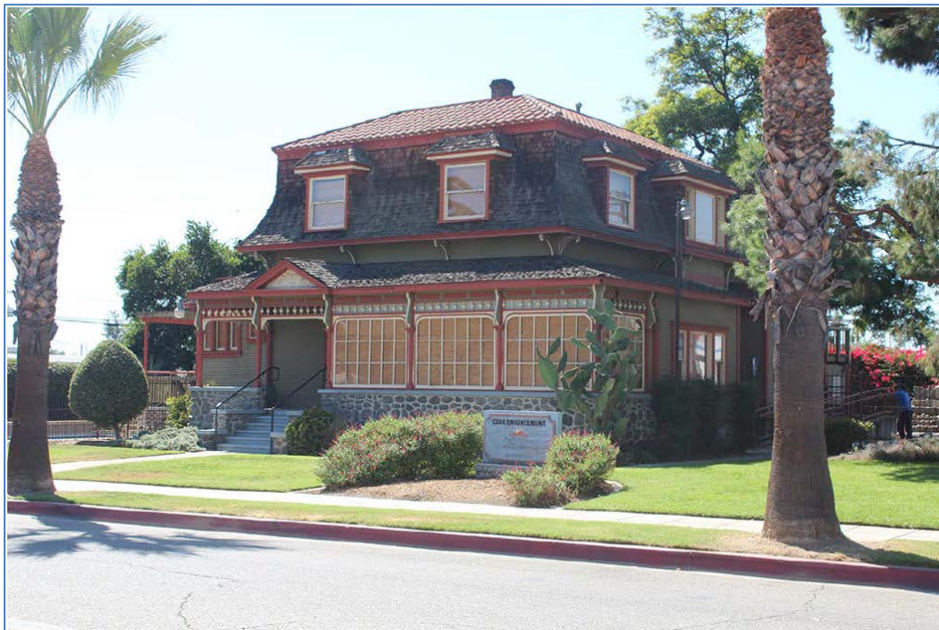
South Vine Ave- Front Façade (southwest view)
