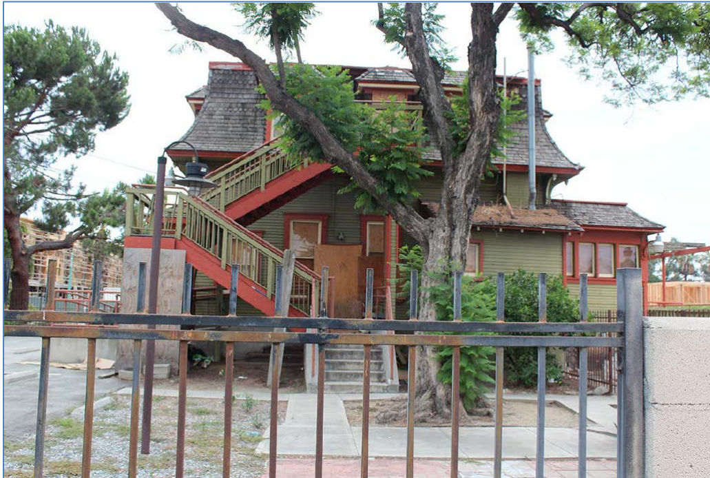
West Elevation- Rear (view from alley)
