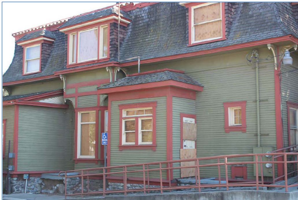
North Elevation- Side (view from parking lot)
