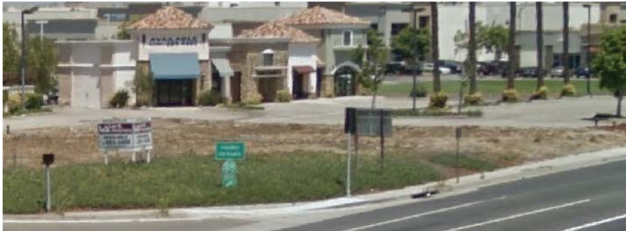
Northwest View of Existing Building
