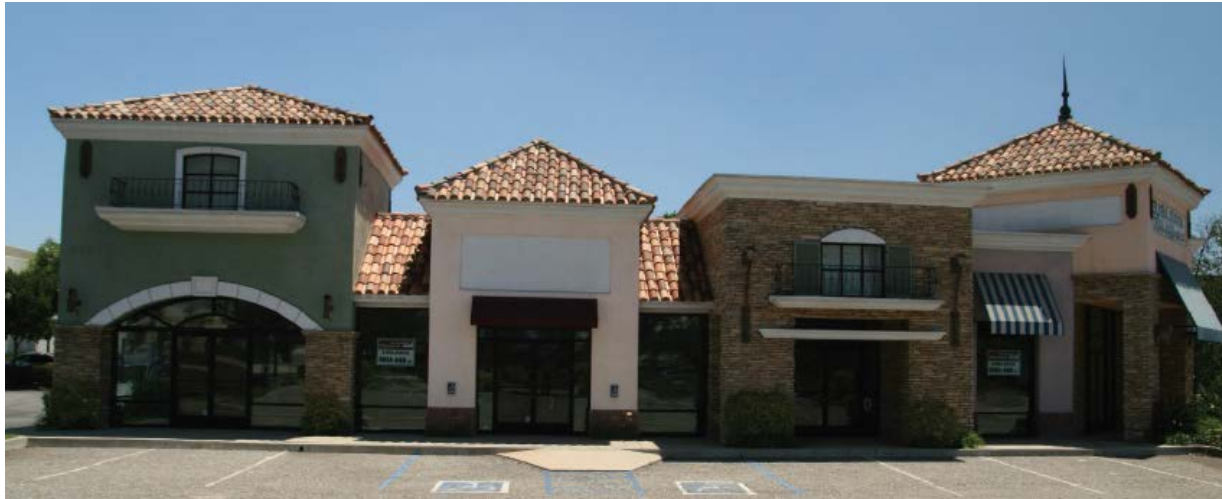
View of Building's East Elevation
