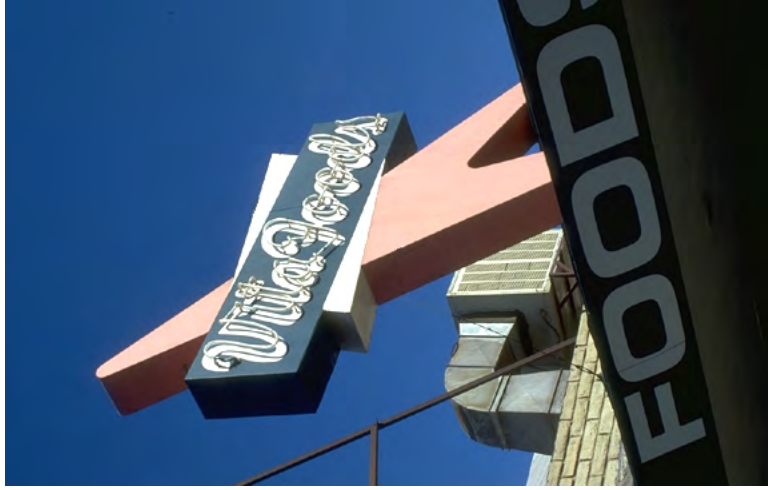
An example of a 1950's style partially roof mounted sign with the largest portion of the design above the roof line.
