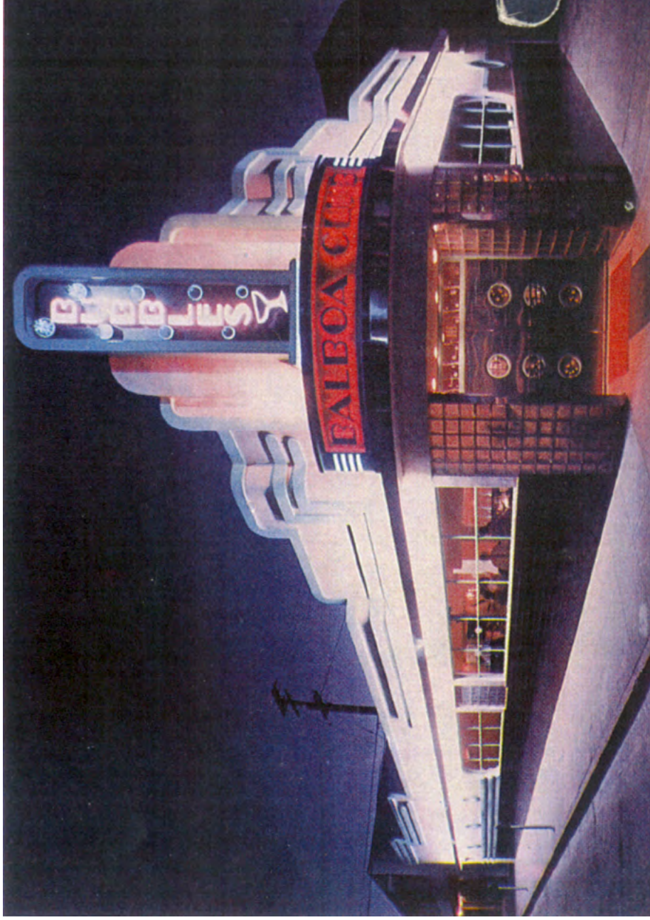
Example of a lit building from the 1920's - 40's time-period. Note the concealed lighting along the facade moldings, neon and internally lit signs.
