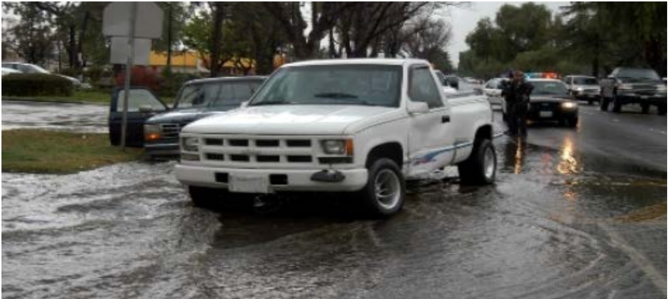
Figure 4-5: An intersection in Ontario is flooded after a storm
