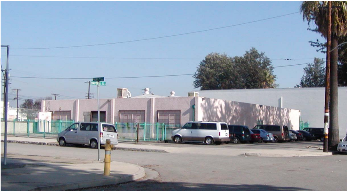
Photograph 2.2.5 The Exterior of the Montalvan Building Facing Northeast on Euclid Street
