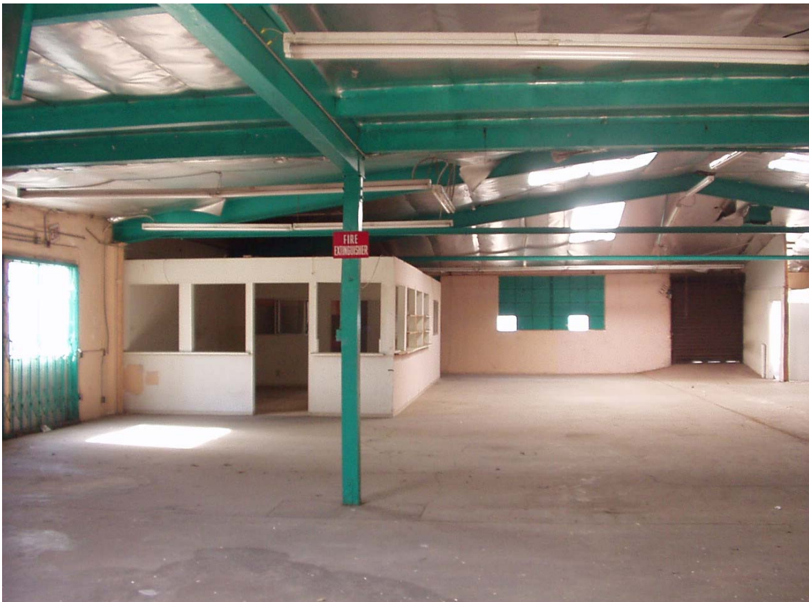
Photograph 2.2.6 The Interior of the Montalvan Building
