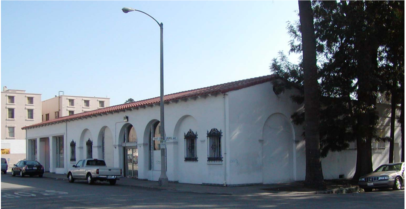
Photograph 2.2.1 The Exterior of the Paul R. Williams Building Facing East on Transit Street
