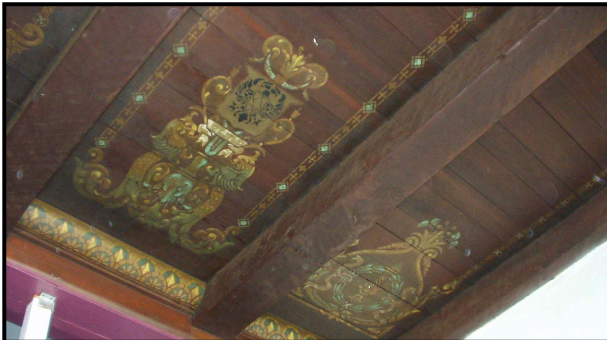
Interior Detail in the Paul. R Williams Building Showing Heavy Timber Elements and Gold-Leaf Coats of Arms
