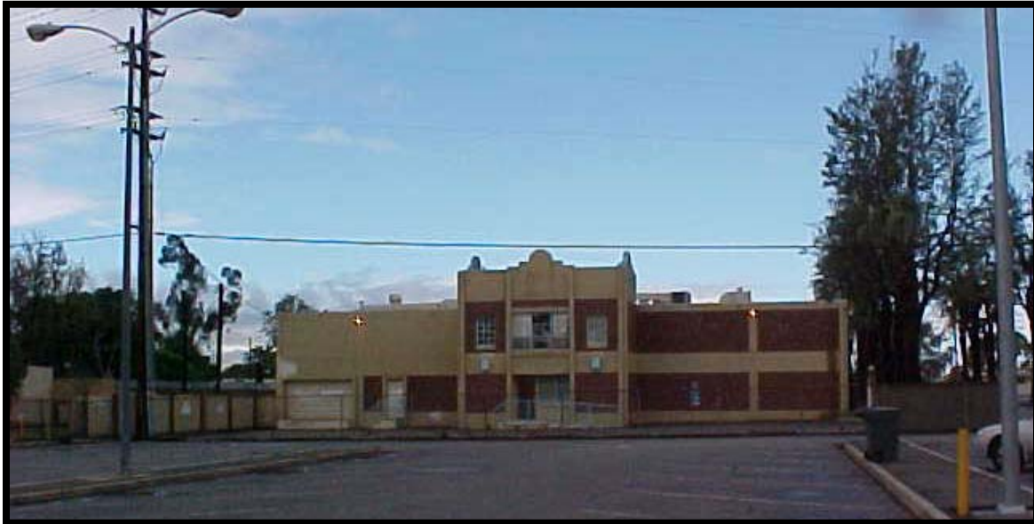
Photograph 3.2.21 Exterior View of the Tobias Building
