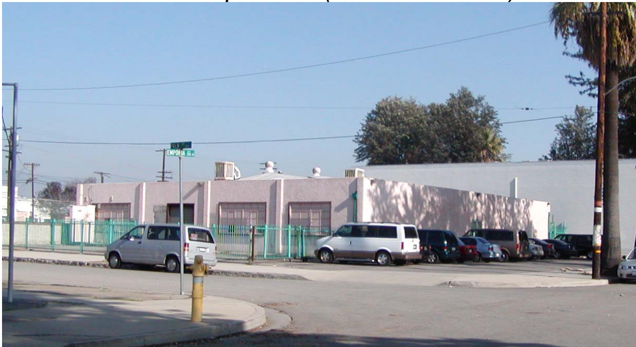
Photograph 3.4.2 Exterior of the Montalvan Building 228 West Emporia Street (APN: 1049-056-06-0000)
