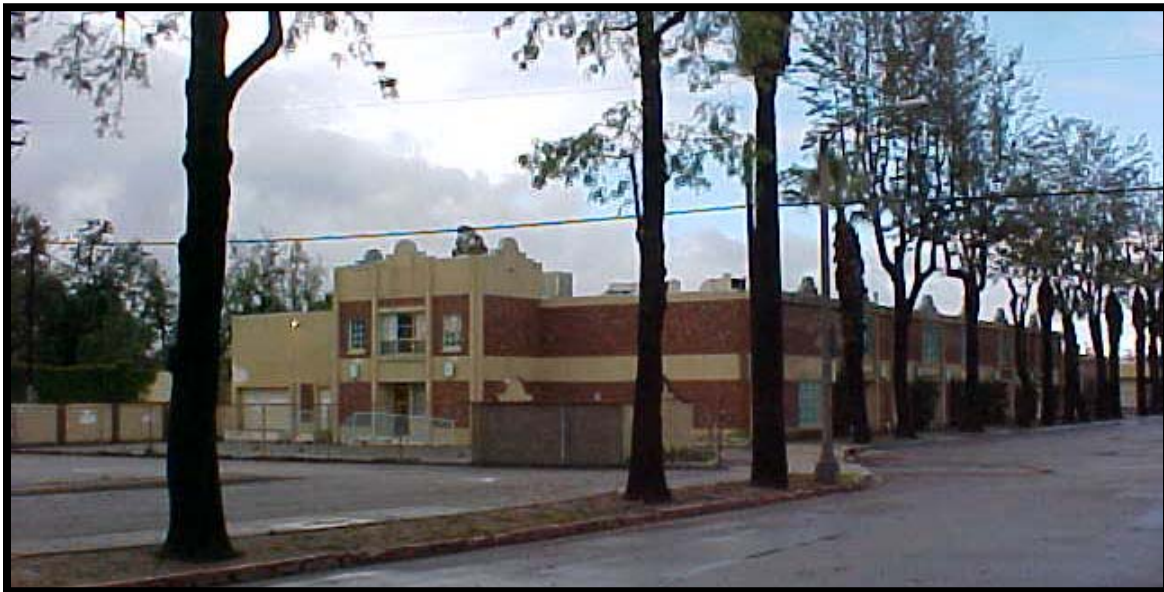
Photograph 3.2.22 Exterior View of the Tobias Building
