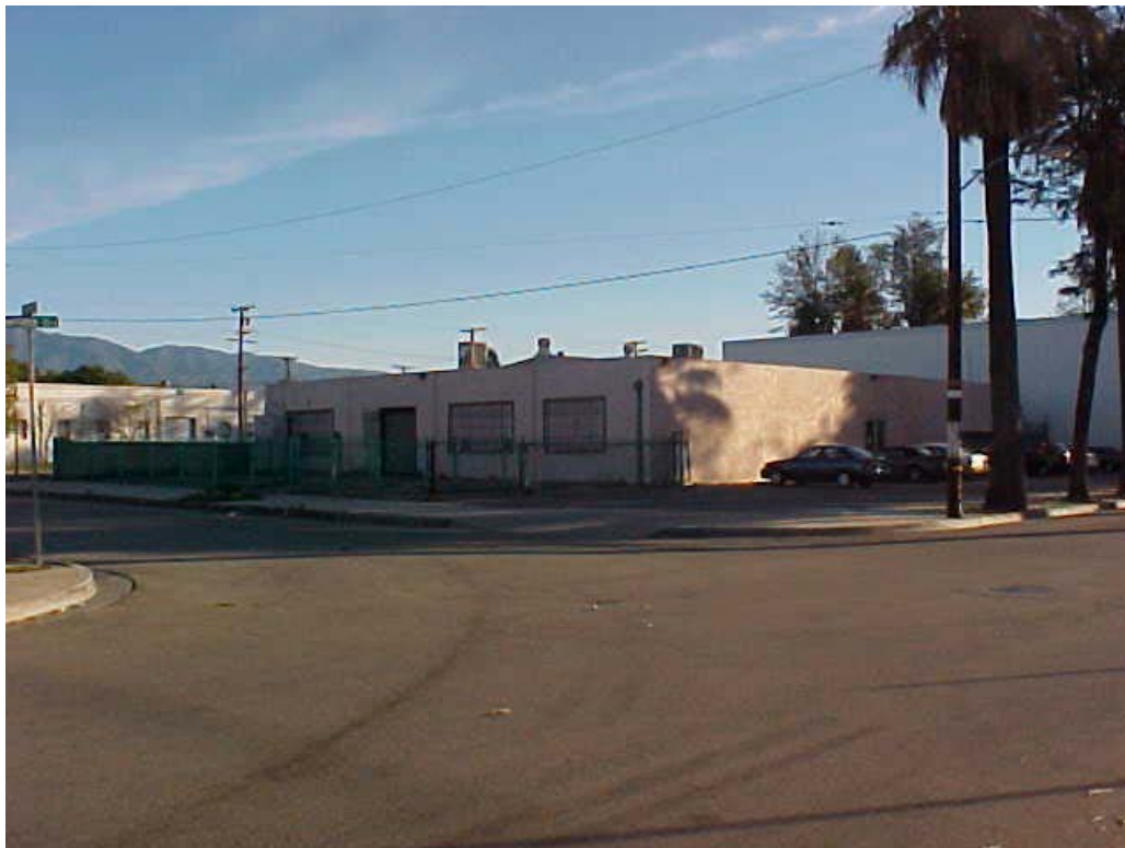
Photograph 3.1.1 A View of the Montalvan Building Looking Northeast from Emporia Street
