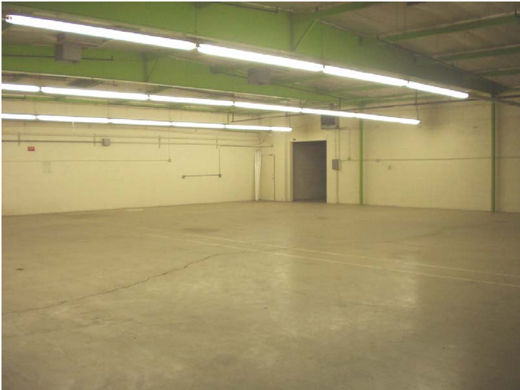
Photograph 2.2.9 The Interior of the Tobias Building – Warehouse
