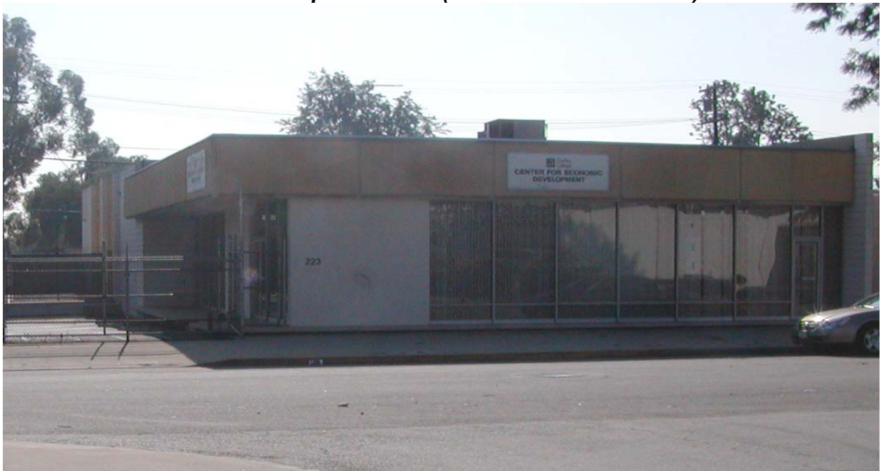
Photograph 3.4.4 Exterior of the Tobias Annex Building 301 West Emporia Street (APN: 1049-059-08-0000)
