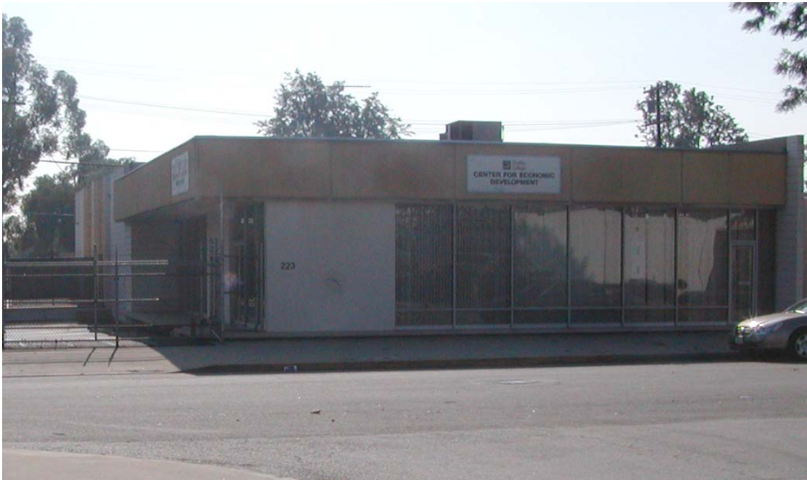
Photograph 2.2.10 The Exterior of the Tobias Annex Facing South on Palm Avenue
