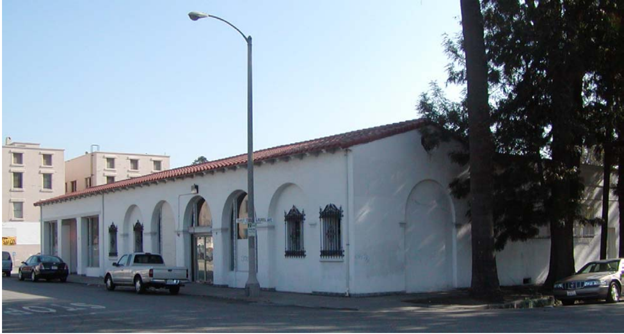
Photograph 3.4.1 Exterior of the Paul R. Williams Building 119 West Transit Street (APN: 1049-058-01-0000)
