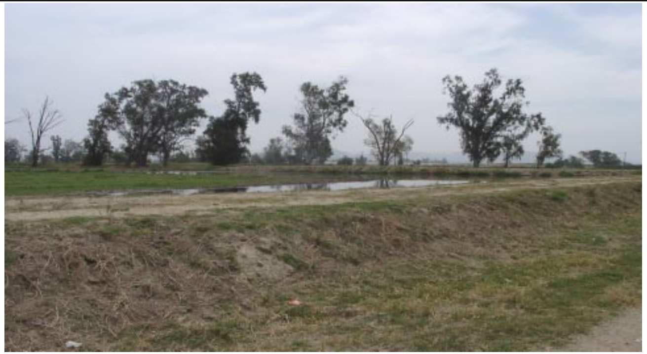
View to southeast of bermed detention area
