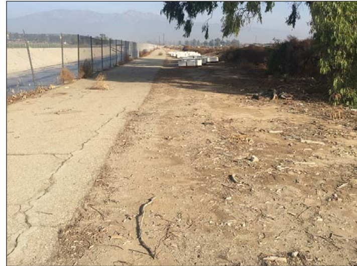
PHOTOGRAPH 8: View of the developed road that runs adjacent to the western study area boundary, facing north.
