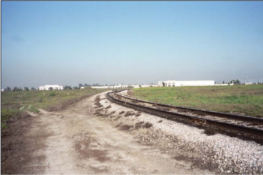
LOOKING WEST AT RAILROAD SPUR CROSSING THE WESTERN PORTION OF THE SITE.
