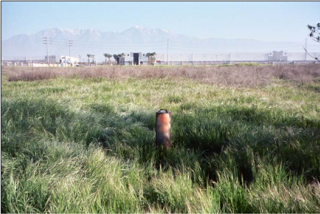
LOOKING NORTHWEST AT ON-SITE APPARENT LANDFILL GAS MONITORING WELL.
