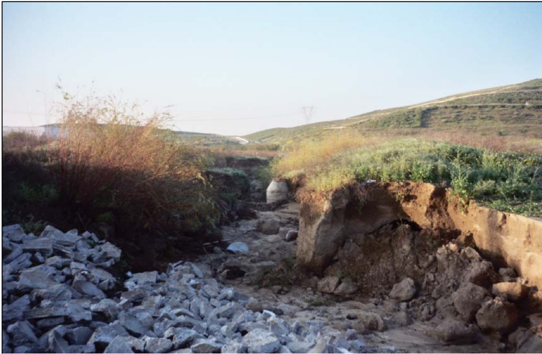
LOOKING SOUTH AT GULLY CROSSING THE SITE SOUTH OF DUPONT STREET.
