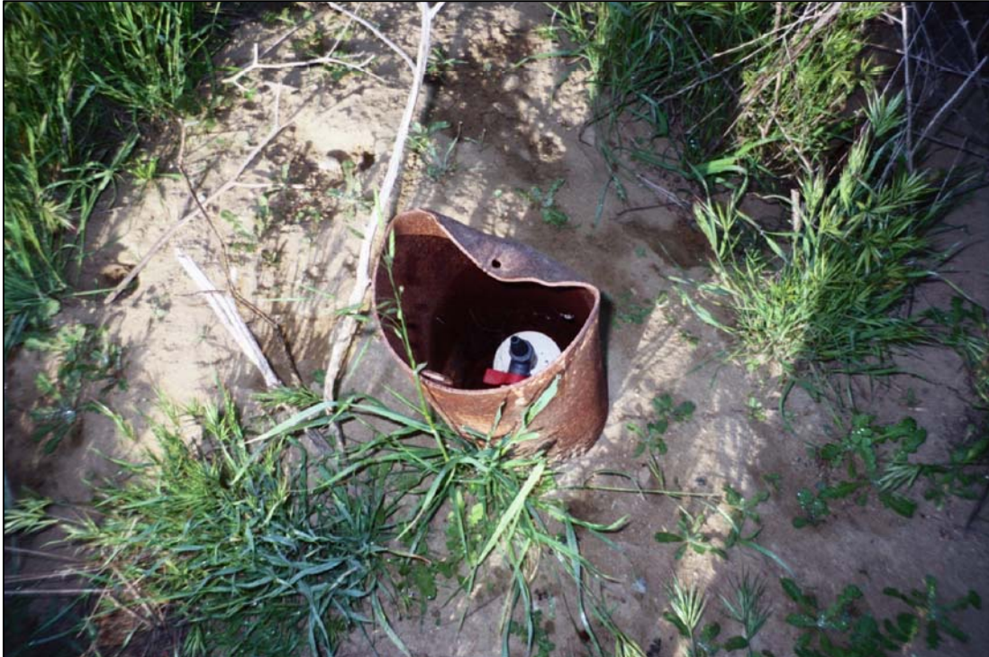
LOOKING SOUTHWEST AND DOWN AT ON-SITE APPARENT LANDFILL GAS MONITORING WELL.
