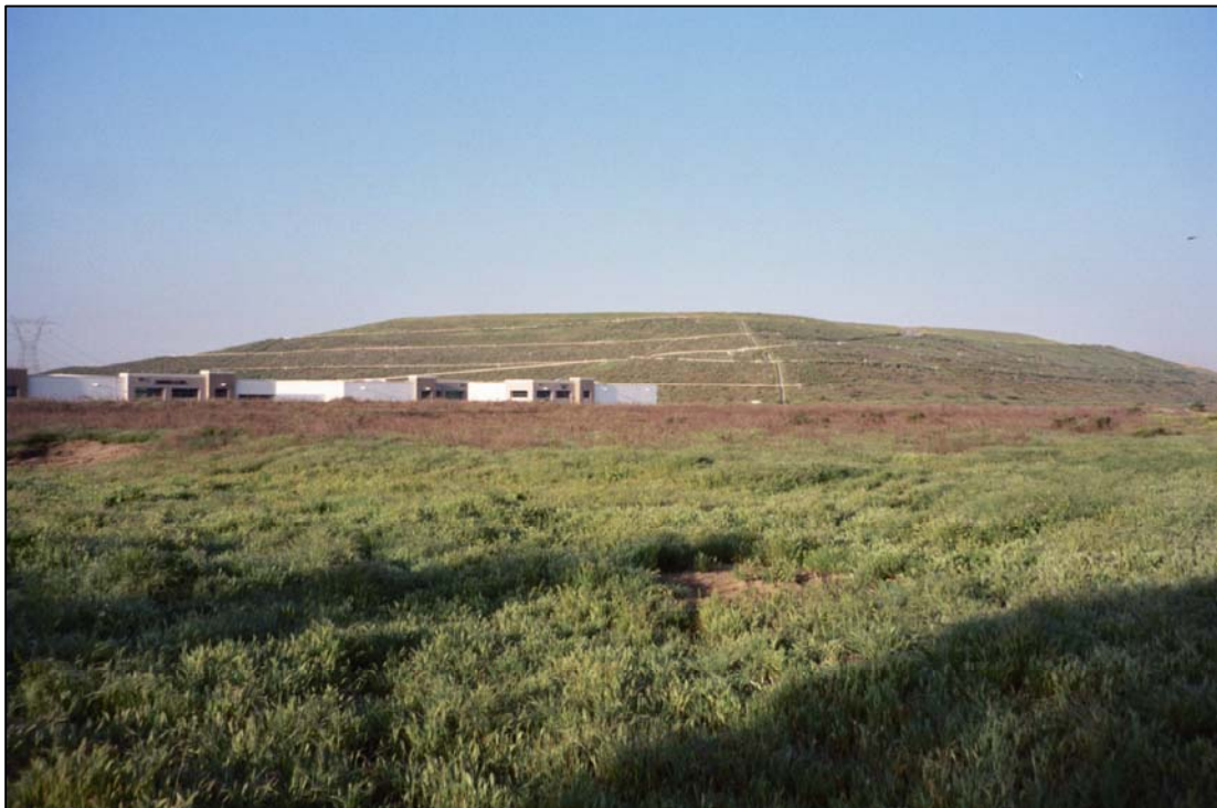
LOOKING SOUTHWEST ACROSS THE SITE FROM NEAR THE NORTHEAST CORNER.
