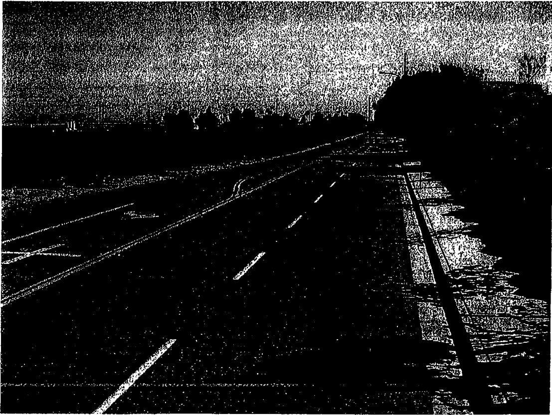
VIEW LOOKING SOUTH DOWN TURNER AVENUE FROM NORTHWEST CORNER OF THE SITE. SITE IS TO THE LEFT WITH SINGLE FAMILY RESIDENCES TO THE RIGHT.
