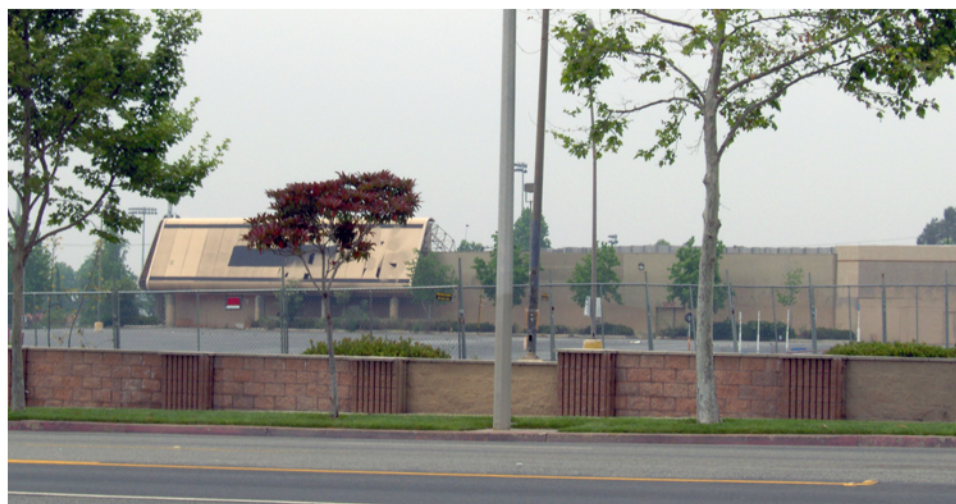
Village wall along Mountain Ave.
