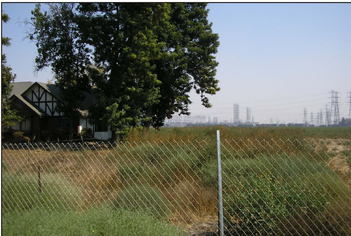
Photograph 8: Looking east toward abandoned home and electrical substation in the background.
