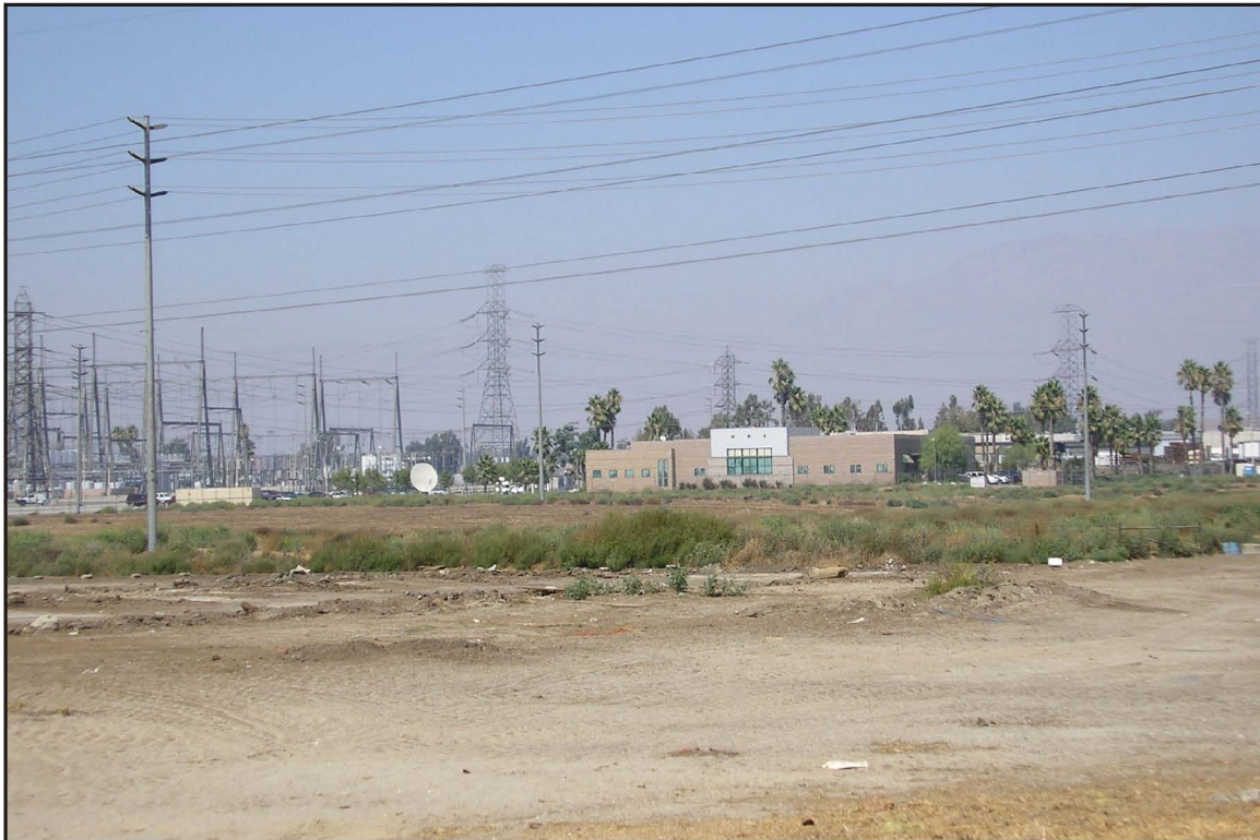
Photograph 16: Looking northwest toward Edison electricity building and electrical substation.
