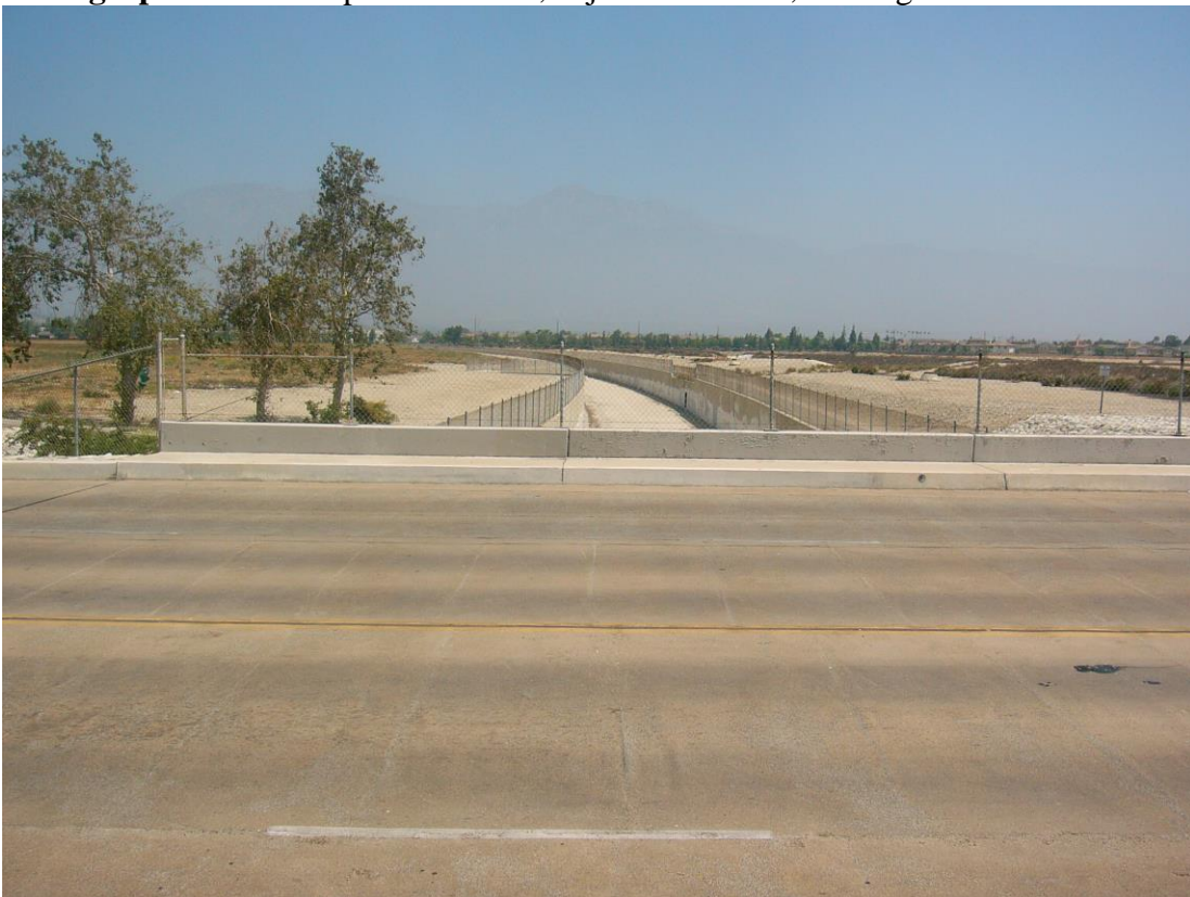
Photograph 6: Central portion of site, looking south along culverts.
