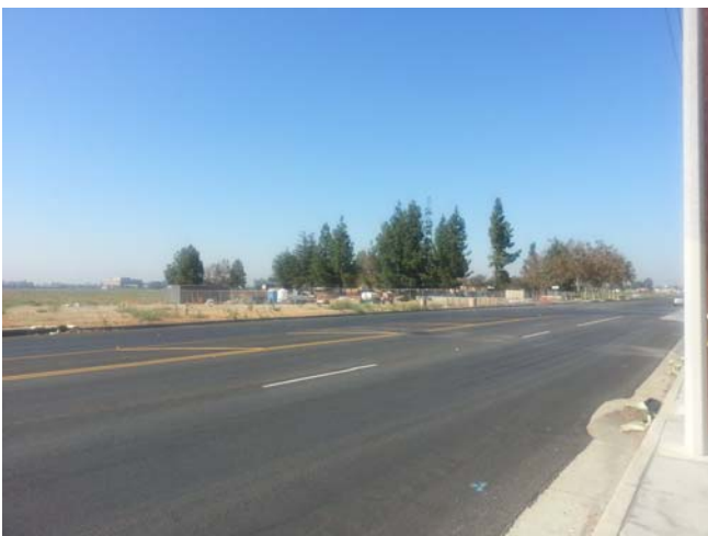
L11_Construction East of School 34, 4' 38.933000", 117, 36' 4.039000"
