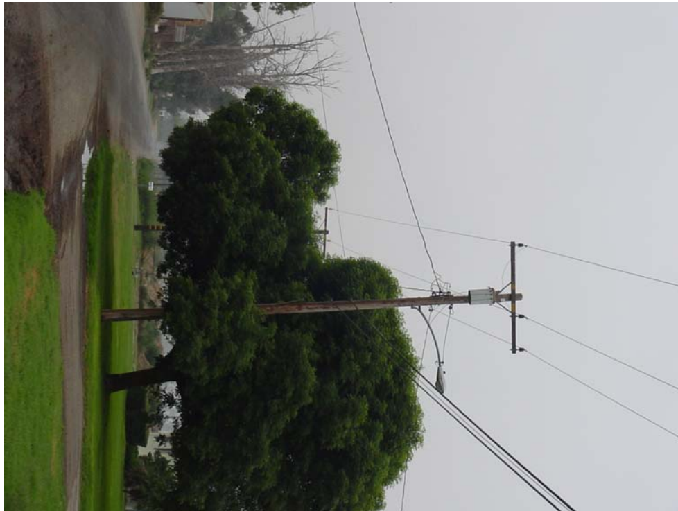
View of a single pole mounted transformer located along the south property boundary.
