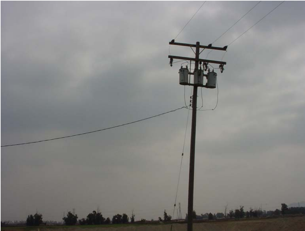
Pole-mounted transformer located next to irrigation well #3
