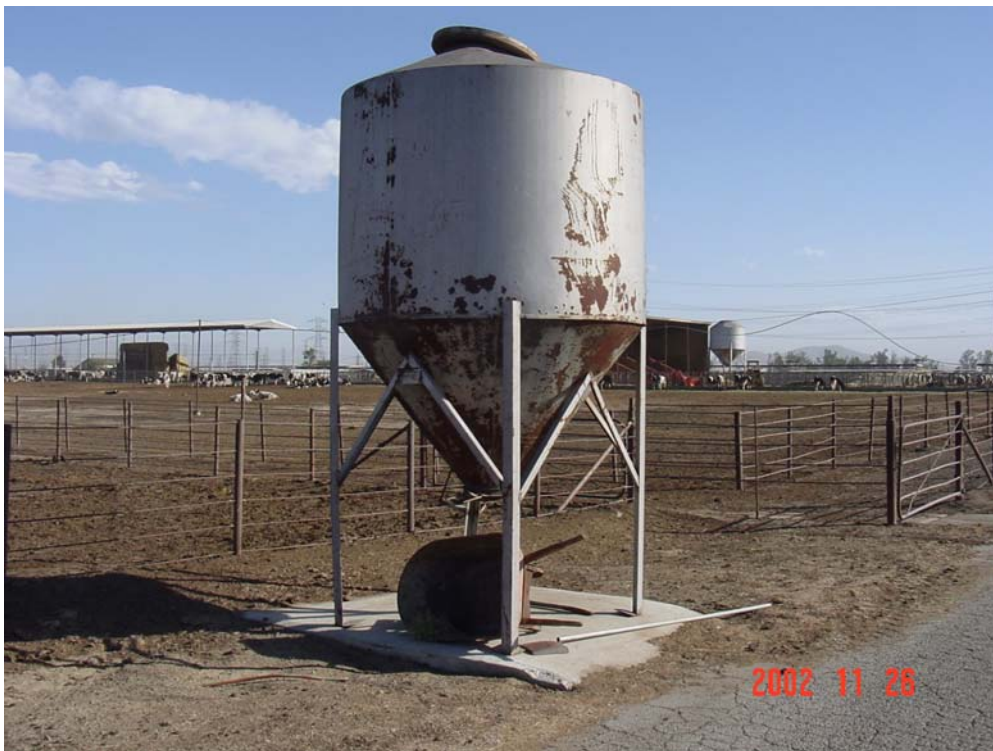
Overview Of Grain Silo 3.
