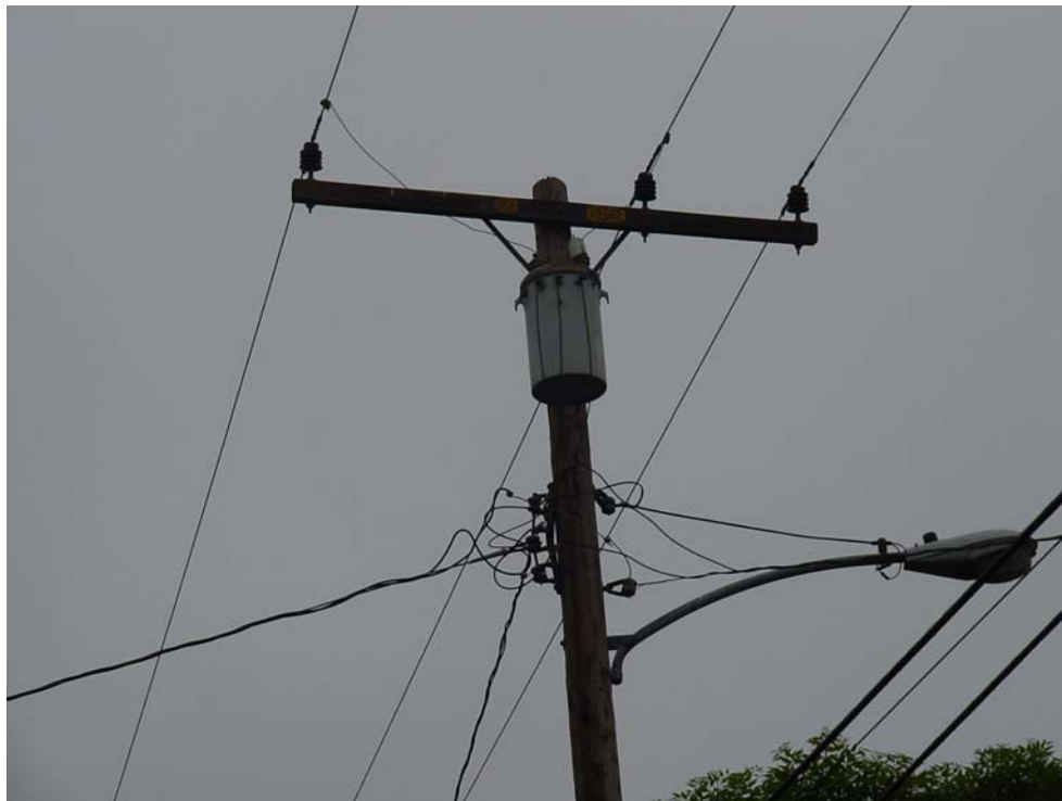
Close up view of a single pole mounted transformer located along the south property boundary.
