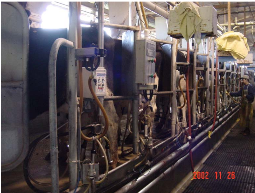
Overview Of Inside Of Milking Barn.
