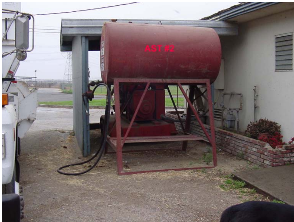
View of AST No. 2 adjacent to the southeast corner of the milking barn.
