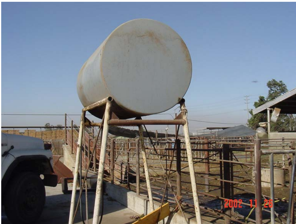
Overview Of AST 3, 500 Gallon Diesel Fuel.
