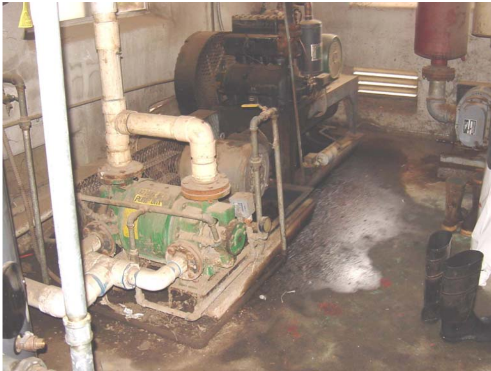
View of vacuum pump and compressor in the equipment room.
