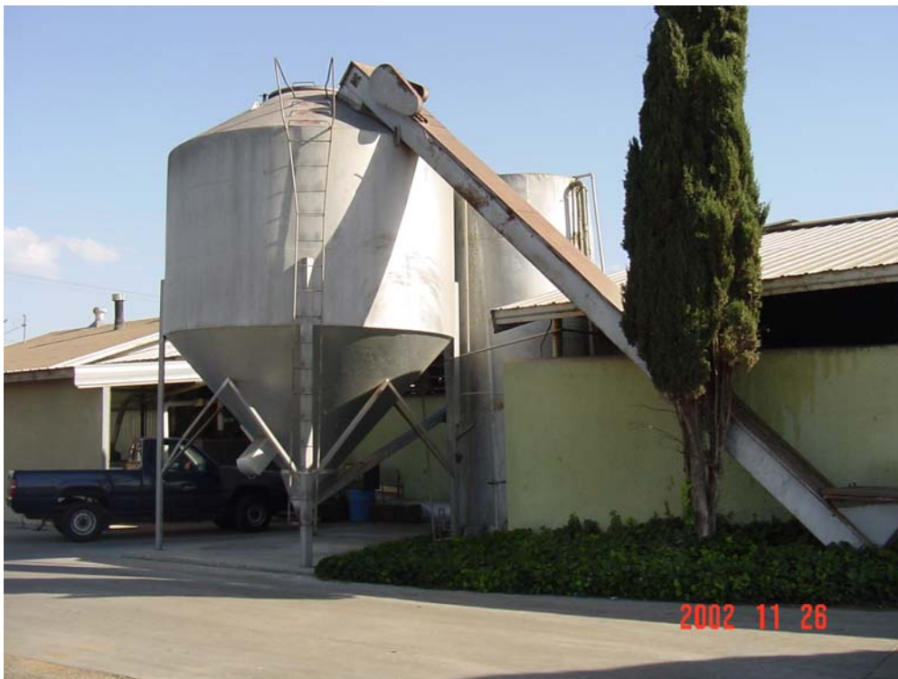
Overview Of Grain Silo 1 And Water Tank AST 2.
