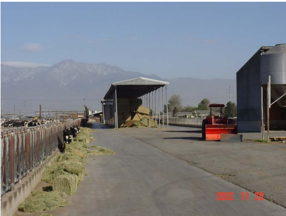
Overview Of Hay Barn 3 and 4 And Grain Silo 4.
