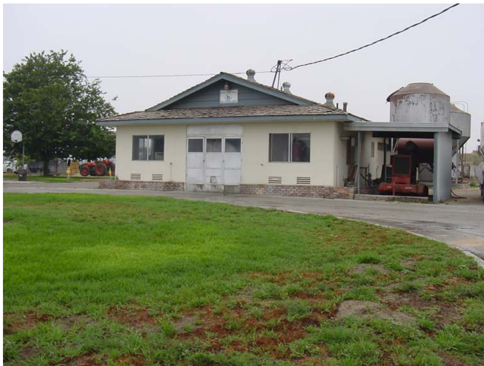
Overview of the milking barn looking north-northwest from Eucalyptus Avenue
