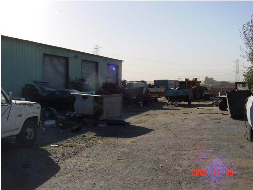
Overview Of Northeast Corner.
