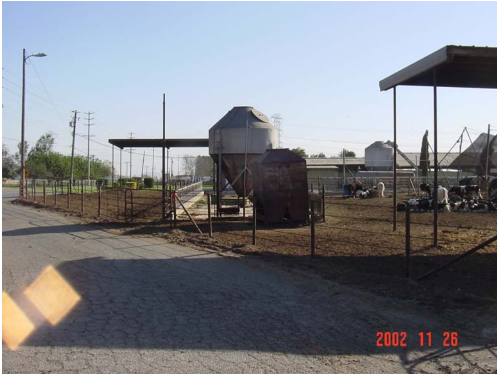
Overview Of Grain Silo 2.
