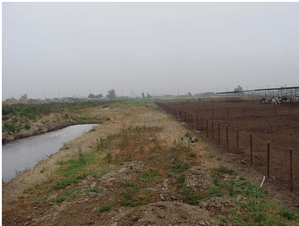
Overview of holding pond No. 3, looking north.
