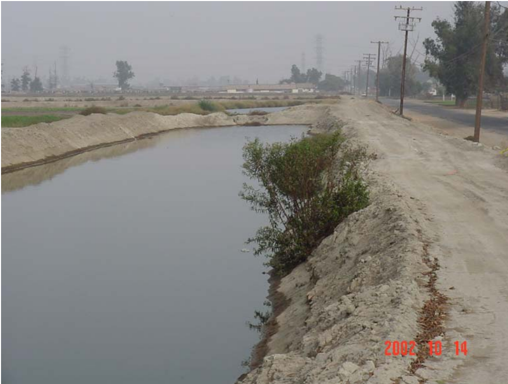
Percolation pit and utility poles on southern border of property
