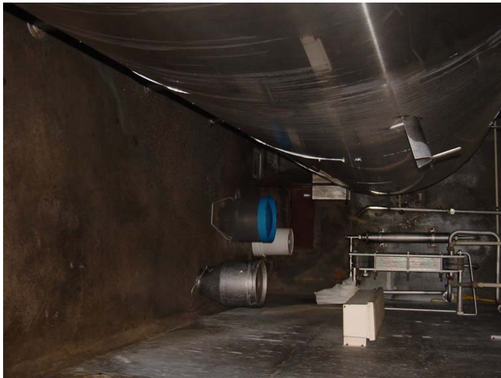
View looking north along the east side of AST No. 1.
