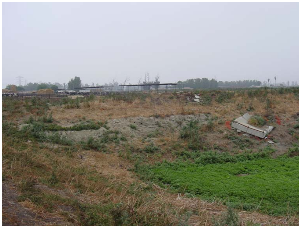
View of Holding Pond No. 1 looking south-southwest.
