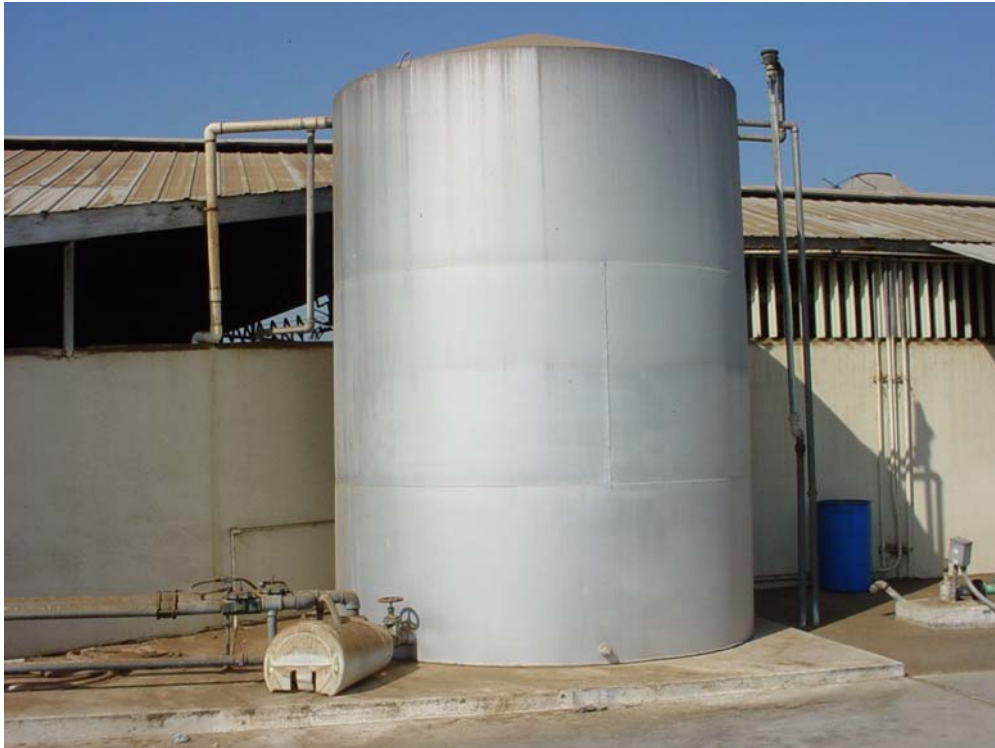
Approximately 10,000 gallon capacity water well AST on east side of milking barn
