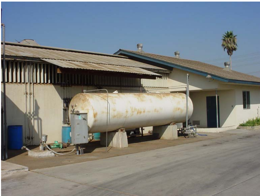
7,000 gallon capacity water AST on east side of milking barn
