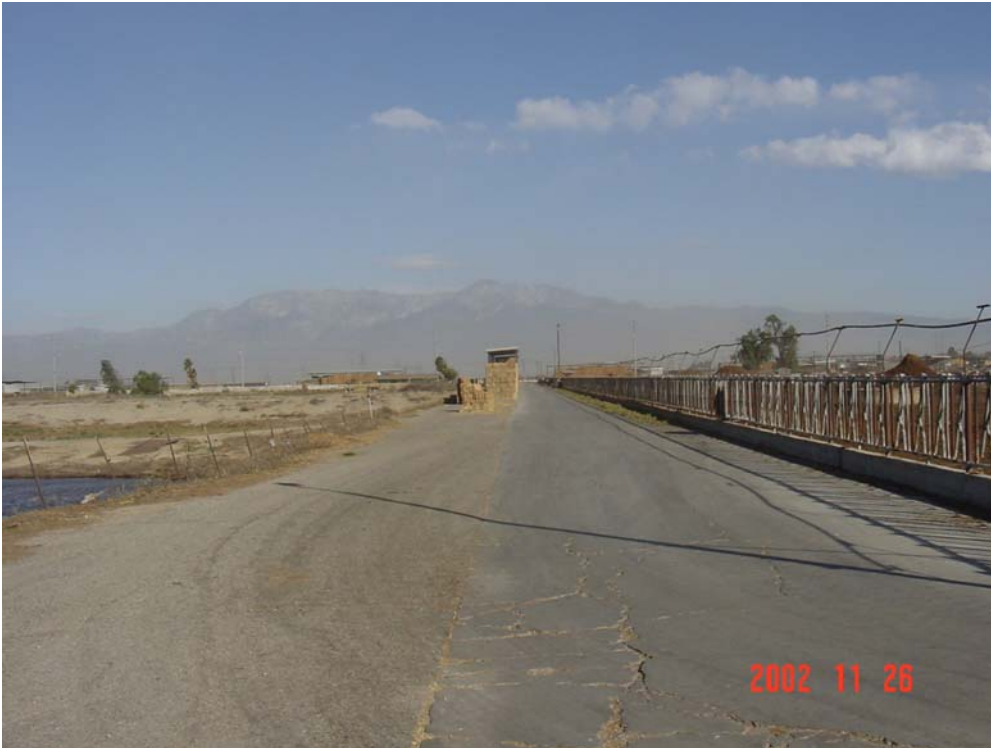
Overview, Looking North From Pond 6.
