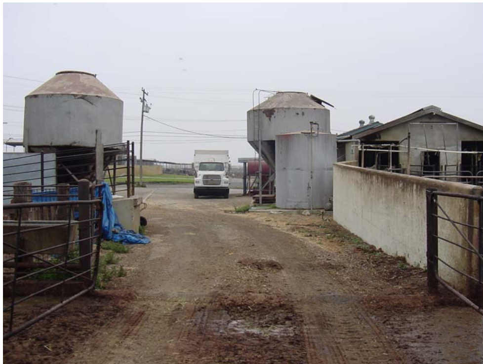
Overview looking south along the east side of the commodity bin.
