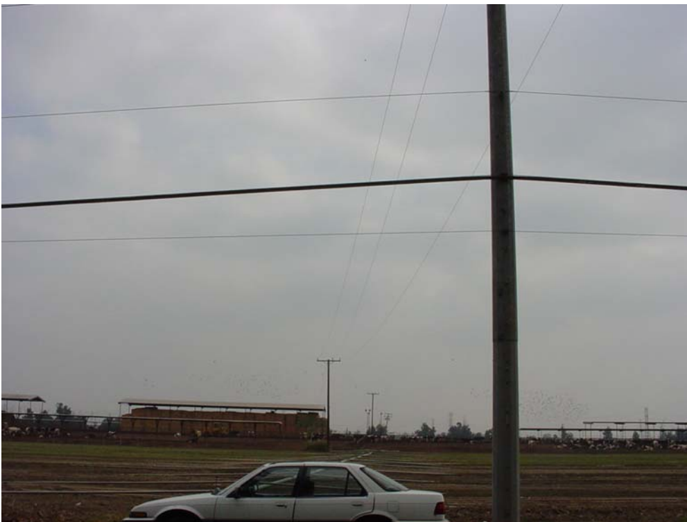
Utility lines running from Archibald to irrigation well #3
