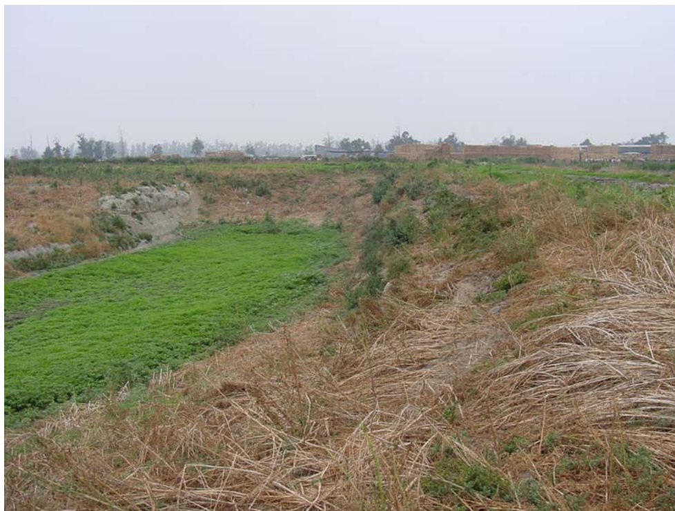
View of Holding Pond No. 1 looking west.
