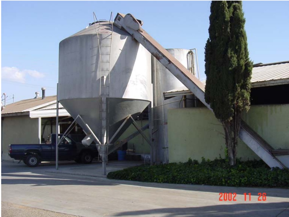
Overview Of Grain Silo 1.
