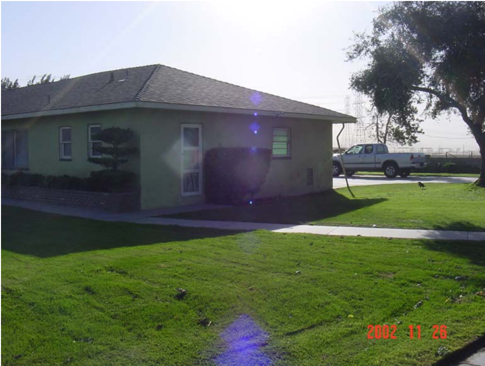
Overview Of Detached Garage At 10469 Edison Avenue.
