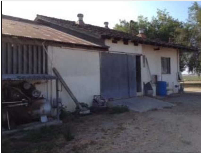
This photo is taken of the west facing section of Building B. The picture displays how the shed attaches to the tank section.
