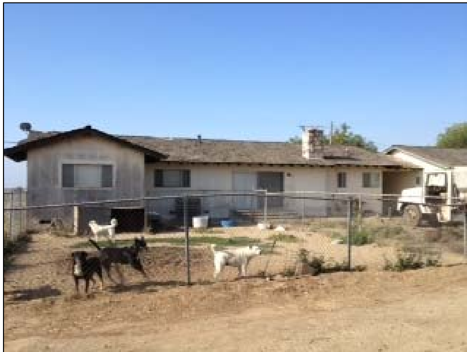
This photo includes the view of the northern façade, or back, of Building A. Photo was taken from just northeast of the home.
