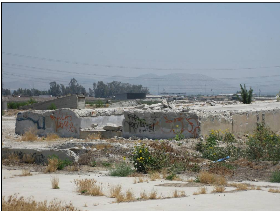
View of a demolished dairy located along Edison Avenue in the northern half of the project area. Most of the dairies and dairy remnants off Edison were built in the 1968-1969 period.
