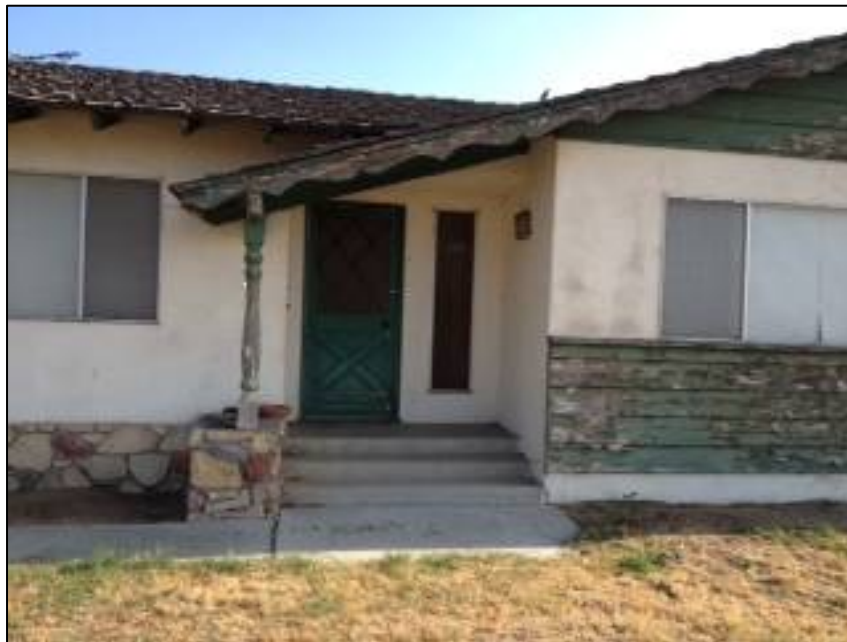
Front entry way on the south side of the Building A residence taken from within the front yard. Note scrolling of fascia and other Ranch style details. Aluminum slider windows and doors appear original.
