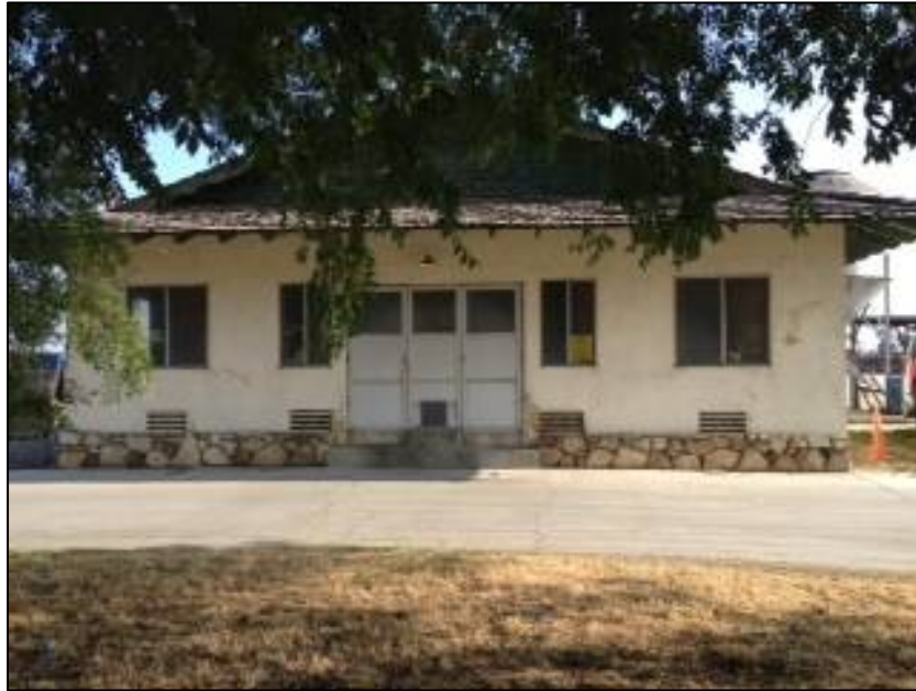
Front (south) façade of Building B which faces south toward Eucalyptus Avenue. The driveway arcs so the milk tanker can park then access the small opening in the front door for pumping.
