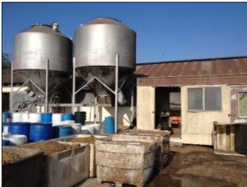
The photo is a view of the eastern facing portion of Building B and the grain silos.
