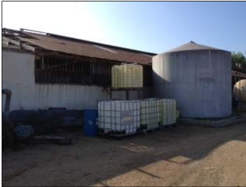
The photo depicts the northwest corner of Building B.
