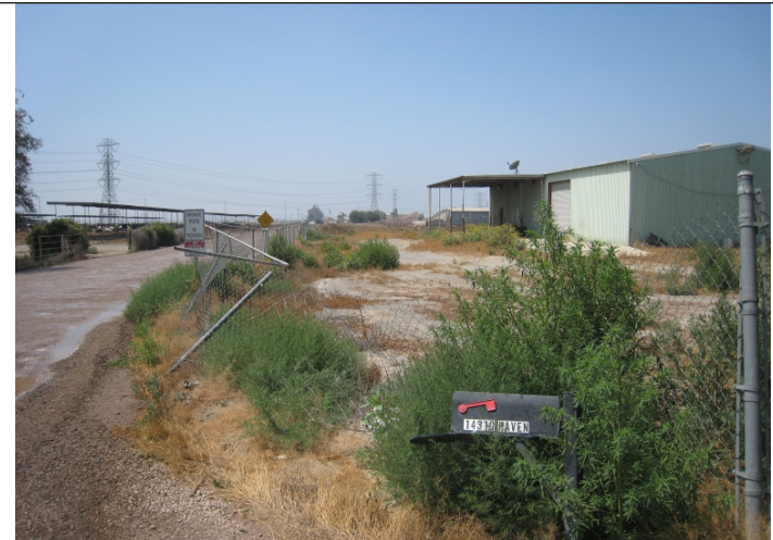
Photograph 16: South facing view of abandoned development at corner of Edison Avenue and Haven - Summer Avenue. June 19, 2012.
