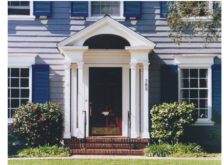
Articulated Portico Entry
