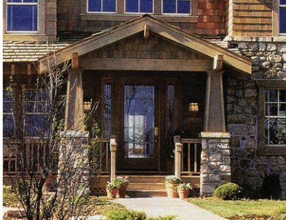
Front Porch with Battered Columns
