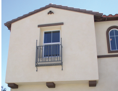
Tile Roof, Gable Vent and Wrought Iron Accents
