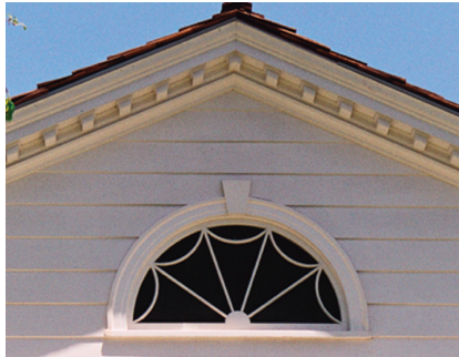
Accent Window and Enhanced Molding details
