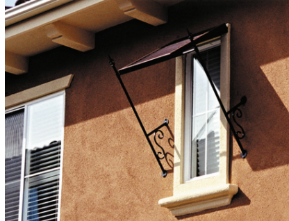
Vertical Windows with Wrought Iron Detail
