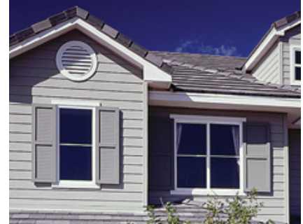
Vented Gable and Horizontal Siding
