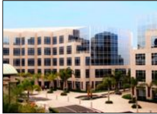
Extended window panels create interest and provide shade, which helps to conserve energy.
