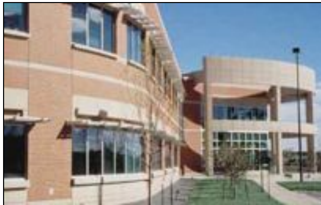
The radius in the building corner is repeated in the curved open pergola at the entry. The pergola simultaneously creates shadows.
