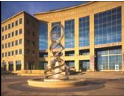
Concave buildings help create shade and cast shadows. They can also help extend the plaza area and create protection from the wind.
