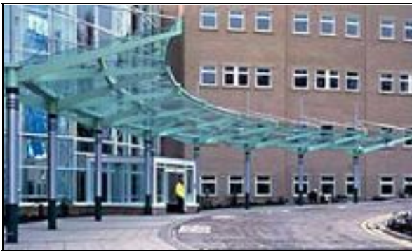
The glass pergola adds interest while highlighting the entrance area of this hospital and also provides shelter.
