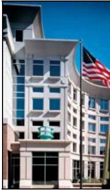
Overhangs provide interesting depth and shadows while also providing sun protection.
