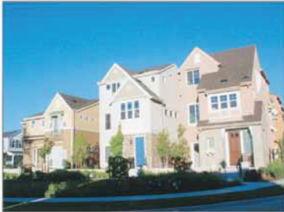
Varied building massing
