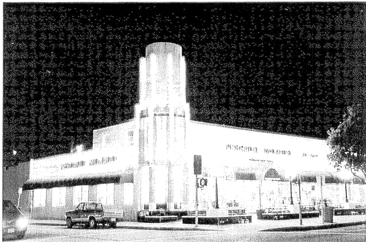
Figure 68, Art Deco Style. Pescado Mojado, formerly the Blue Seal Laundry, is a good example of Art Deco form and ornamentation, with its streamlined elements, stepping tower, and tile detailing.
