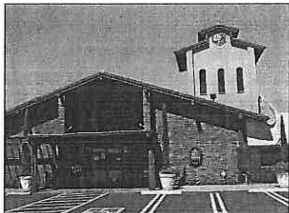
Modern materials and construction used in winery building. Note tower element, exposed rafter tails, and arbor over the entry.
