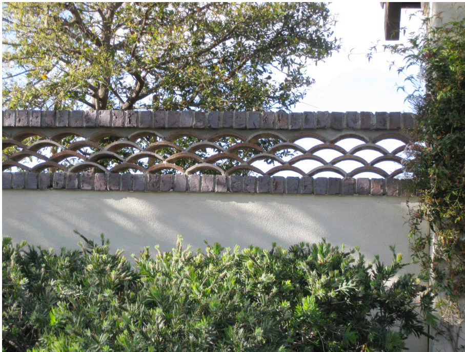
Brick, Tile, & Stucco Wall
