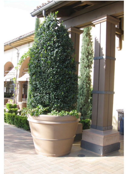
Lightweight Precast Container Pots Over Podium Parking
