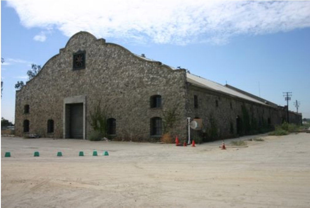
Building 54, north elevation, east end of building, view looking southwest, September 2008.
