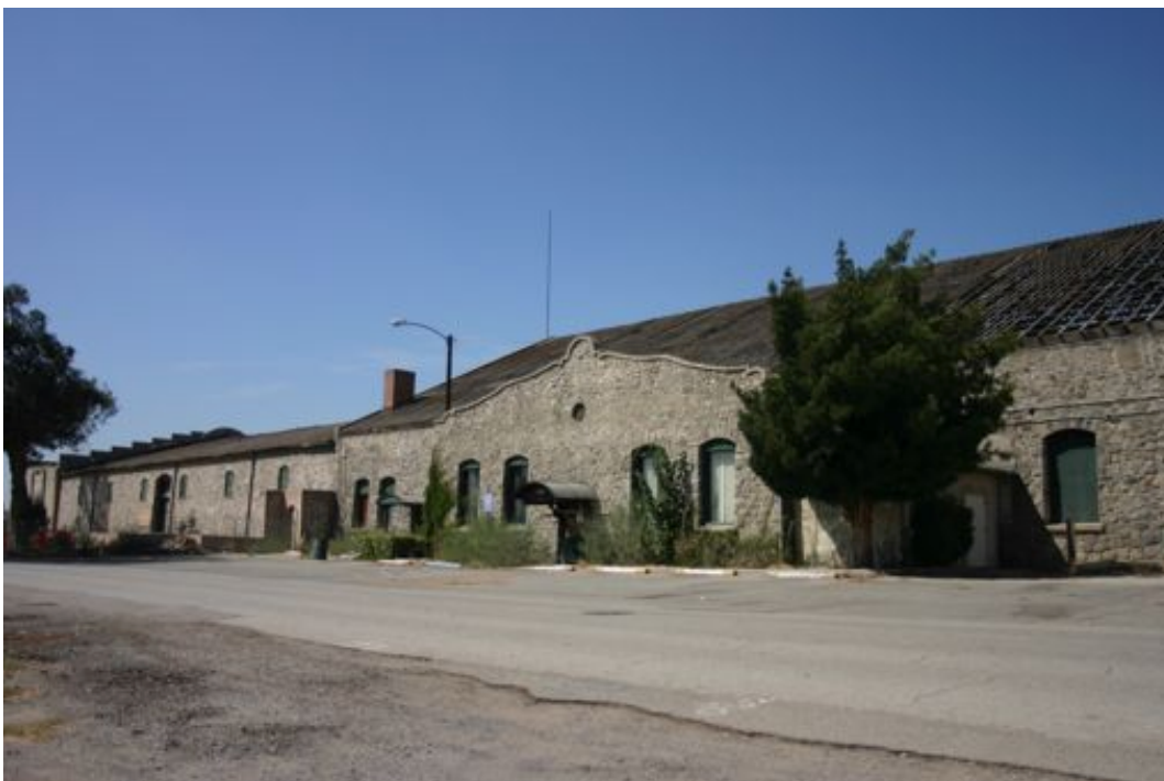
Building 54, south elevation, mid-section of the building, view looking northwest, September 2008
