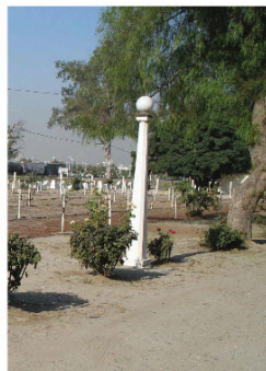
5. WHITE CONCRETE LIGHT POLES W/ ROUND GLOBES
