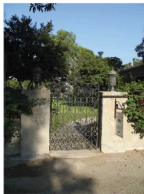
16. MASONRY PERIMETER WALLS
