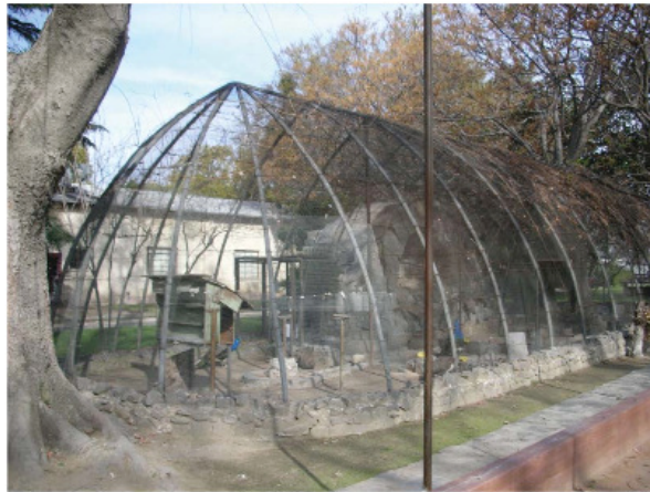
23. METAL AVIARY STRUCTURE
