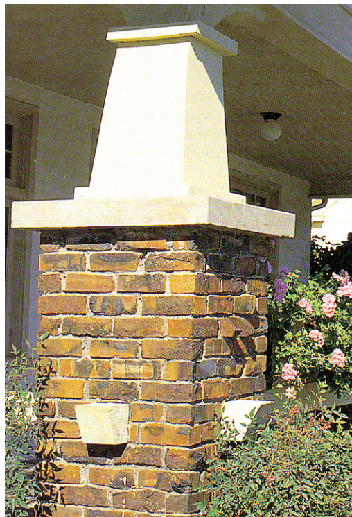
Typical Column Detailing appropriate to Style
