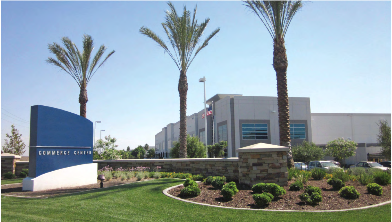
Photo 7.3 - Example of Industrial building
