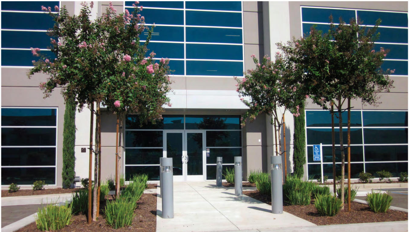
Photo 7.5 - Example of Industrial lighting at office entry
