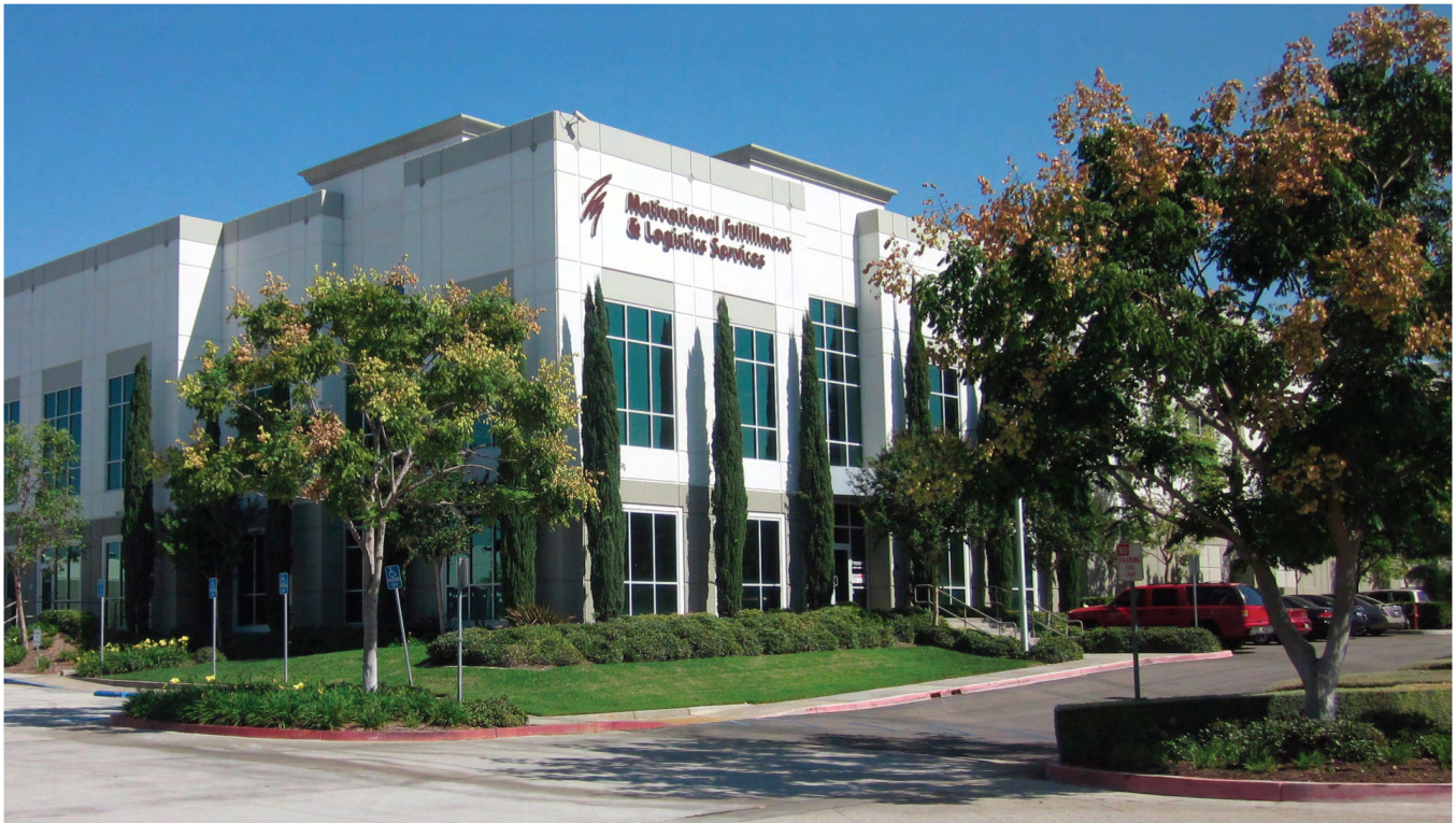
Photo 7.2 - Example of Industrial building
