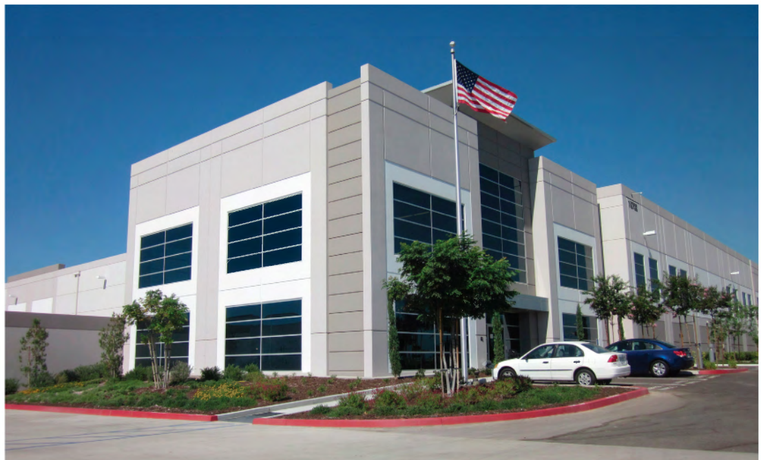
Photo 7.1 - Example of Industrial building with corner office area
