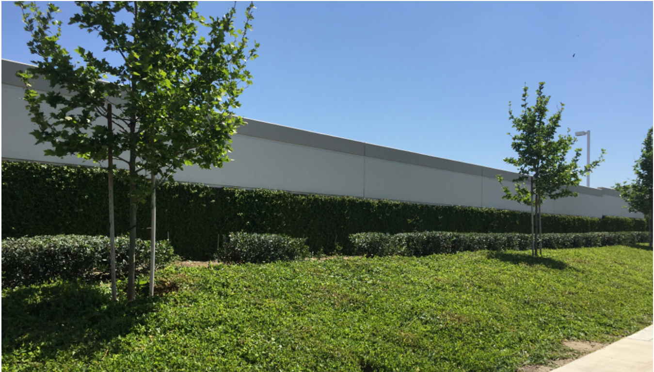
Photo 7.4 - Example of typical screen wall with landscaping
