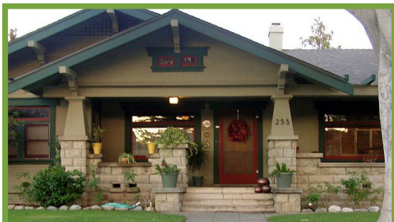
Gable end roofs with extended rake end. Large proportioned columns with heavy base and tapered column form.
