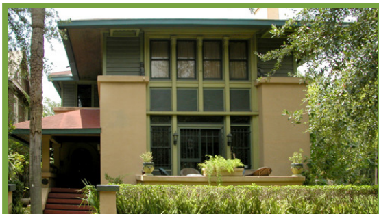
Horizontal massing reinforced by low pitched hip roof, wainscot banding and window pattern.
