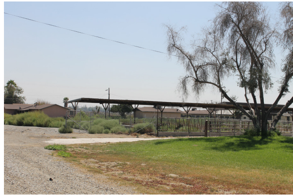
2. Existing dairy farm looking southeast.
