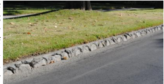
ROCK CURB ON EUCLID AVENUE
