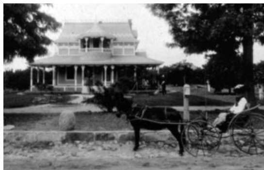
ORIGINAL ROCK CURB ON EUCLID AVENUE
