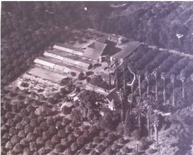
Photo: Large citrus property in the Ontario or North Ontario area – no name or date. Photo shows a large scale Victorian-era home (of the Queen Anne style) surrounded by groves with only the building's façade visible from the driveway. A number of grove associated buildings can be seen to the rear of the residence. (courtesy of the Ontario Public Library, Model Colony Room, Ontario, CA)
