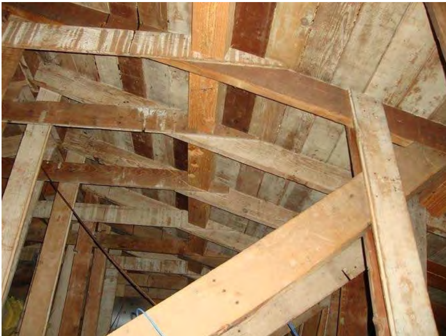
Image 4. Roof framing above second floor.
