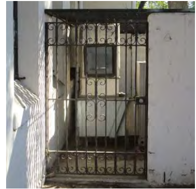
Gate (1 of 2) at south elevation mechanical enclosure.
