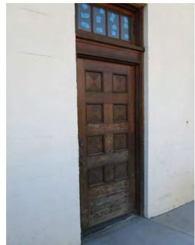
Door and transom at north elevation.
