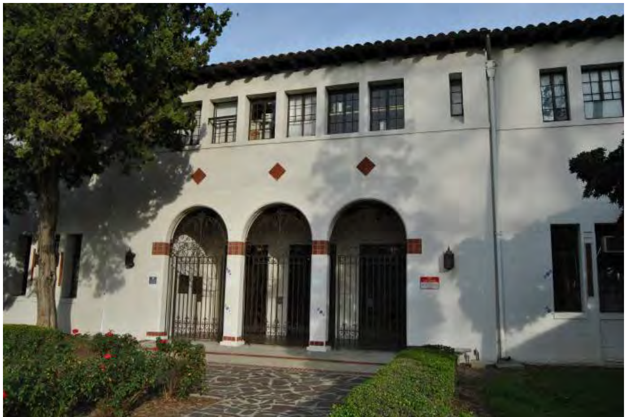
Three gates at west courtyard elevation.
