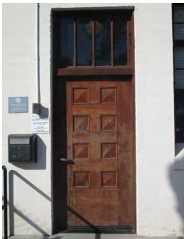
Door and transom at east elevation.
