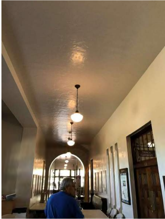
Figure 1 - 1st Floor Corridor Lighting
