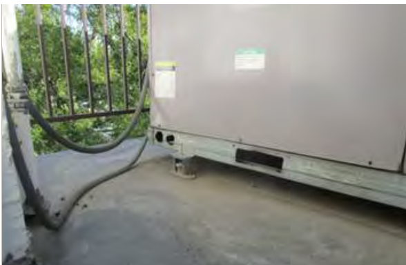
Roof mechanical pad seen from second floor window.
