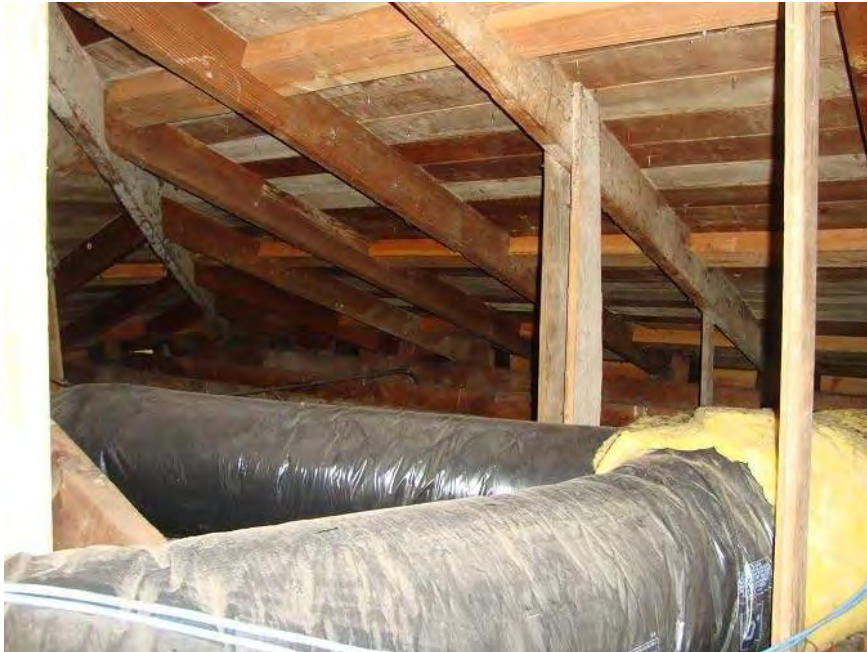
Image 3. Roof framing above second floor. Note straight sheathing.
