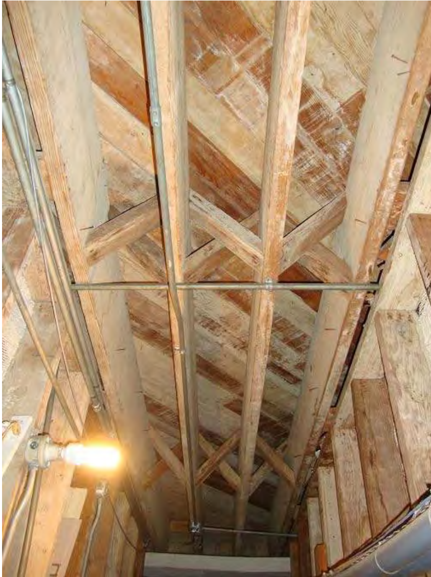
Image 5. Council chambers floor framing viewed from basement, note diagonal sheathing.
