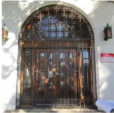
Door, sidelights and arched transom at south elevation.
