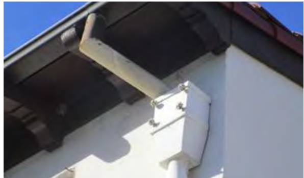
Typical painted downspout and conductor head.
