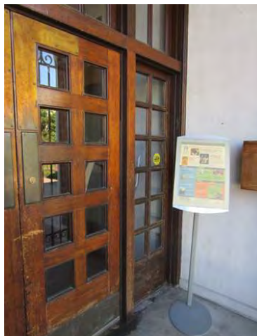
Door, sidelights, and transom at north elevation.
