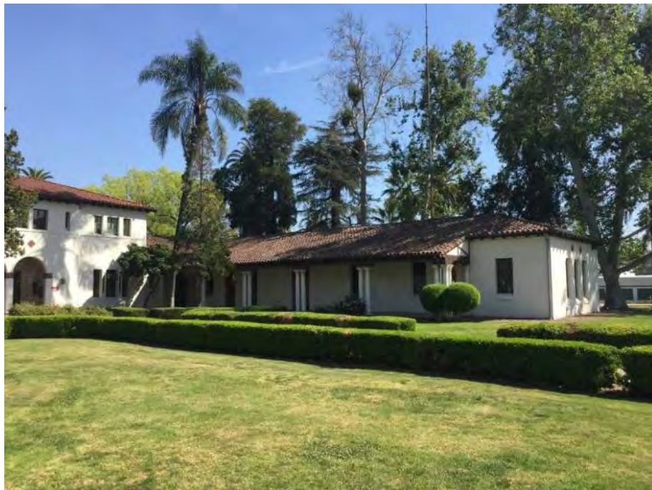
Image 2. North elevation of south wing.
