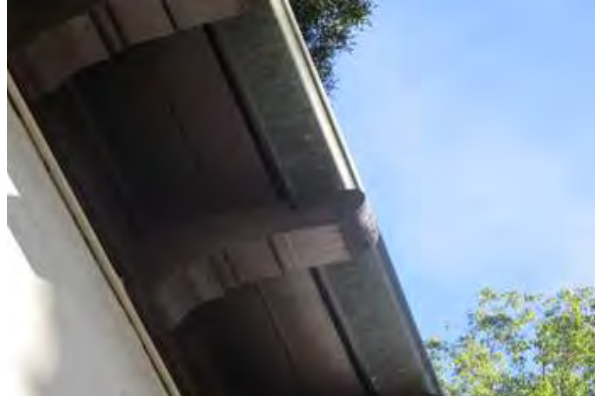
Typical eave condition showing overhang, decorative rafter tails, and copper gutter.
