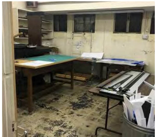
Basement workroom; note vinyl tile has been removed from concrete floor slab.
