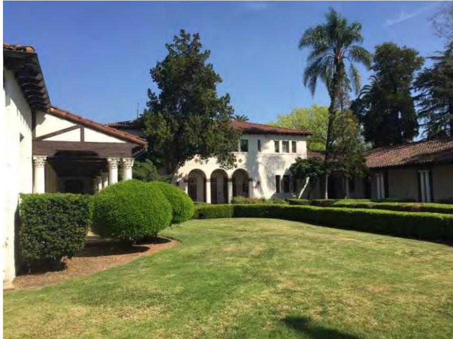
Image 1. West elevation, Museum entrance at center of photograph.
