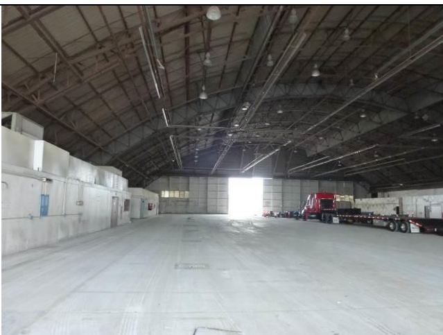
Image 5. View of the interior looking west.
