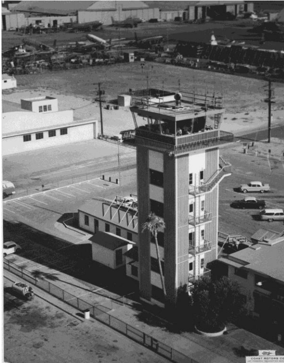
Image 13. View looking northwest at the south and east facades, ca. 1960. Source: Virgil R. Percy, photographer, July 18, 1969 [in Model Colony Room photo archives].
