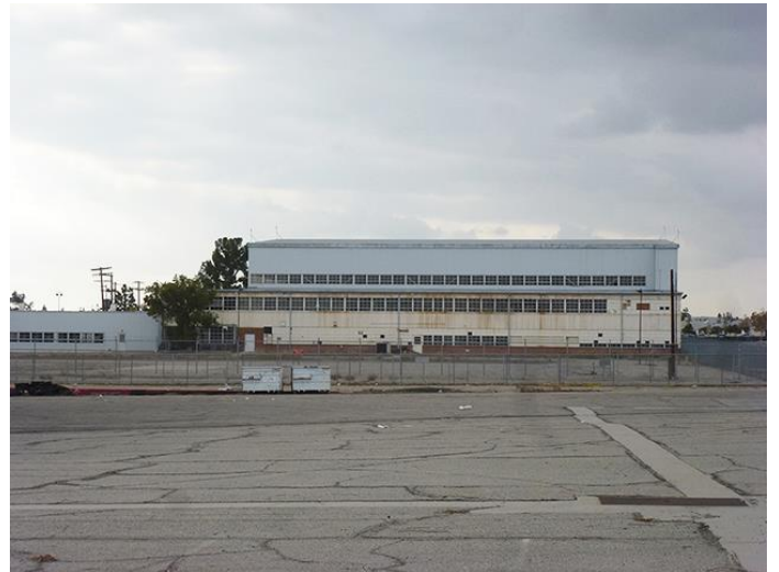
Image 8. View looking west at the east façade.
