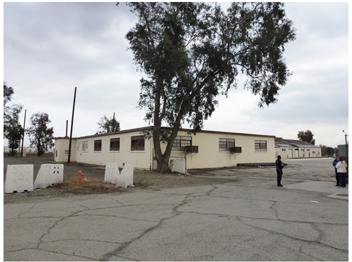
Image 4. View looking southeast at the north and west façades.
