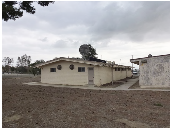
Image 3. View looking southeast at the north and west façades.
