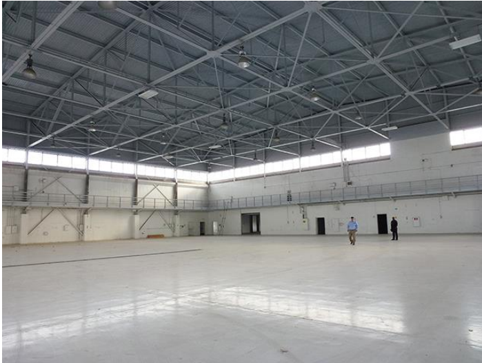
Image 13. Interior view of the hangar looking southeast.
