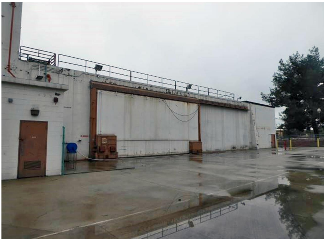
Figure 17. GE Jet Engine Test Cell 1, looking southwest. December 6, 2016. Source: ASM.
