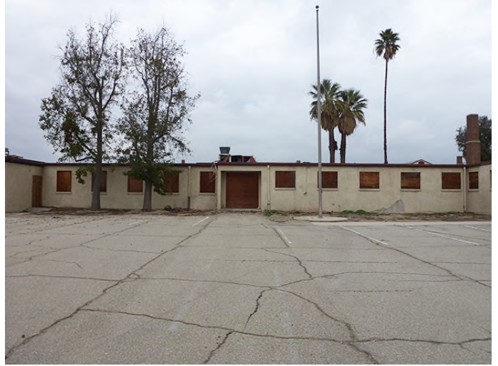
Image 6. Detail view of the south façade.
