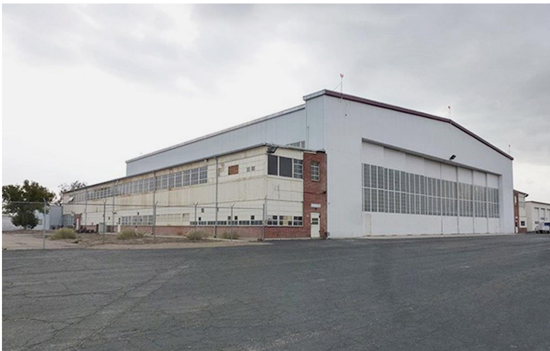
Figure 29. Air National Guard hangar, looking southwest at east and north facades. December 6, 2016. Source: ASM.
