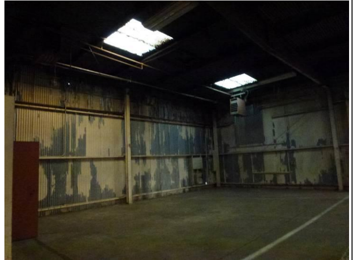
Image 6. Interior view of south wing.
