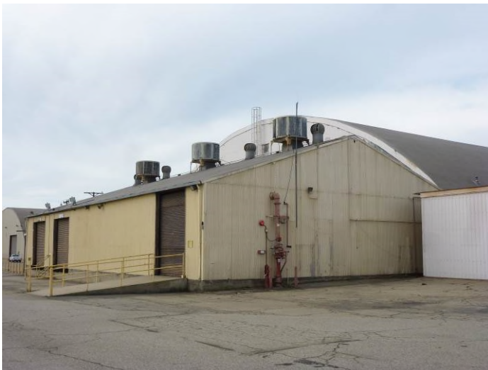
Image 7. View looking west at the southeast and northeast façades of Building 27.
