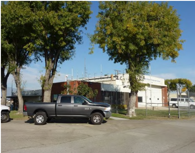
Image 11. View looking northeast at the west and south façades.
