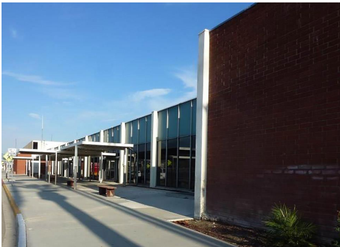
Figure 26. Primary façade of Terminal One, showing additions. December 6, 2016. Source: ASM.
