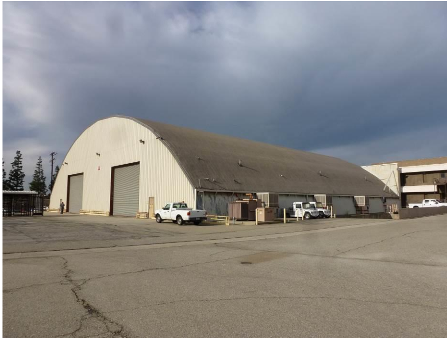
Image 1. View looking west at the southeast and northeast facades of Hangar 7 with the administration building to the right. ASM, December 1, 2016.
