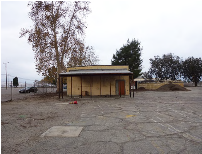
Image 1. View looking north at the south façade.
