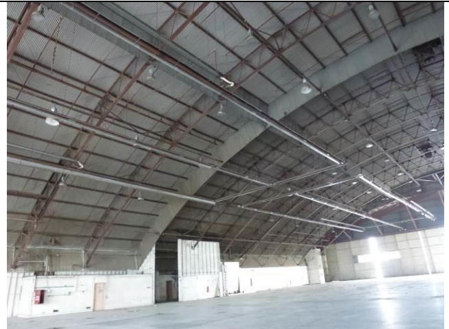
Image 4. Interior view looking northeast.
