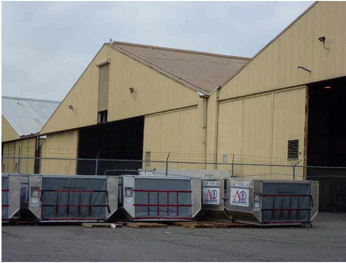
Image 1. View looking southwest at the north and east façades.
