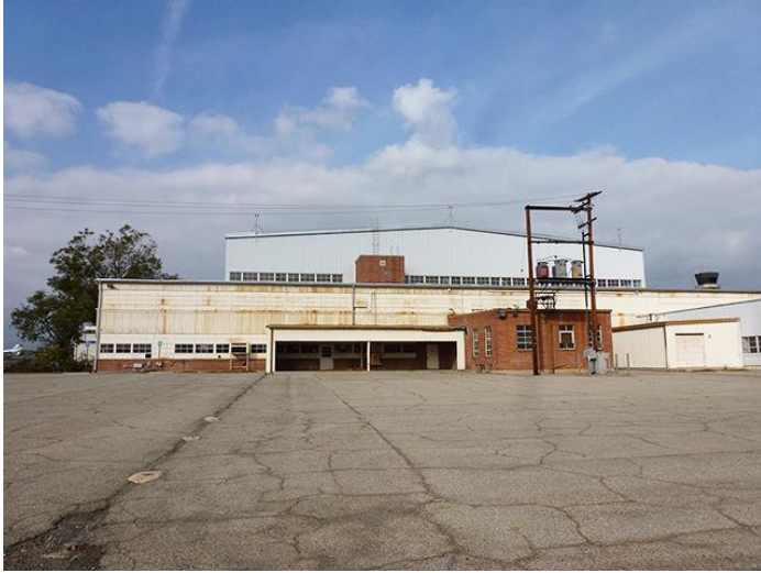
Image 5. View looking north at the south façade.
