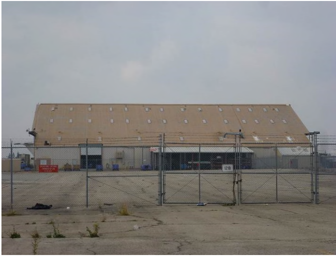
Image 1. View looking west at the east façade.
