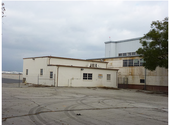
Image 4. View looking northeast at the west and south façades.
