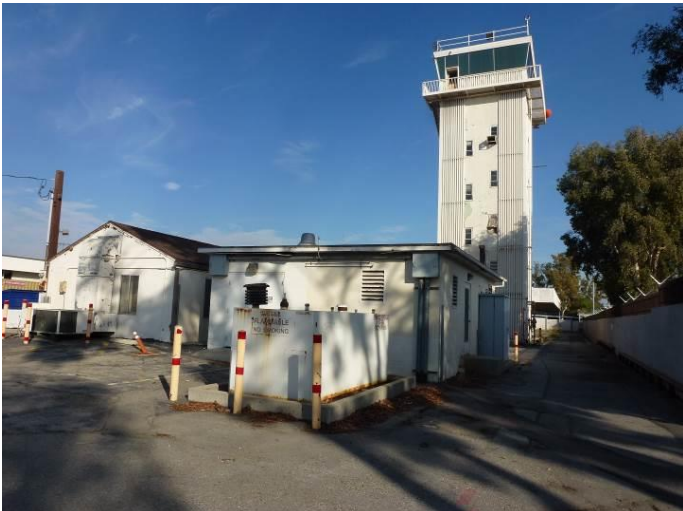
Image 3. View of Control Tower and ancillary buildings looking east. Only the Control Tower is recommended as a contributor to the historic district.
