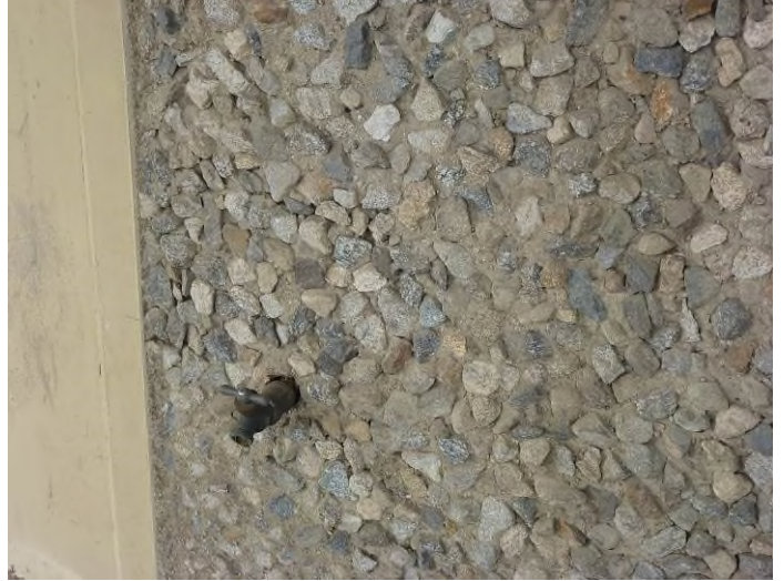
Image 2. Detail view of aggregate concrete panel.
