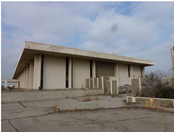
Image 3. Detail view looking northwest at the south and east façades.
