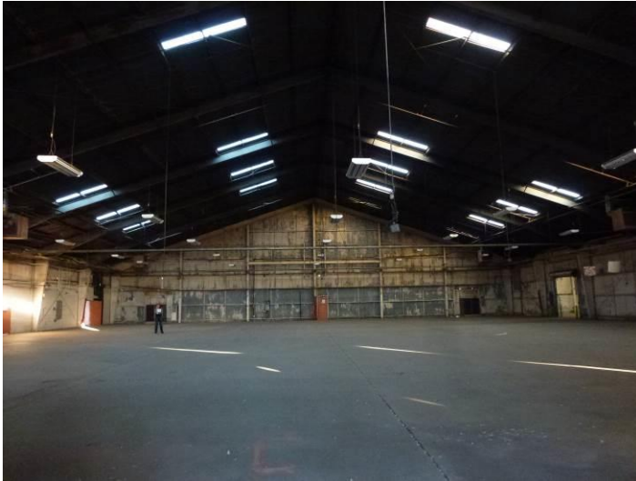
Image 5. Interior view looking southwest.
