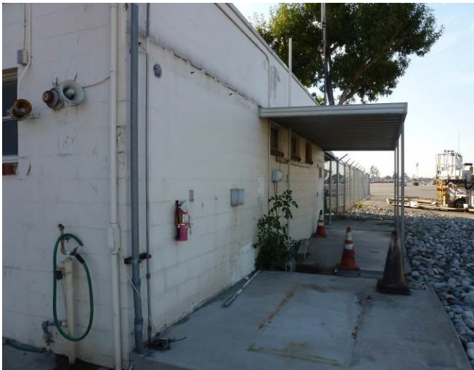
Image 7. Detail view looking west at the north façade of the personnel quarters.
