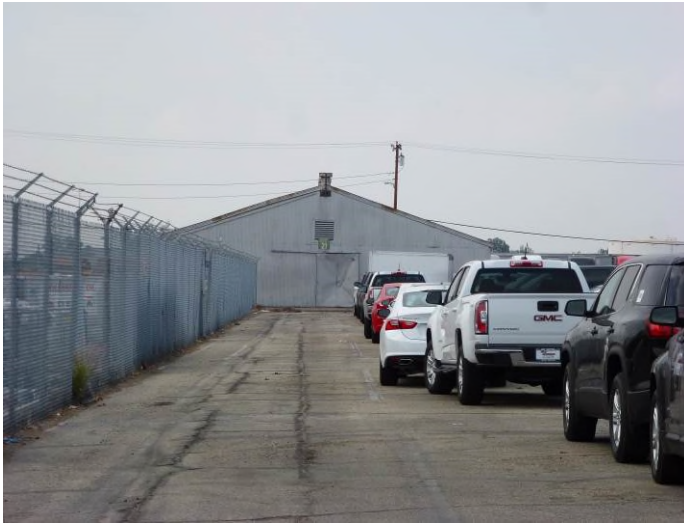
Image 1. View looking west at the east façade.
