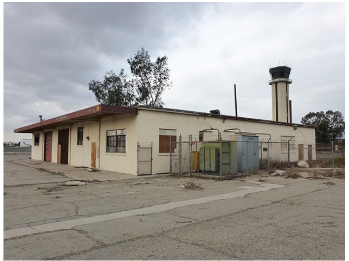
Image 2. View looking northwest at the south and east façades.
