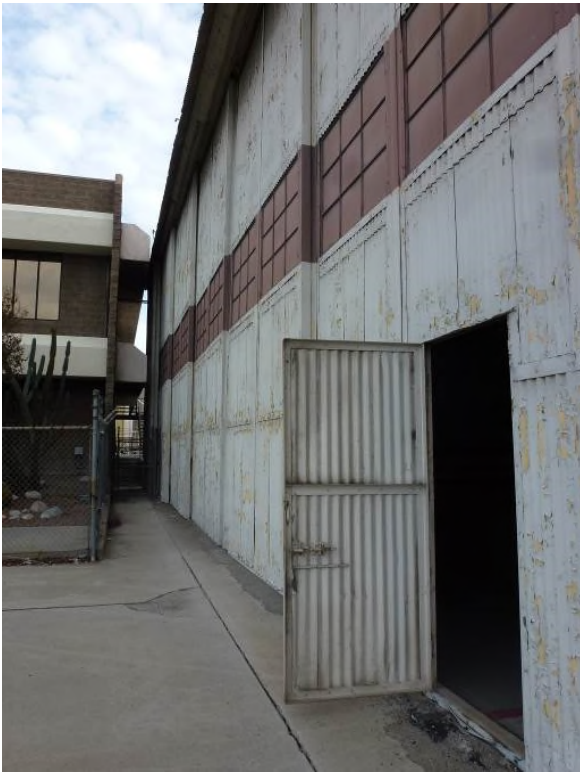
Image 3. Detail view looking at the northwest façade.
