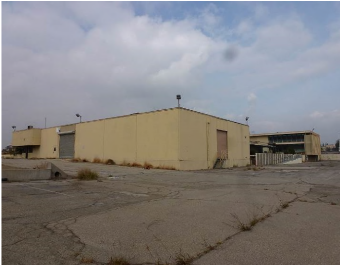
Image 1. View looking northwest at the south and east façades.
