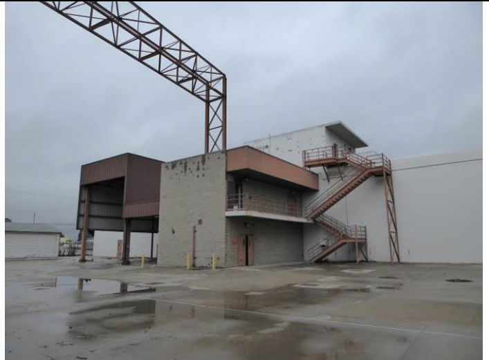
Image 12. View looking northwest at the south façade of Test Cell 2.
