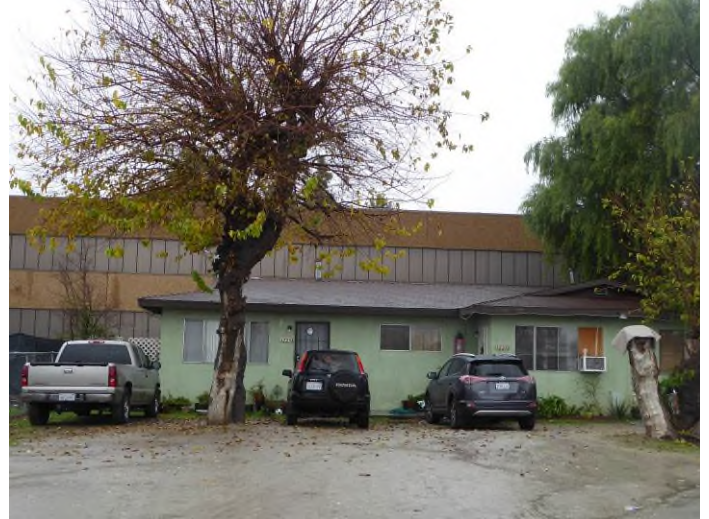
Image 6. View looking southwest at the east and north façades.
