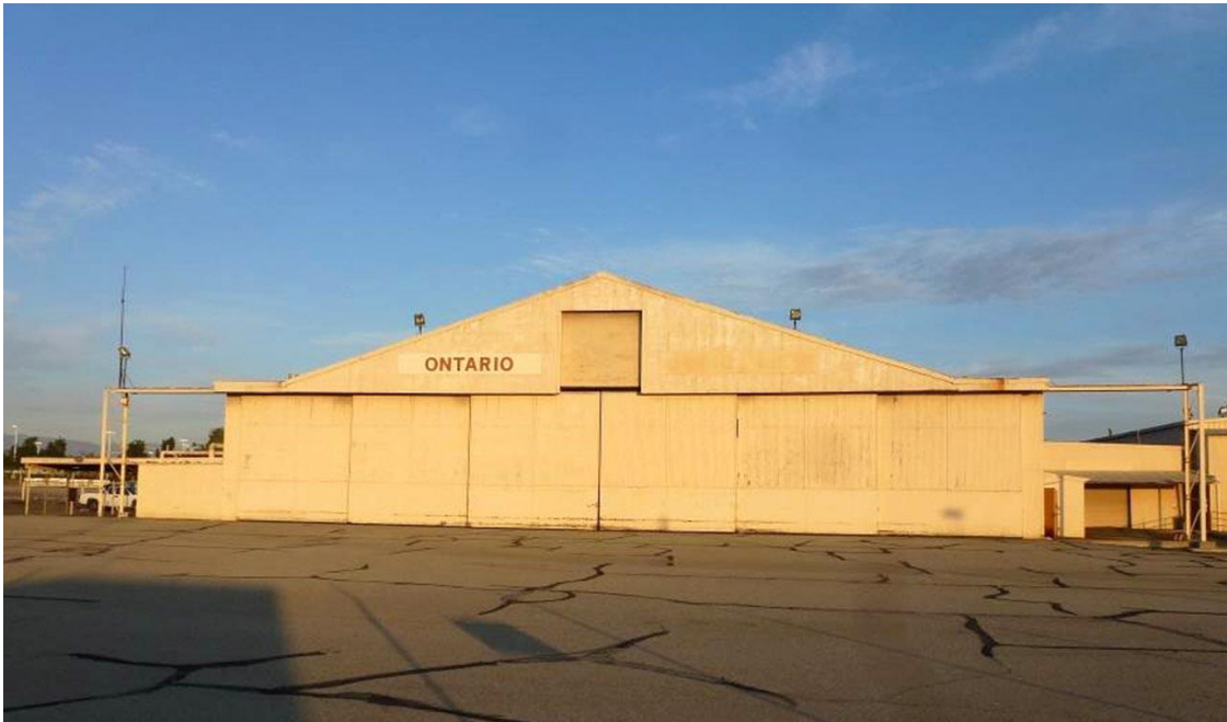
Figure 18. Aerojet-General Hangar, looking east at the west façade. December 6, 2016. Source: ASM.
