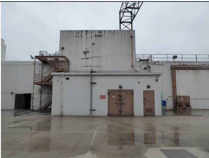
Image 3. Detail view looking south at the north façade of Test Cell 1.
