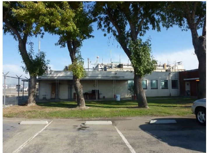
Image 8. View looking east at the west façade of the personnel quarters.
