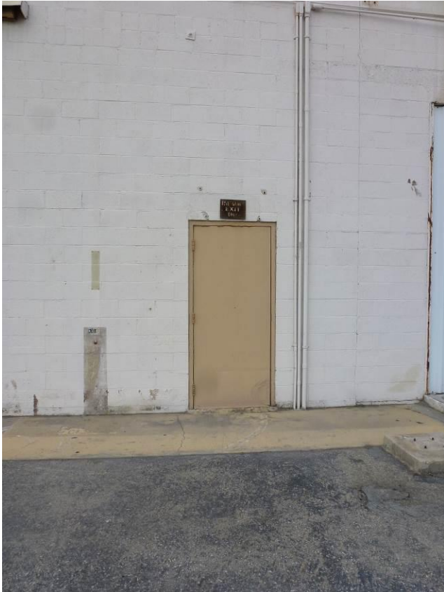
Image 3. Detail view looking west at the east façade.
