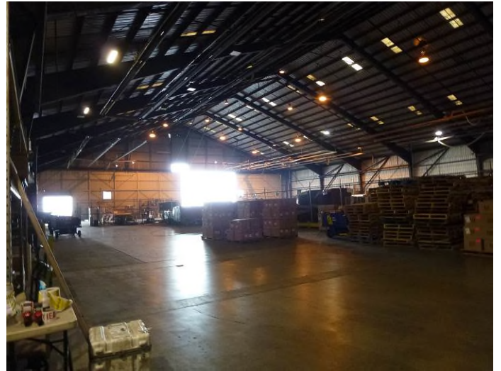
Image 4. Interior view looking southwest.
