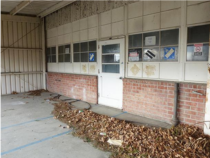
Image 9. Detail view looking northwest at the south façade of the Hangar.
