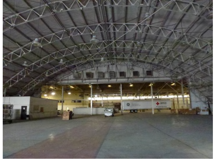
Image 2. Interior view looking northwest.
