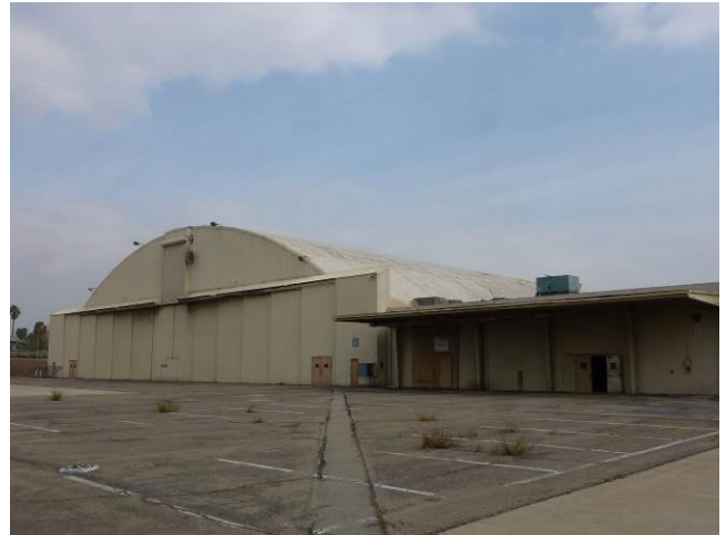
Image 2. View looking northeast at the south and west façades.
