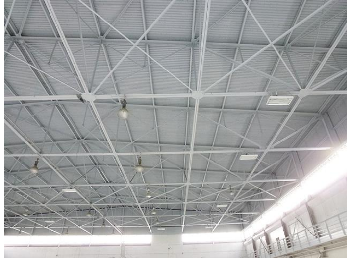
Image 14. Detail view of the interior of the hangar ceiling.
