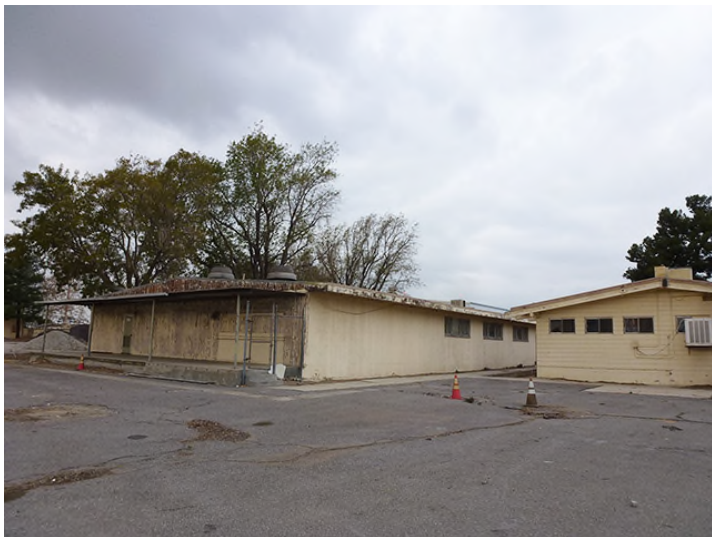
Image 3. View looking northwest at the south and east façades of buildings E and F.
