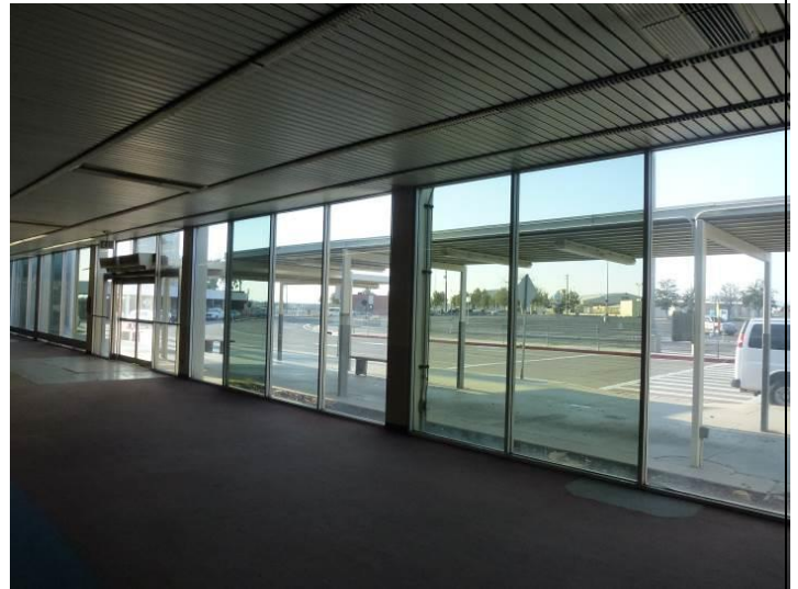
Image 4. Interior view looking west.
