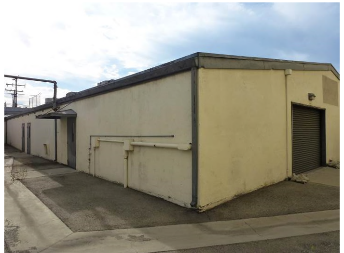
Image 2. View looking south at the northeast and northwest façades of Building E.
