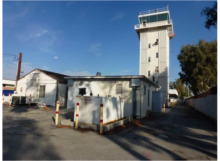
Image 18. View looking northeast at the west façades of the Control Tower and ancillary buildings.
