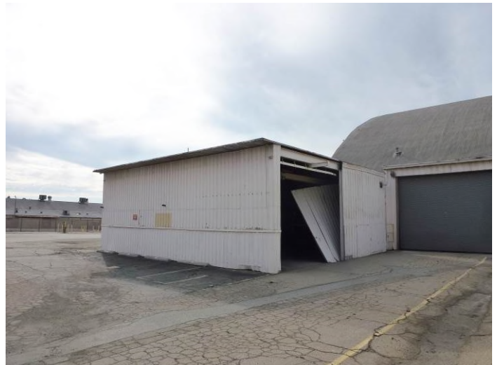
Image 12. View looking south at the northwest and northeast façades of the Wash Building.
