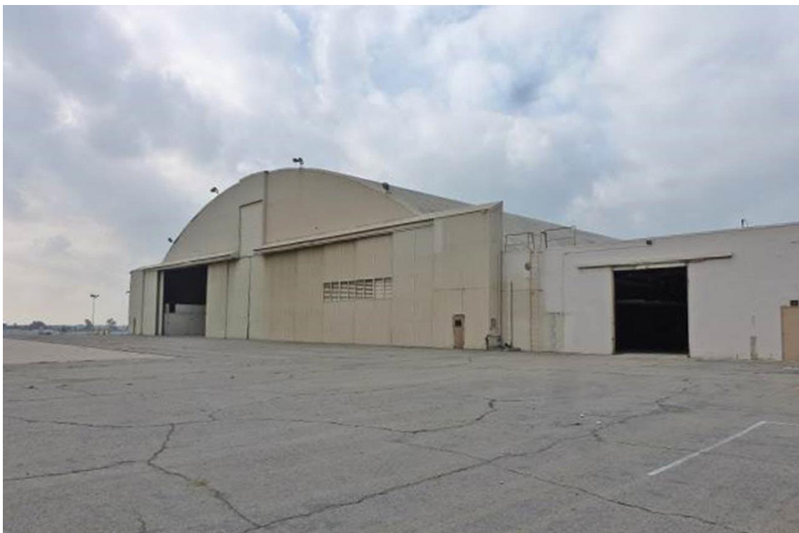
Figure 11. Lockheed Hangar 2, looking southwest. December 6, 2016. Source: ASM.
