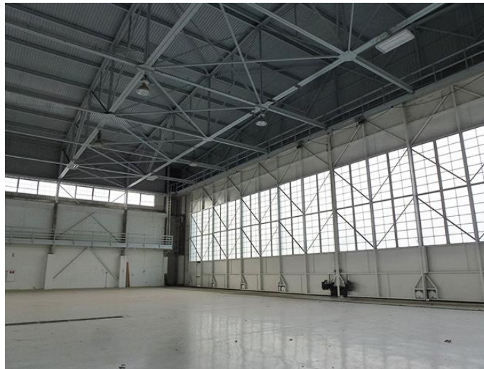
Image 11. Interior view of the hangar looking northwest.
