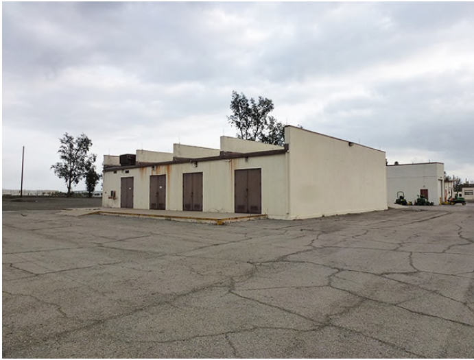
Image 1. View looking southeast at the north and west façades.
