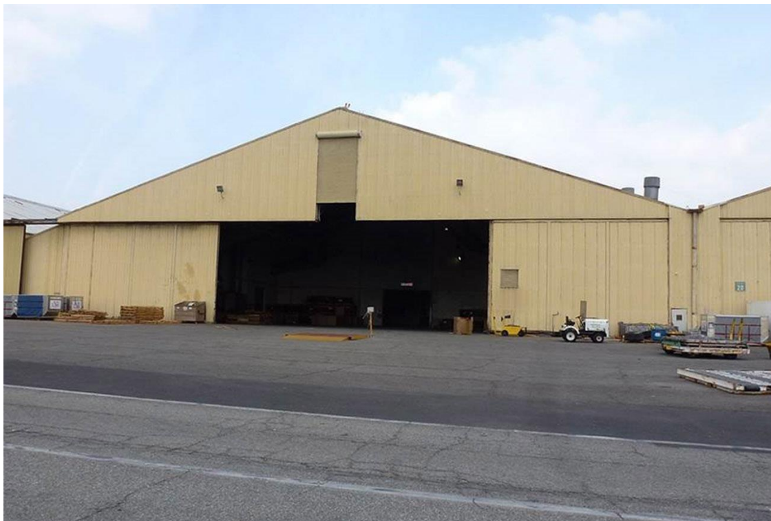
Figure 19. Lockheed Hangar 19, looking south at the north façade. December 6, 2016. Source: ASM.
