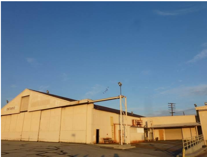
Image 1. View looking northeast at the west and south façades.
