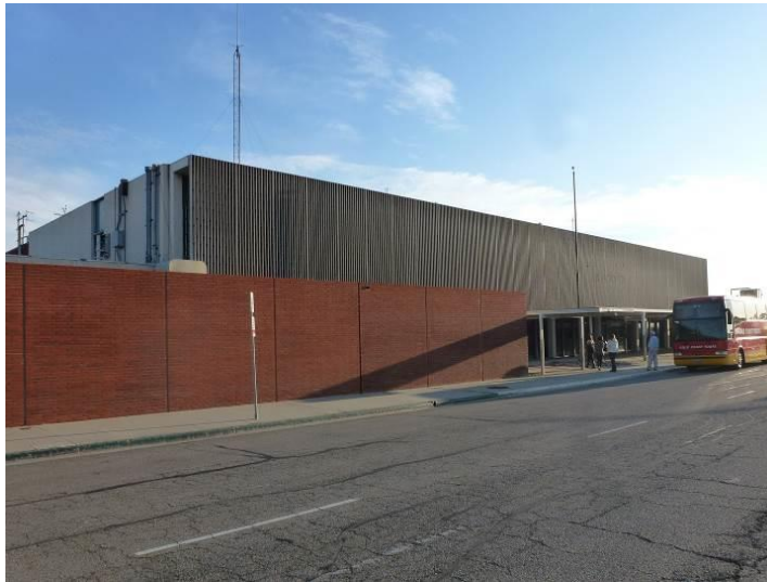
Image 3. View looking south at the northeast and northwest façades.
