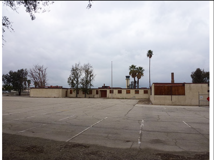
Image 4. View looking north at the south façade.
