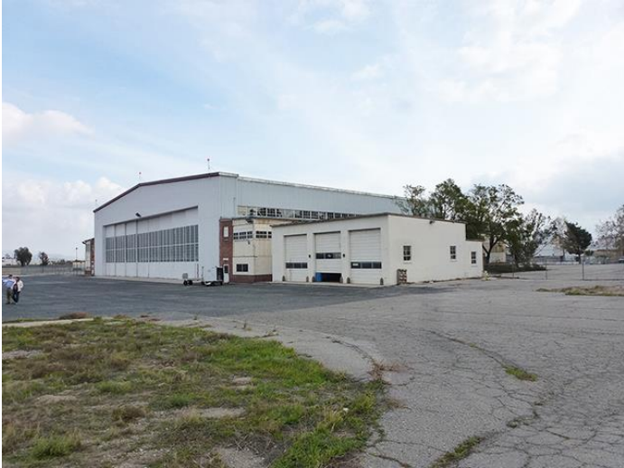
Image 1. View looking southeast at the north and west façades, with Fire Station in the foreground.
