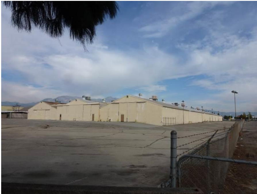
Image 4. View looking north at the southwest and southeast façades of the Storage Hangars. ASM, December 1, 2016.
