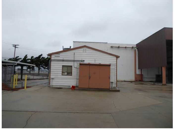
Image 10. View looking north at the south façade of the Guard House.
