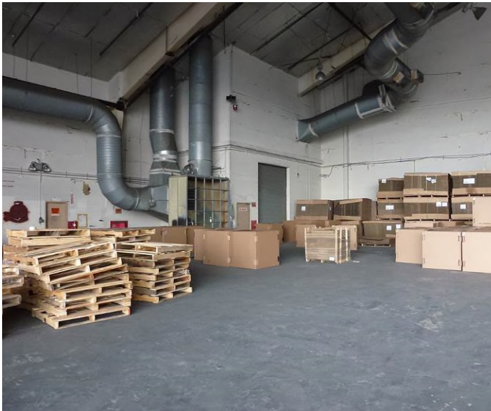
Image 3. Interior view looking northwest.
