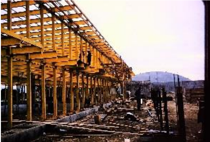
Image 9. View looking northeast at the south façade, ca. 1956. Source: Collection of Colin Russell.
