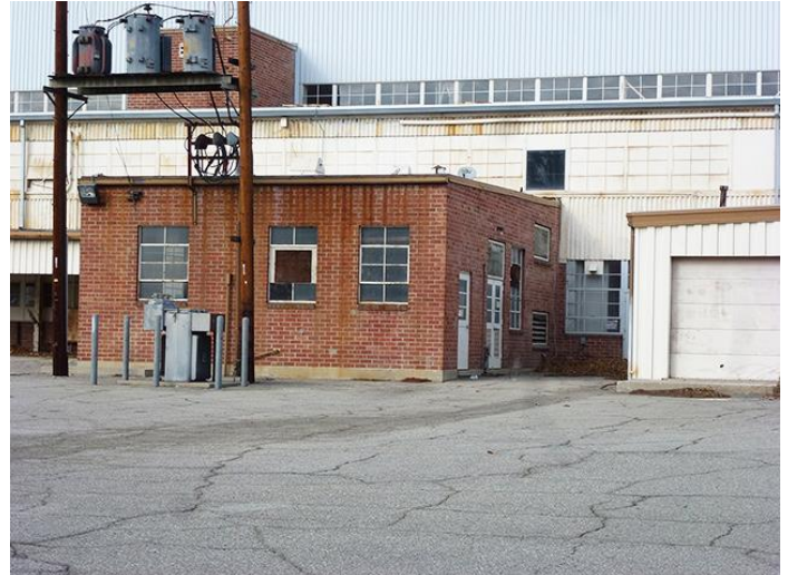
Image 6. View looking northwest at the south and east façades of the Diesel Tanks room.
