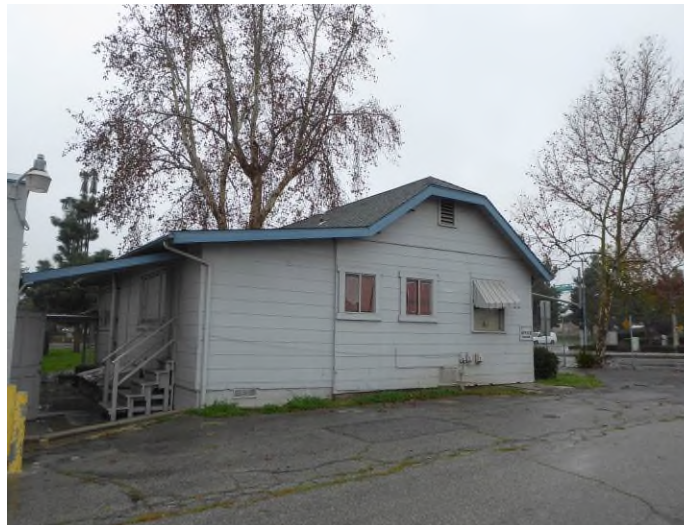
Image 3. View looking northwest at the south and east façades.
