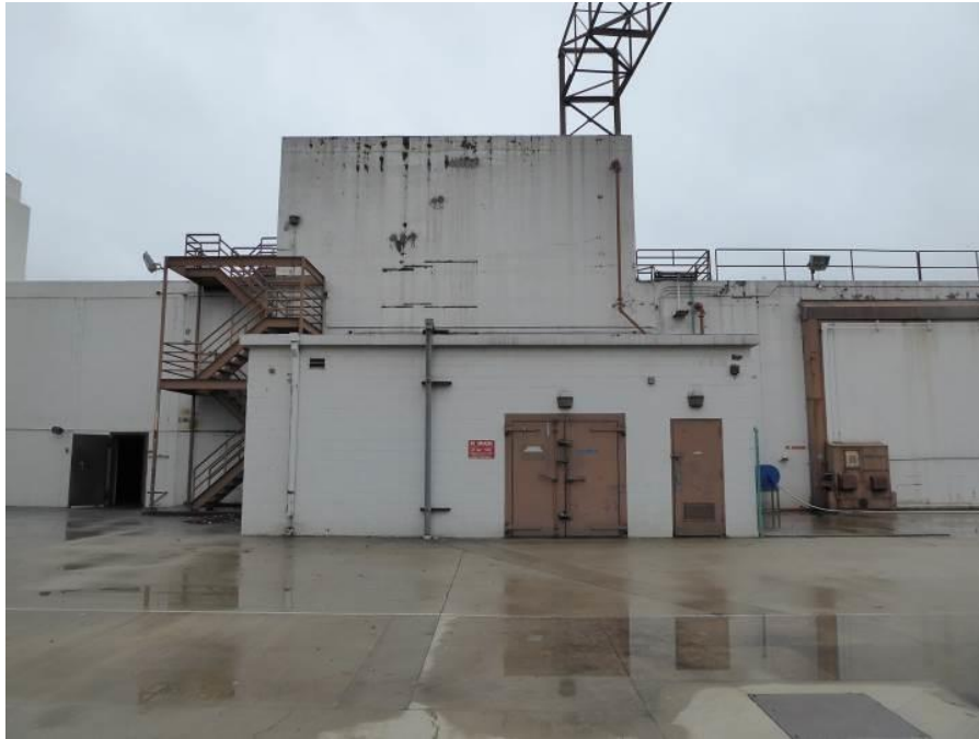
Image 5. View looking east at the Jet Engine Test Cell area. ASM, December 1, 2016.
