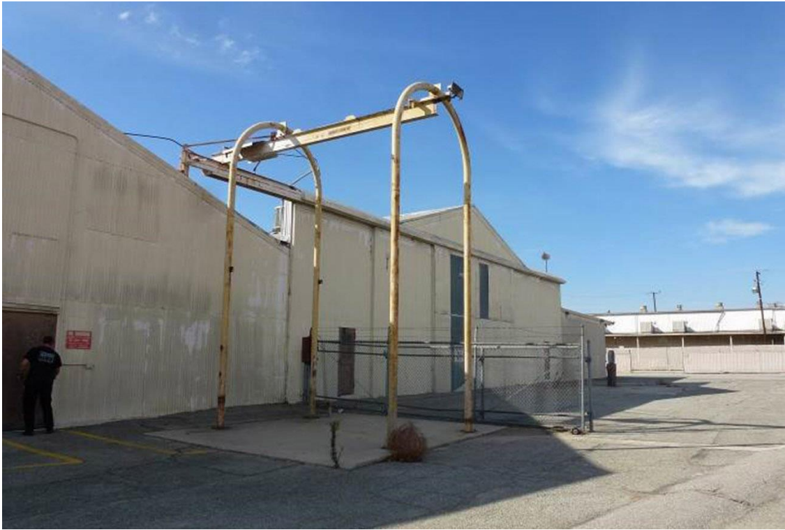
Figure 15. GE storage hangars, looking west at northeast façade, December 6, 2016. Source: ASM.
