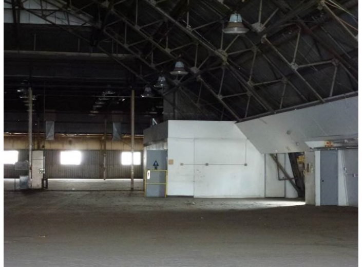
Image 6. Interior view looking southeast.
