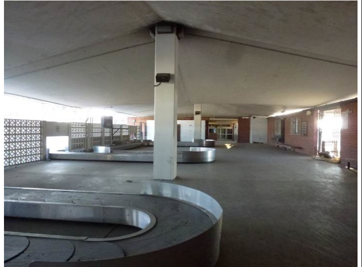
Image 4. Interior view looking west.
