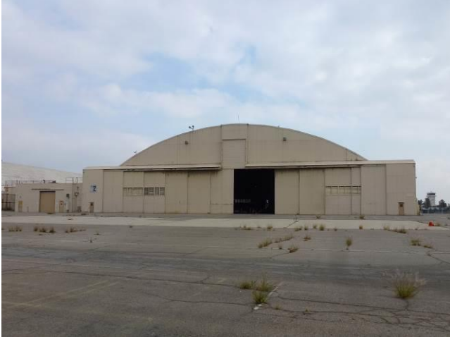
Image 1. View looking north at the south façade.
