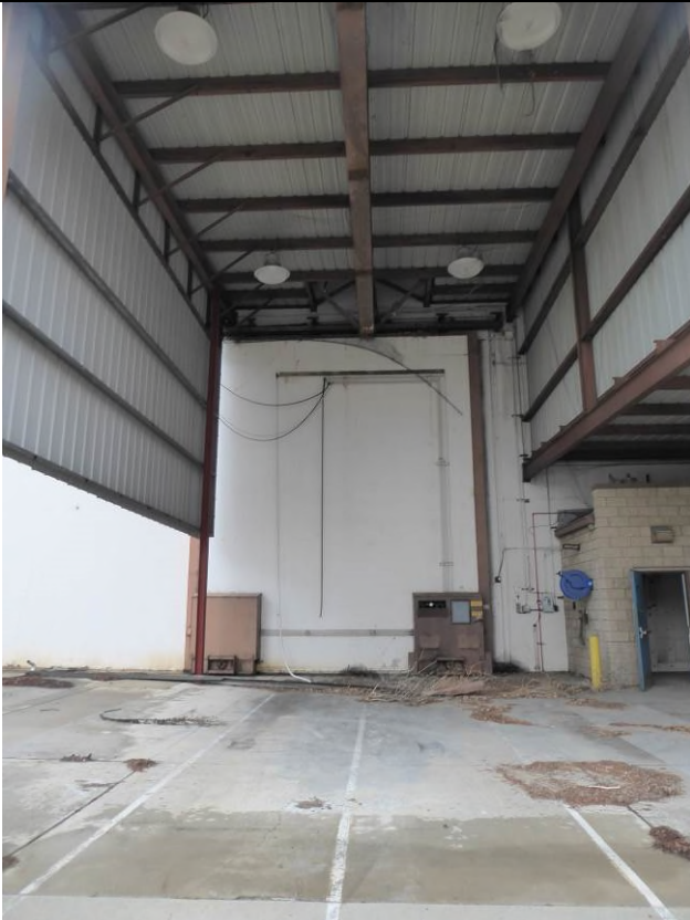
Image 15. Detail viewing looking north at the south façade of Test Cell 2.
