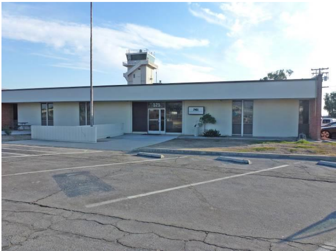
Image 6. View looking south at the north façade of the FAA building. This building is recommended as a contributor to the historic district.
