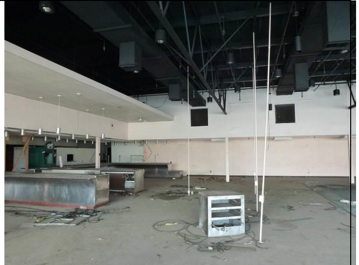
Image 4. Interior view looking southwest.
