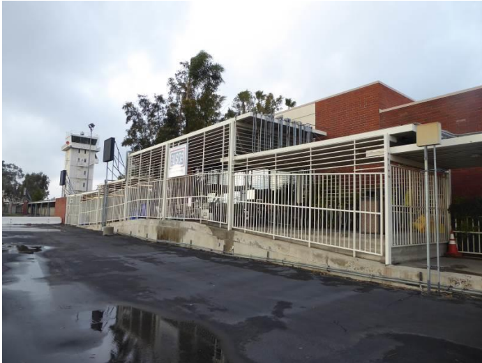
Image 5. View of Control Tower looking west from runway. As a later addition to the terminal, this portion of the building does not contribute to the historical significance of the building.
