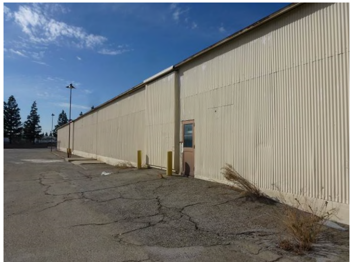
Image 4. Detail view looking west at the southeast façade.
