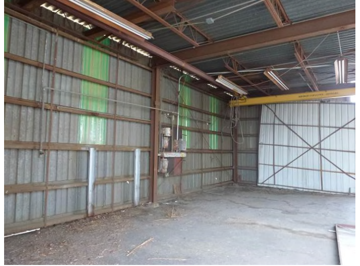
Image 14. Interior view of the Wash Building.
