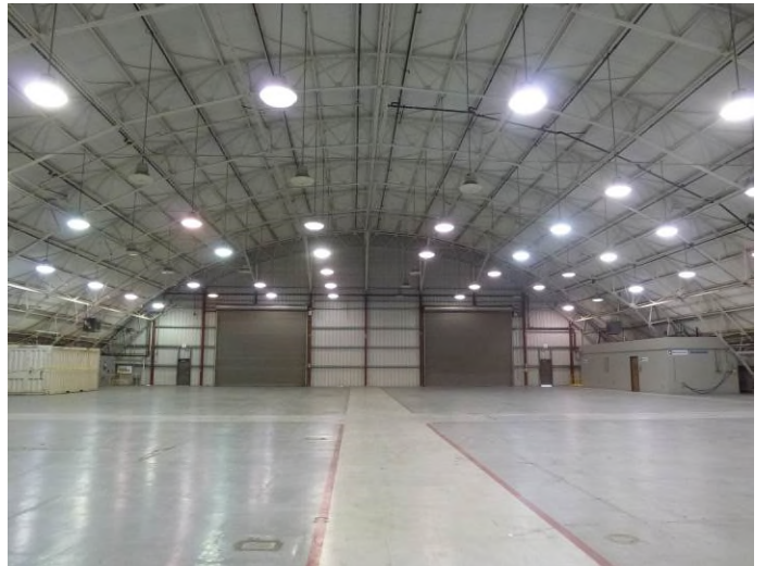
Image 4. Interior view looking southeast.
