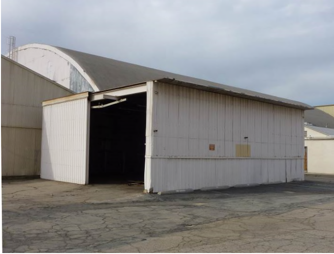
Image 13. View looking north at the southwest and southeast façades of the Wash Building.
