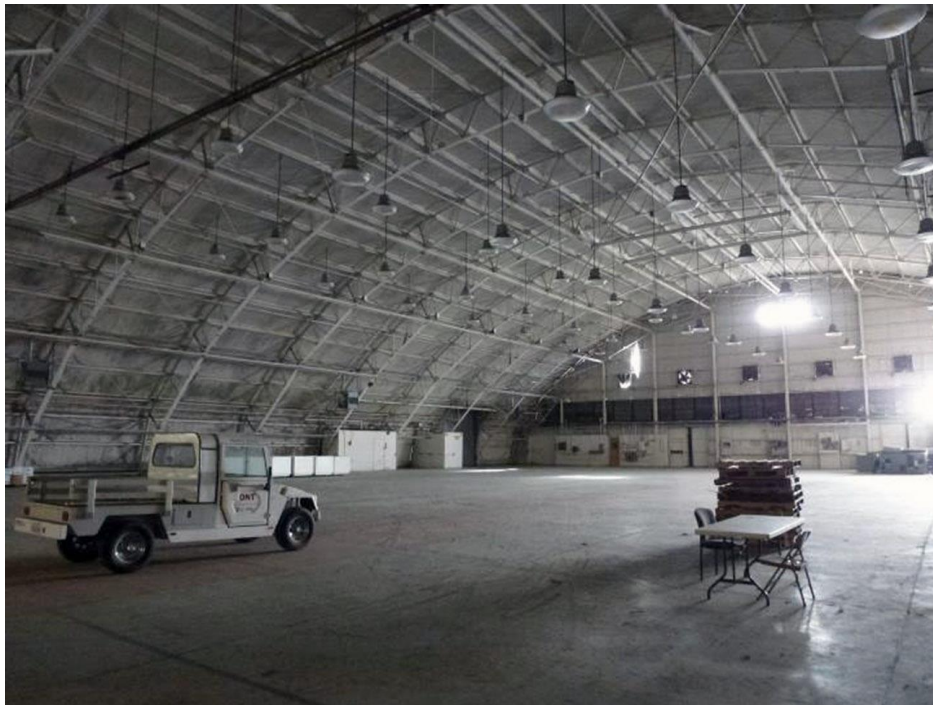
Figure 14. Interior of GE Engine Hangar 3. December 6, 2016. Source: ASM.
