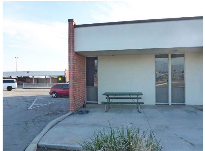
Image 4. Detail view looking at the north façade.
