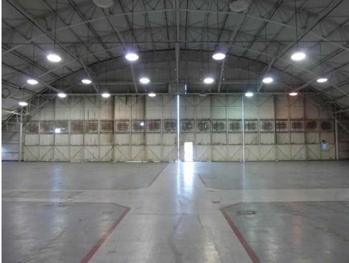
Image 5. View of the interior looking northwest.
