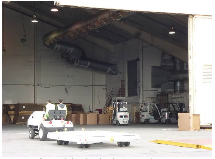
Image 2. Interior view looking northeast.
