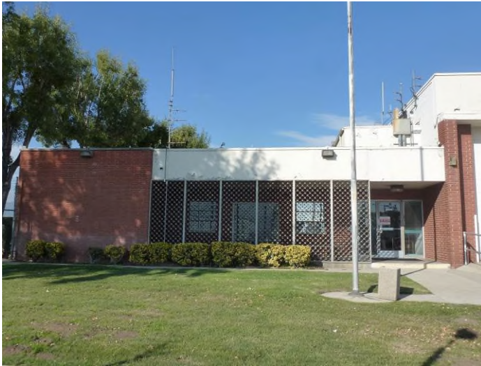
Image 3. Detail view looking at the south façade.
