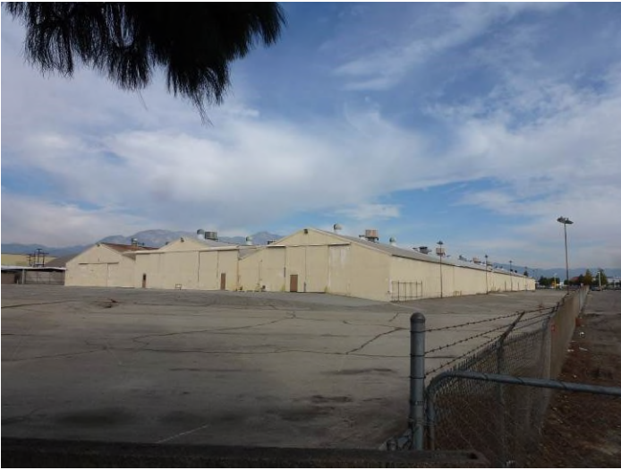
Image 1. View looking north at the southwest and southeast façades.
