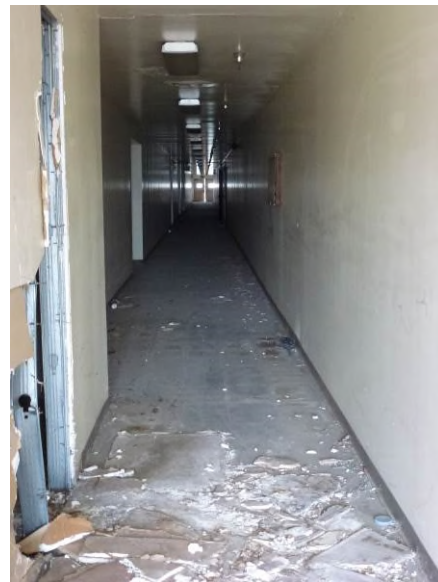
Image 4. View of the interior looking west.
