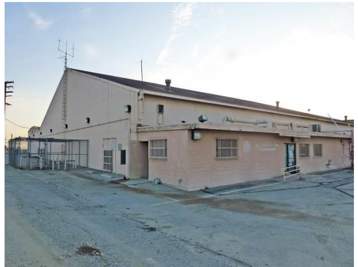
Image 2. View looking southwest at the east and north façades.
