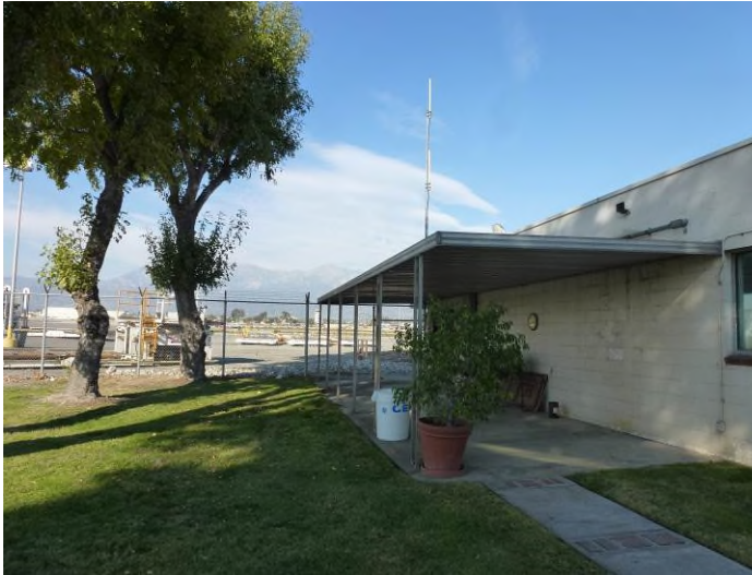
Image 9. Detail view looking northeast at the west façade.
