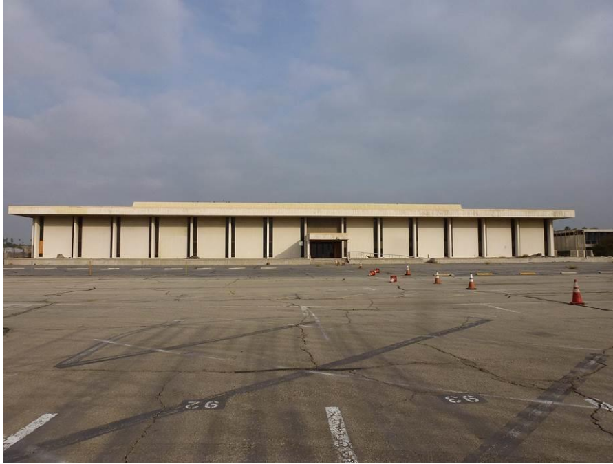
Image 1. View looking north at the south façade of Building 15.
