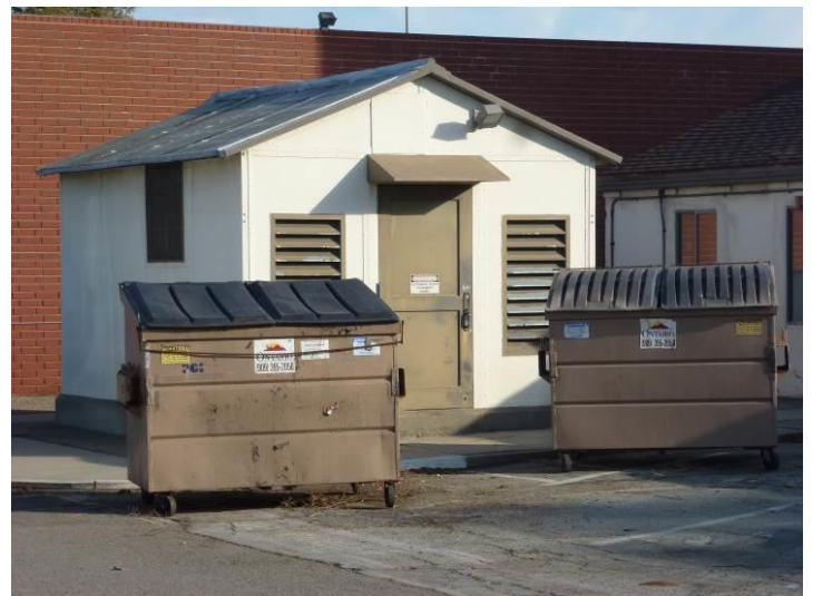
Image 12. View looking southeast at north and west façades of ancillary building to the north of the control tower.
