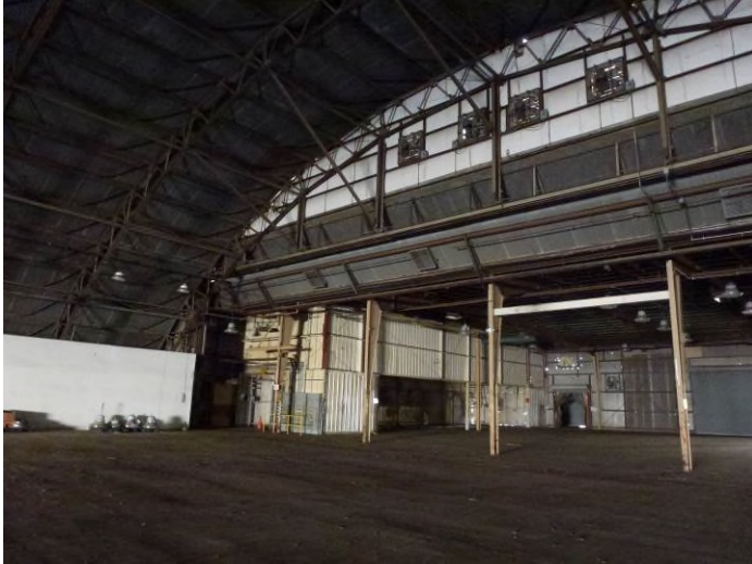
Image 5. Detail interior view looking east.
