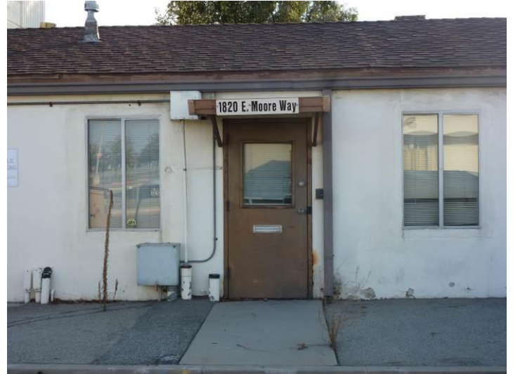
Image 10. View looking south at the north façade of ancillary building north of the control tower.
