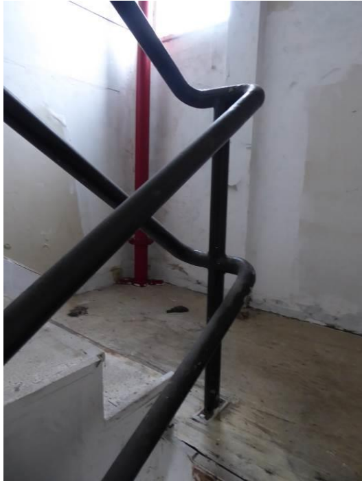
Image 5. Detail view of the interior staircase.
