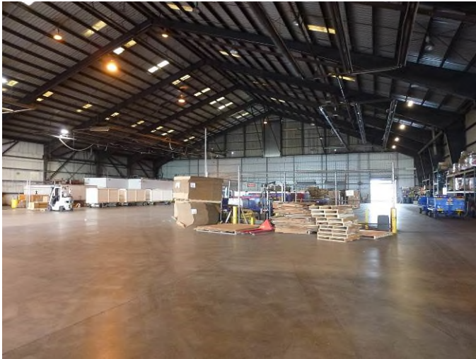
Image 3. Interior view looking north.
