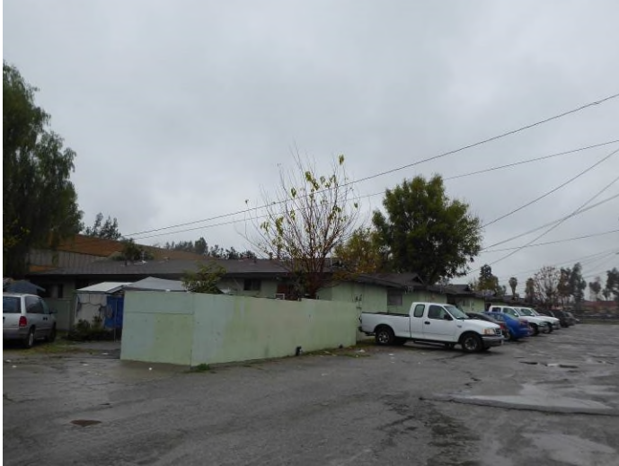
Image 5. View looking northwest at the south and east façades.
