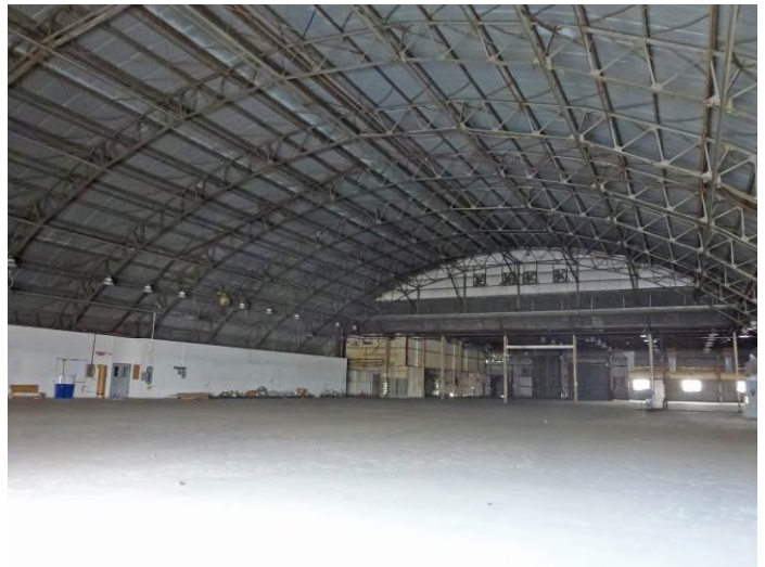
Image 4. Interior view of Hangar 4 looking southeast.
