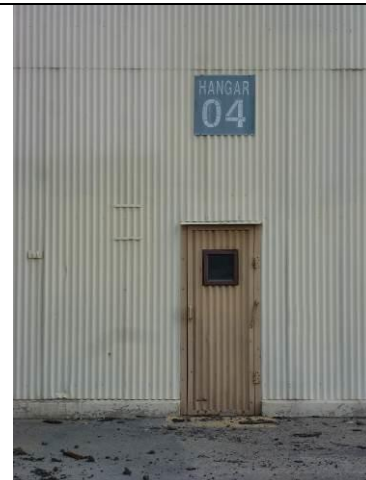
Image 6. Detail view looking east at west façade.
