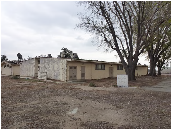
Image 1. View looking southeast at the north and west façades.
