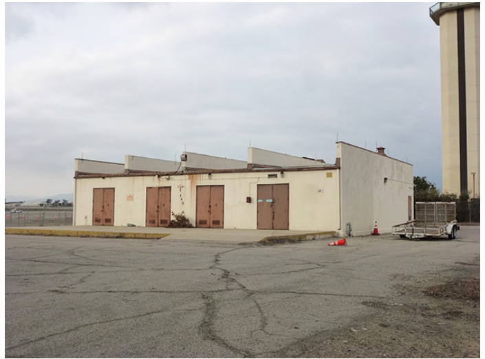
Image 4. View looking northwest at the south and east façades.
