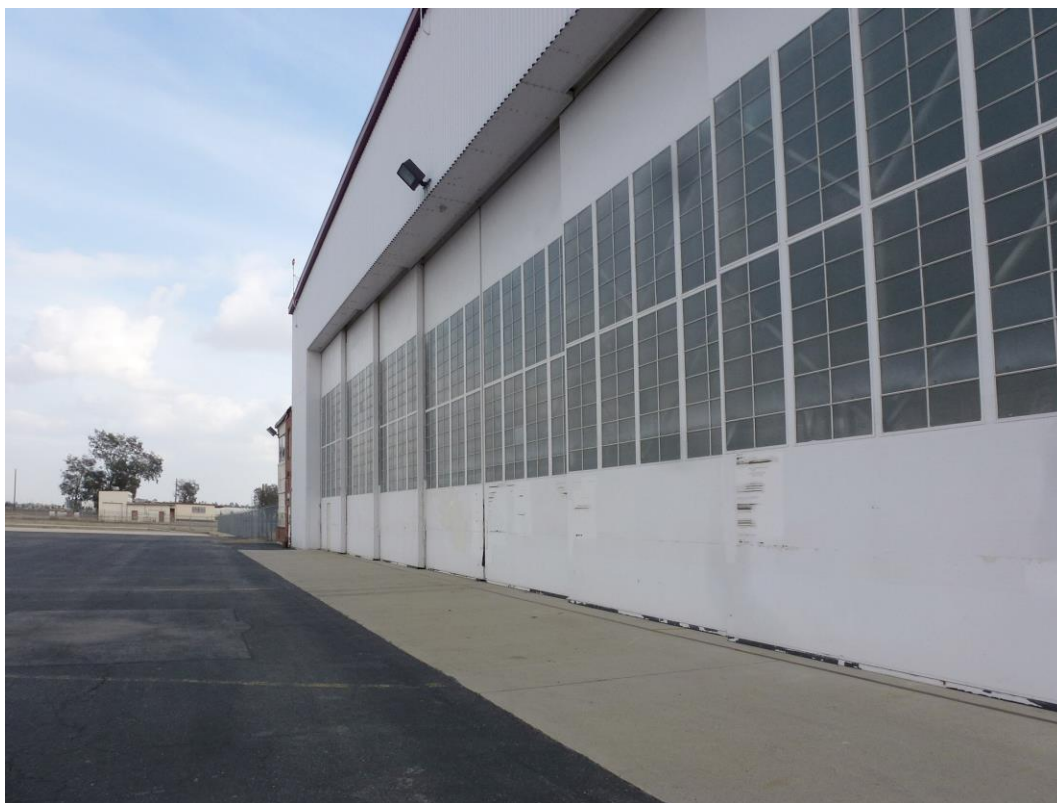
Figure 32. Multi-leaved doors on ANG Hangar. December 6, 2016.
