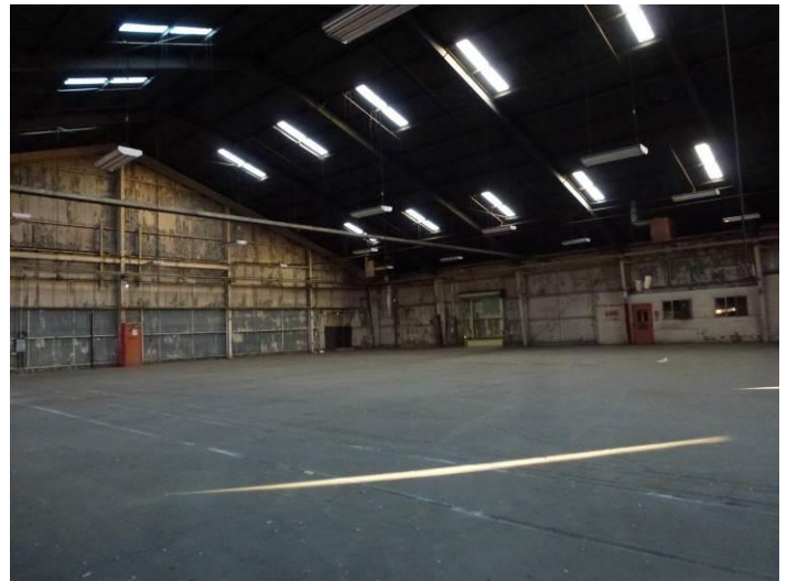
Image 4. Interior view looking southeast.
