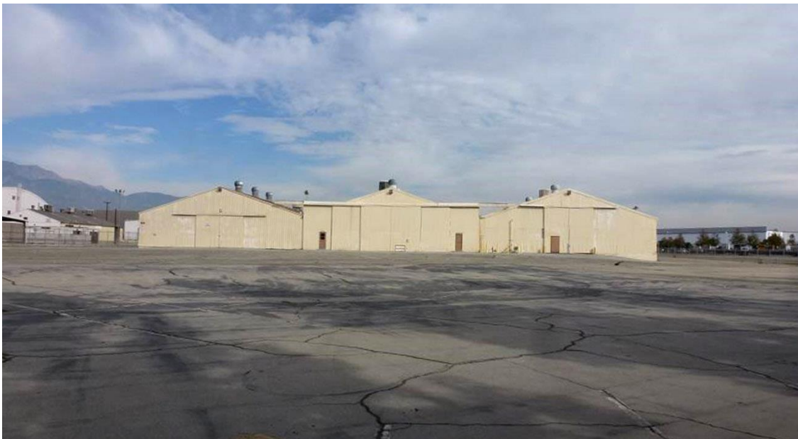
Figure 16. GE storage hangars, looking north at south façade, December 6, 2016. Source: ASM.
