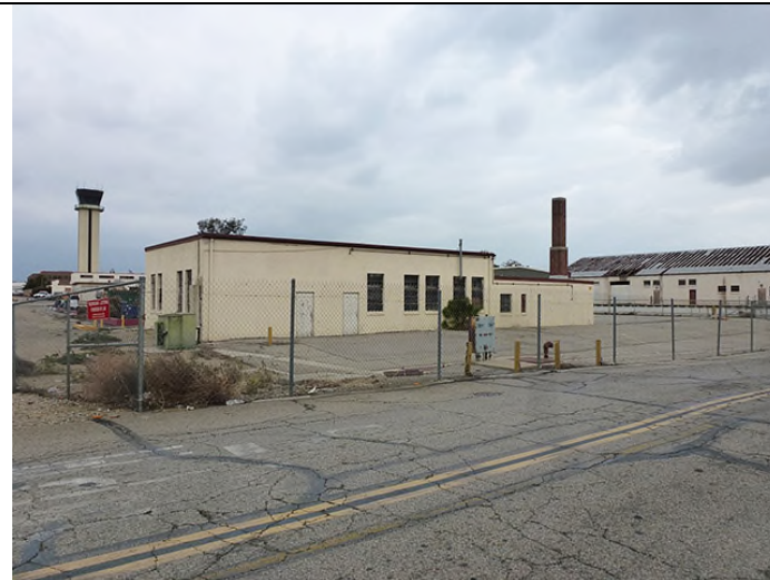
Image 3. View looking northeast at the west and south façades.
