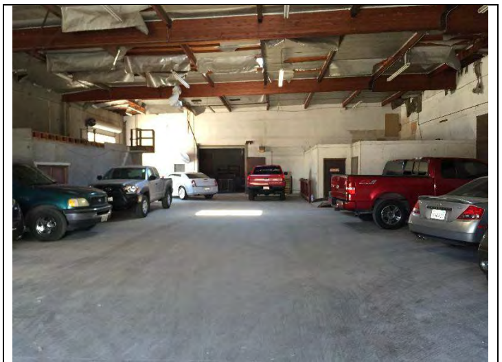
22. View of Interior Parking/Garage area within Main building (Building A)
