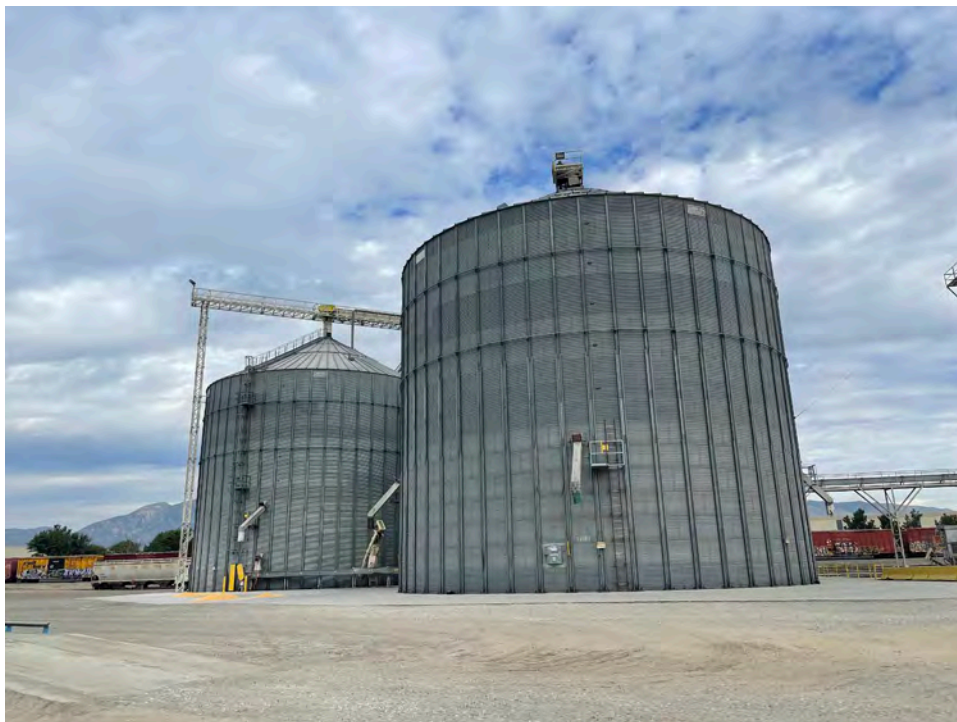
Photograph 10: Scoular grain storage silos.
