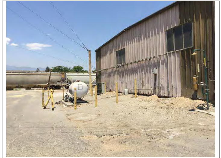
2. View of Warehouse Building (Building C)
