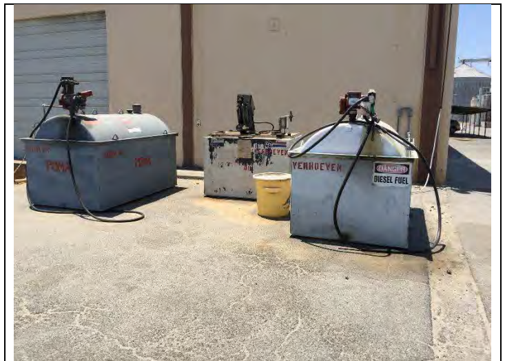
12. View of Diesel ASTs and Hydraulic Oil AST near Main Building (Building A)
