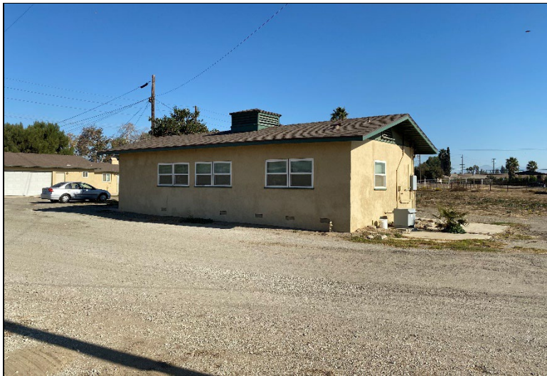
Figure 4. Eastern façade (view west; December 13, 2023).
