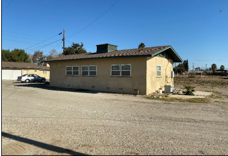
Figure 4. Eastern façade (view west; December 13, 2023).
