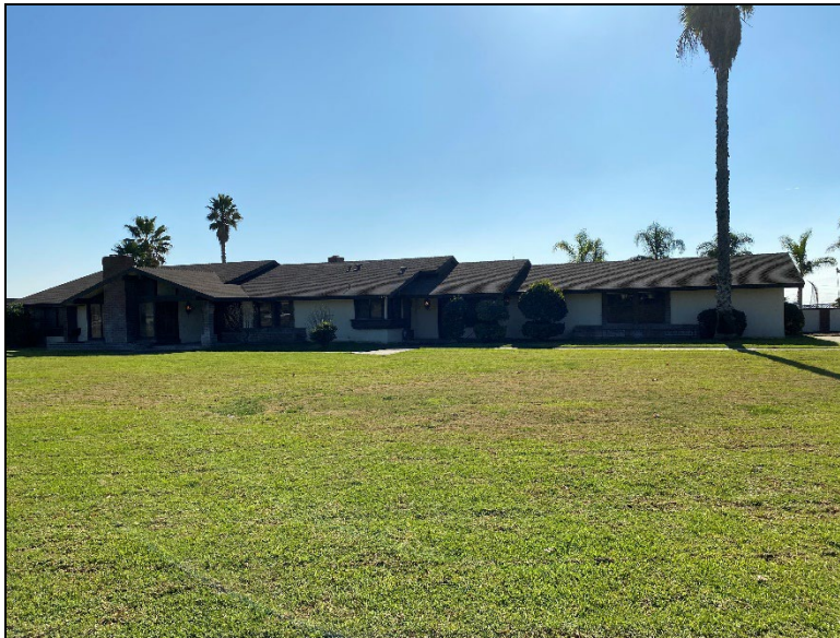
Figure 7. Northern façade (view south; December 13, 2023).
