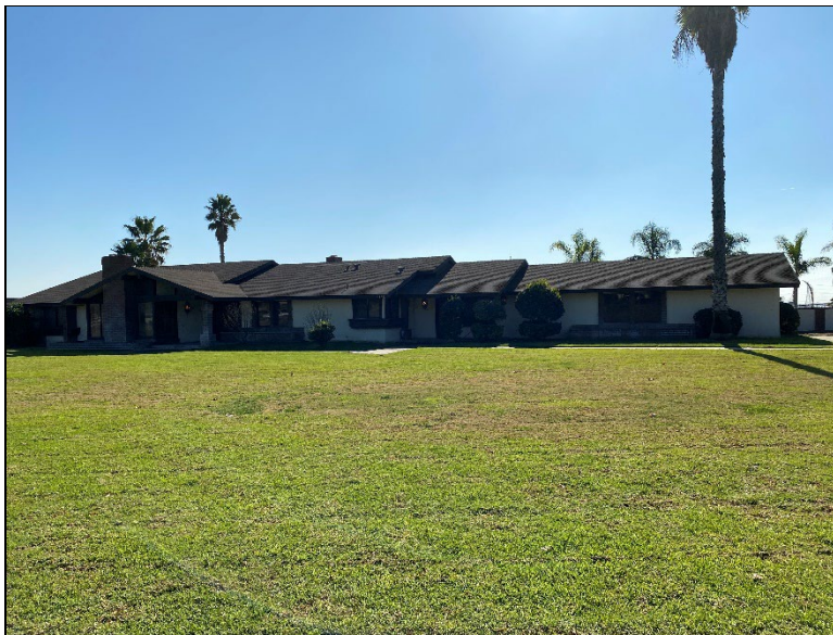
Figure 7. Northern façade (view south; December 13, 2023).
