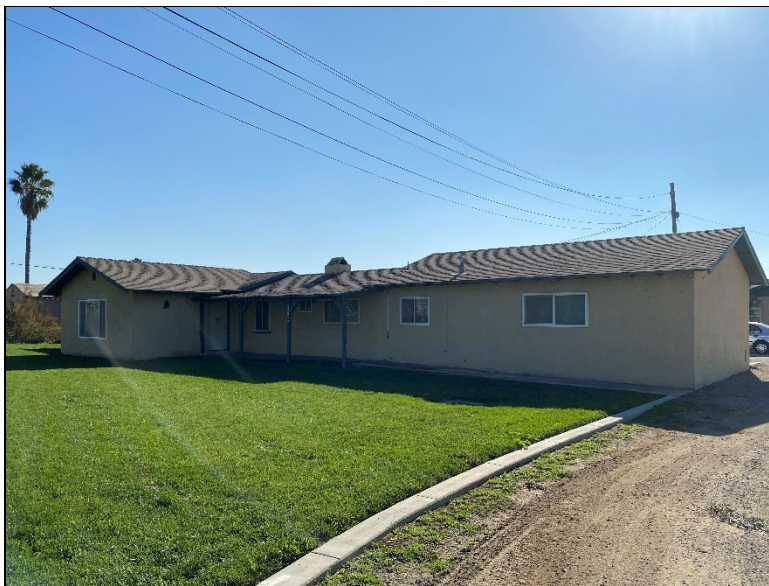
Figure 3. Northern façade (view southeast; December 13, 2023).
