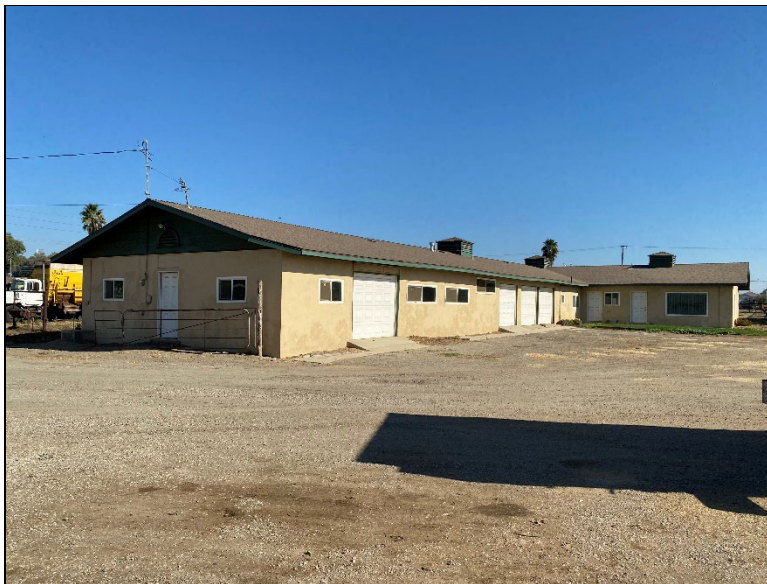
Figure 5. Western and Southern façades (view southwest; December 13, 2023).
