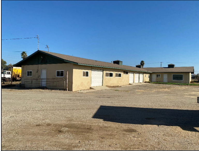
Figure 5. Western and Southern façades (view southwest; December 13, 2023).
