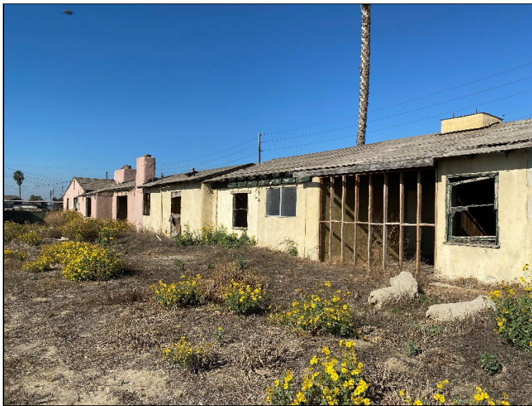
Figure 2. Southern façade (view northwest; December 13, 2023).
