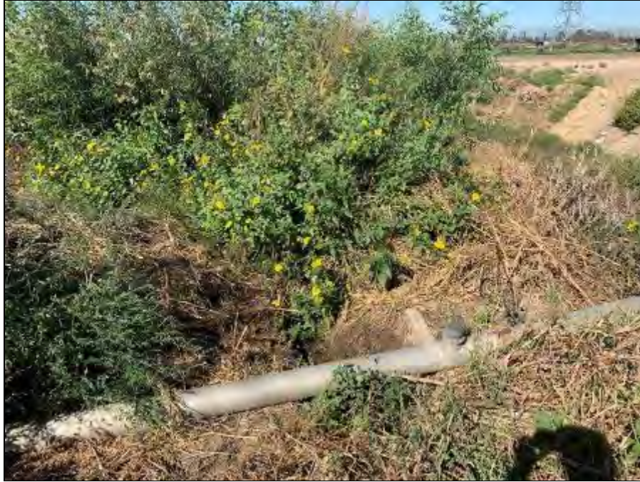
Photo 21. Irrigation Pipes Feeding into the Excavated Basin located north of Edison Avenue and within the Project Area.
