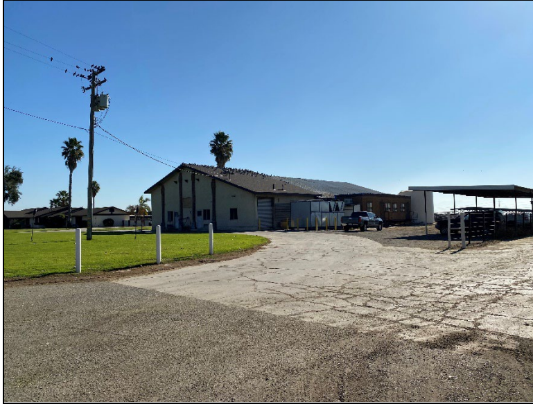
Figure 8. Northern façade (view southeast; December 13, 2023).
