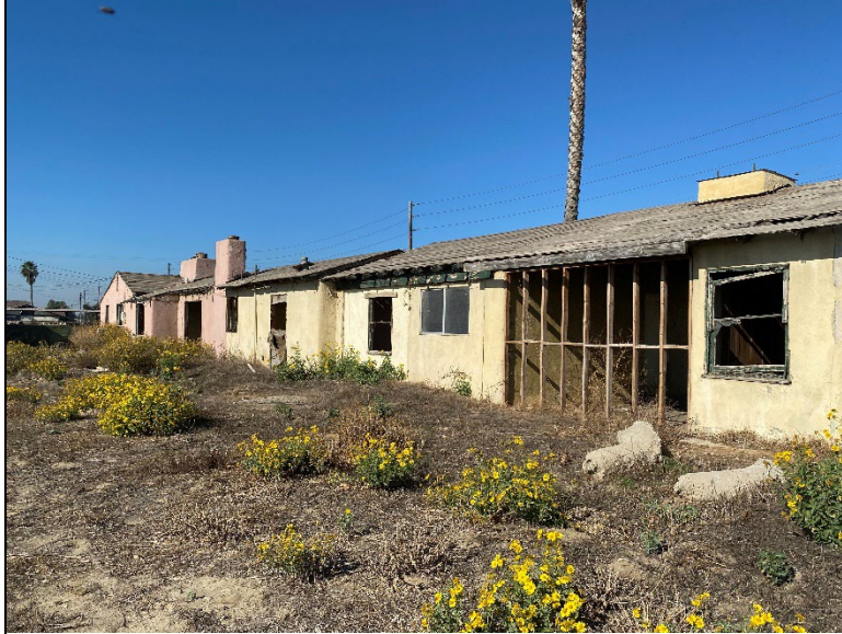
Figure 2. Southern façade (view northwest; December 13, 2023).
