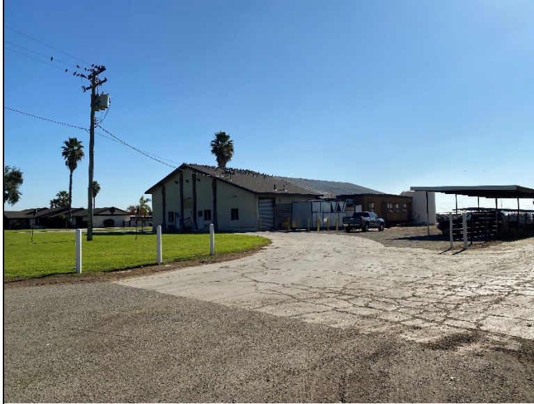
Figure 8. Northern façade (view southeast; December 13, 2023).
