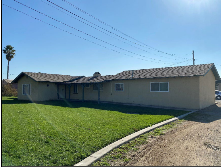
Figure 3. Northern façade (view southeast; December 13, 2023).
