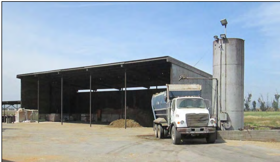
Dry feed sorter. View looking southwest.
