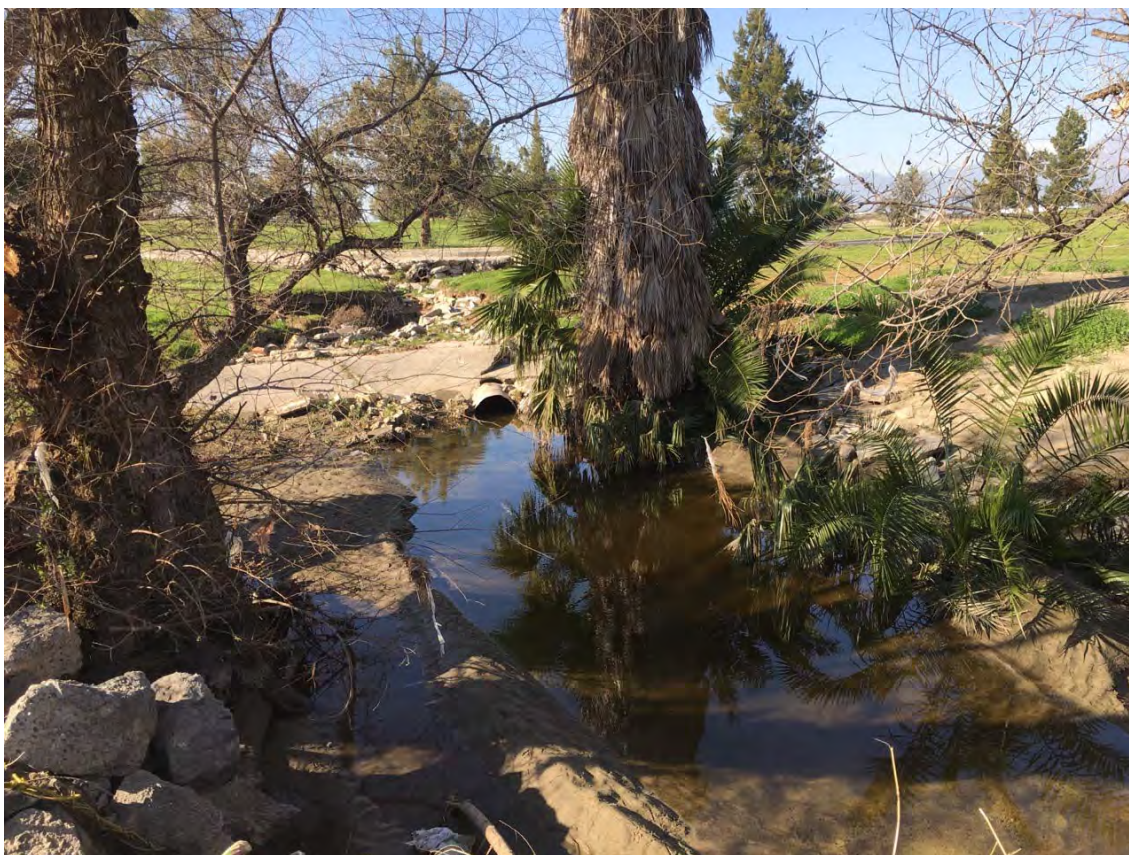
Overview of P-36-024903 including modern culverts, facing north.
