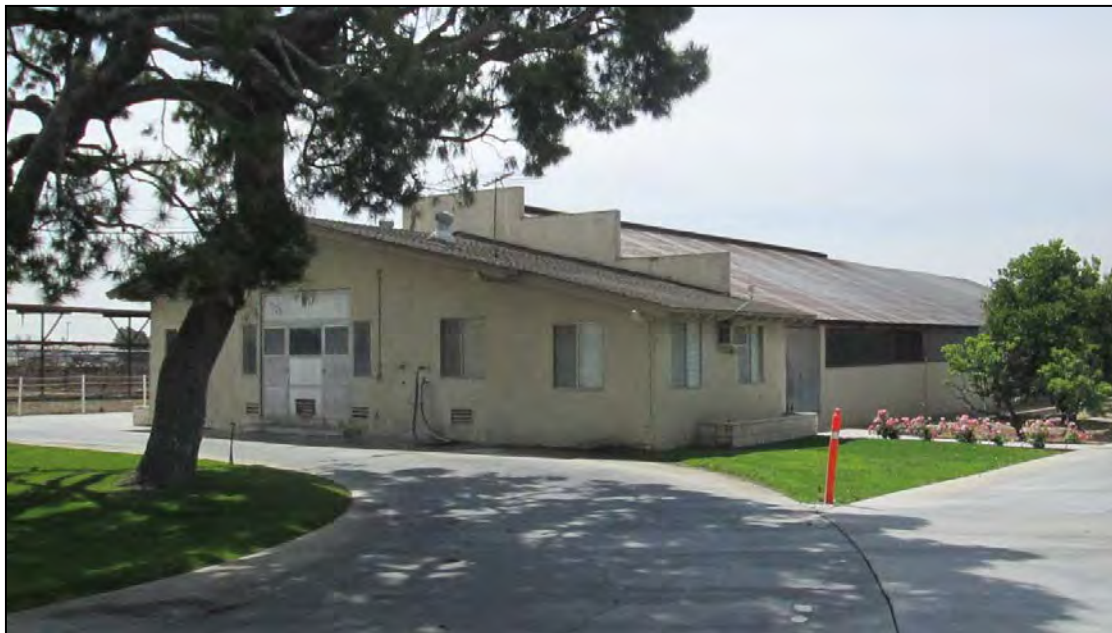
North (front) and west elevations of Main Dairy Barn. View looking southeast.
