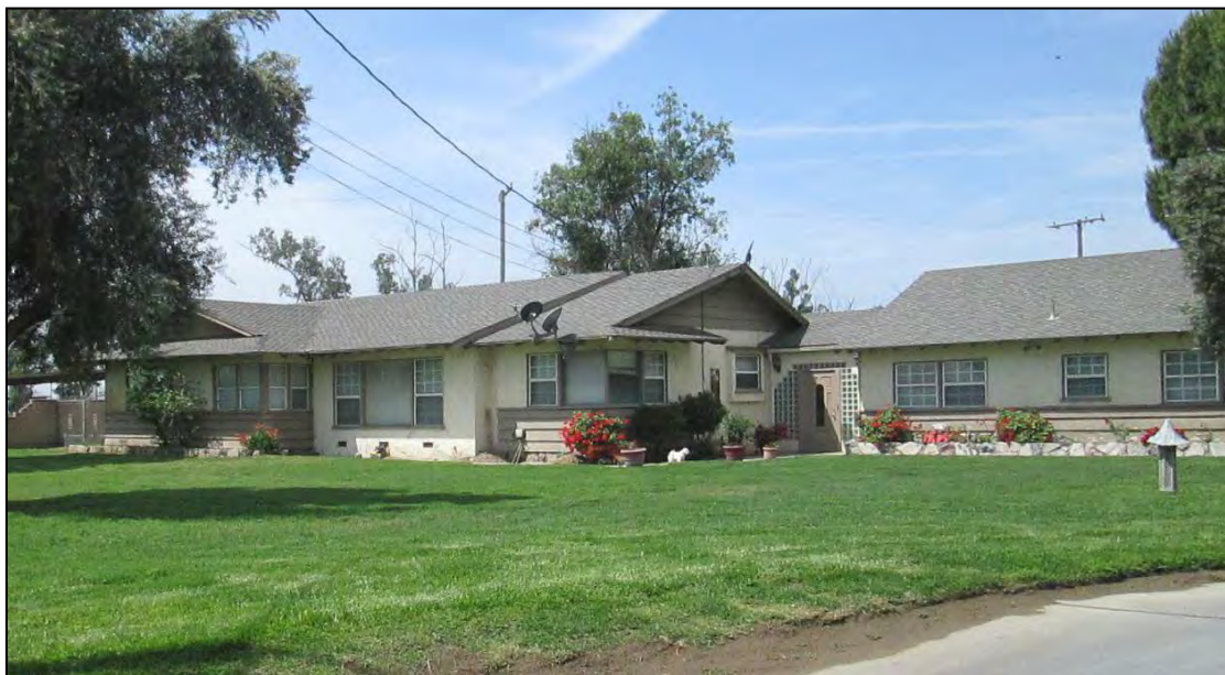
Boersma-Borba House. View looking southwest.
