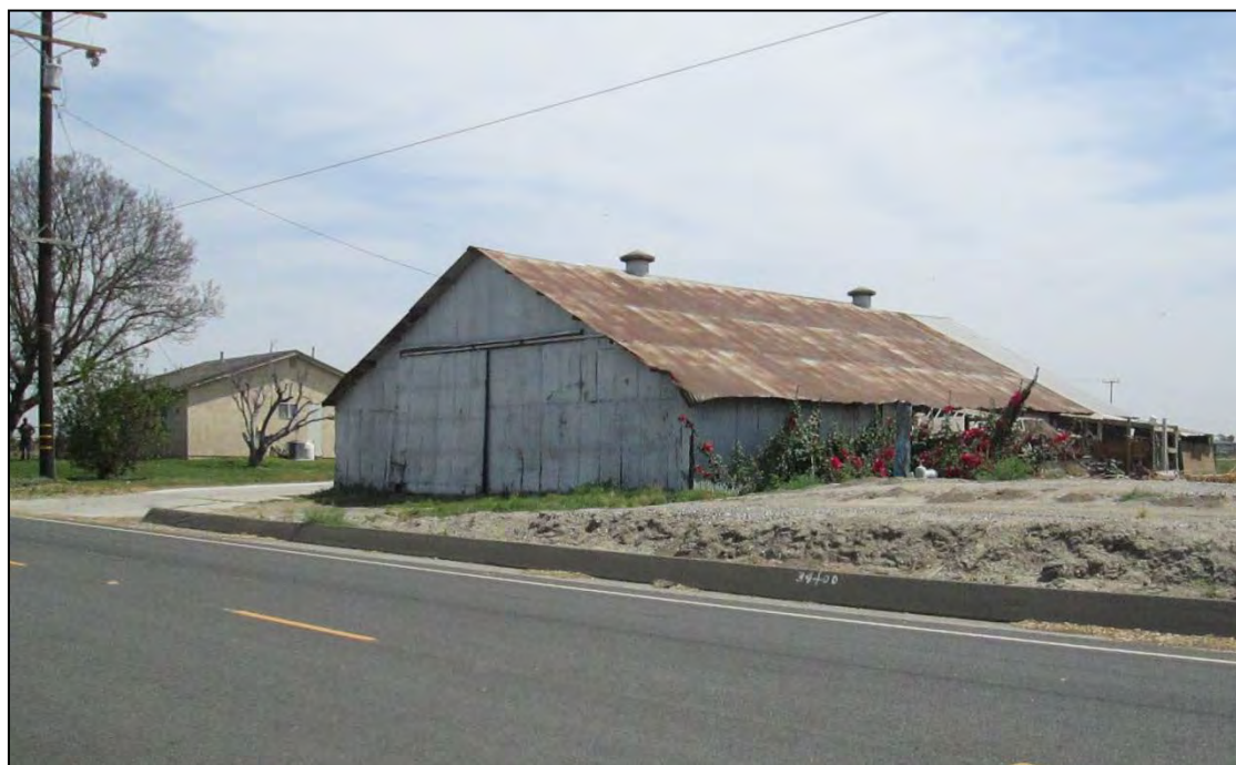
Storage barn. View looking northeast.
