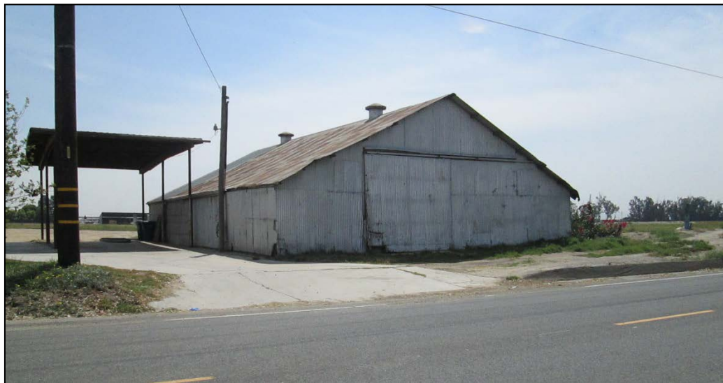
Storage barn. View looking southeast.
