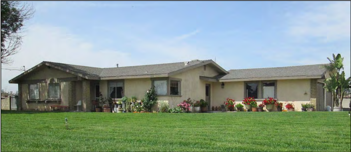
Farm manager's house. View looking west.
