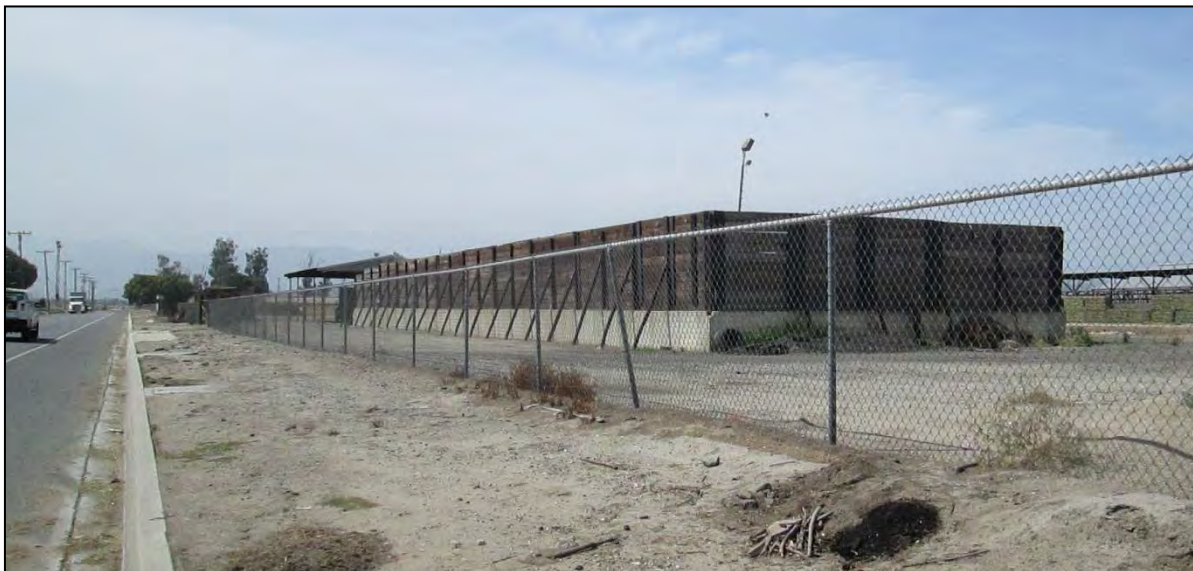
Dry manure-holding structure on South Grove Ave. View looking south.
