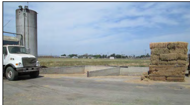
Wet food mixing bay. View looking northwest.
