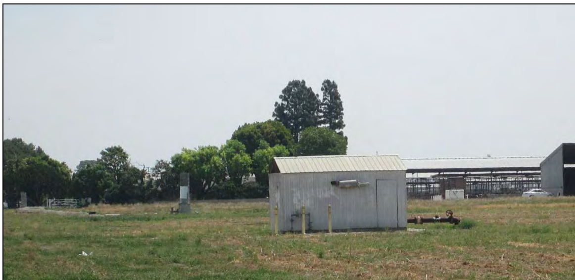
Water pump located west of Main House, along Eucalyptus Ave. View looking east.
