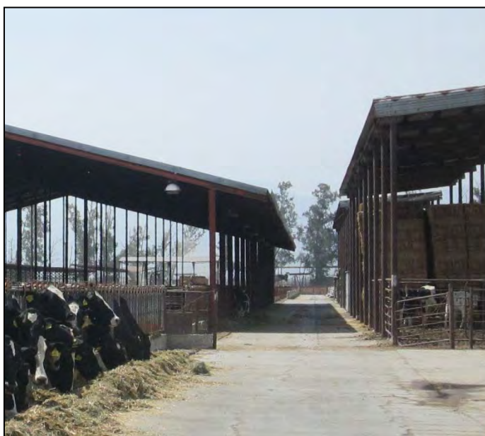
Hay shed (left) across from gable cow shade structure. View looking south.
