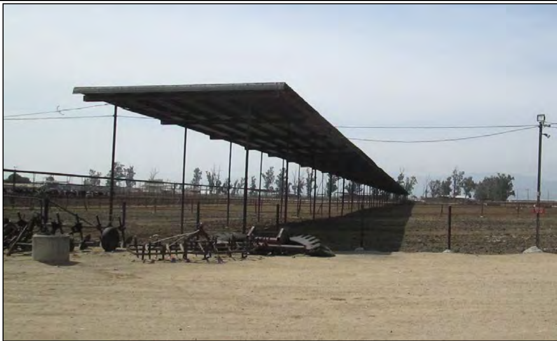
Cattle shade east of Main Dairy Barn. View looking south.
