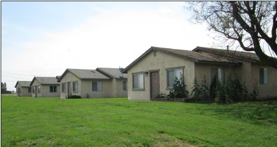
Single-family residences, built by Borba in 1988. View looking southeast.
