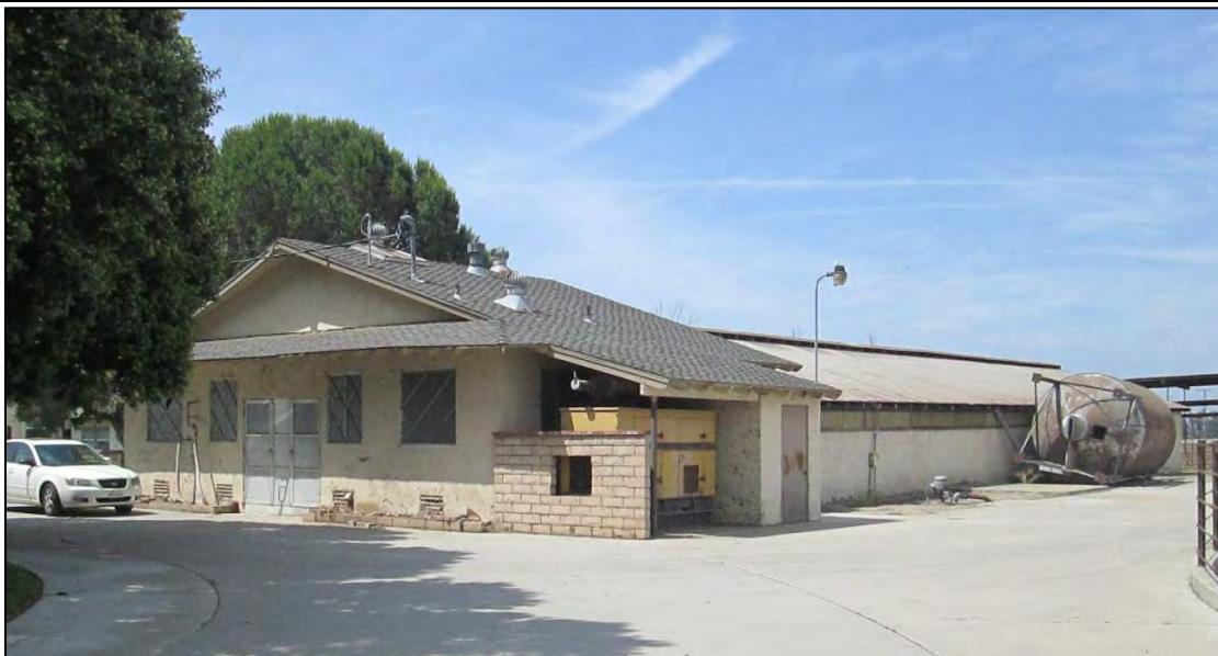
Dairy barn built for Harry Boersma Farm, bought by Borba in 1993. View looking west.
