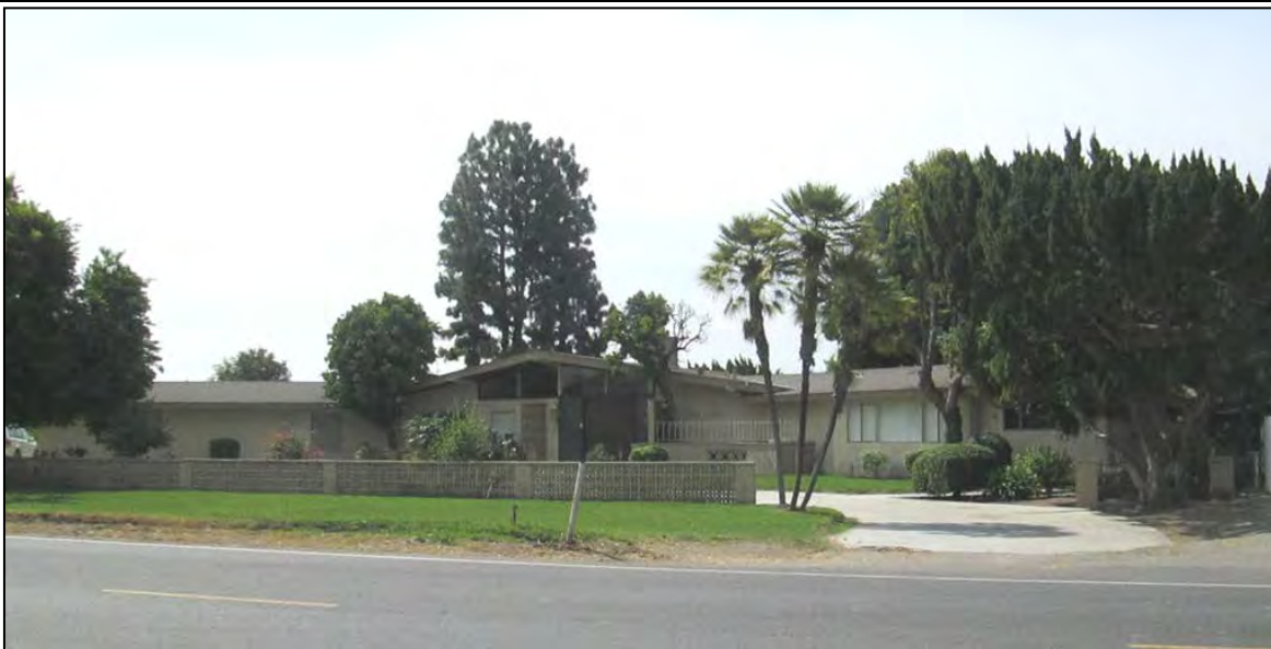
Borba Dairy Main House. View looking southeast.
