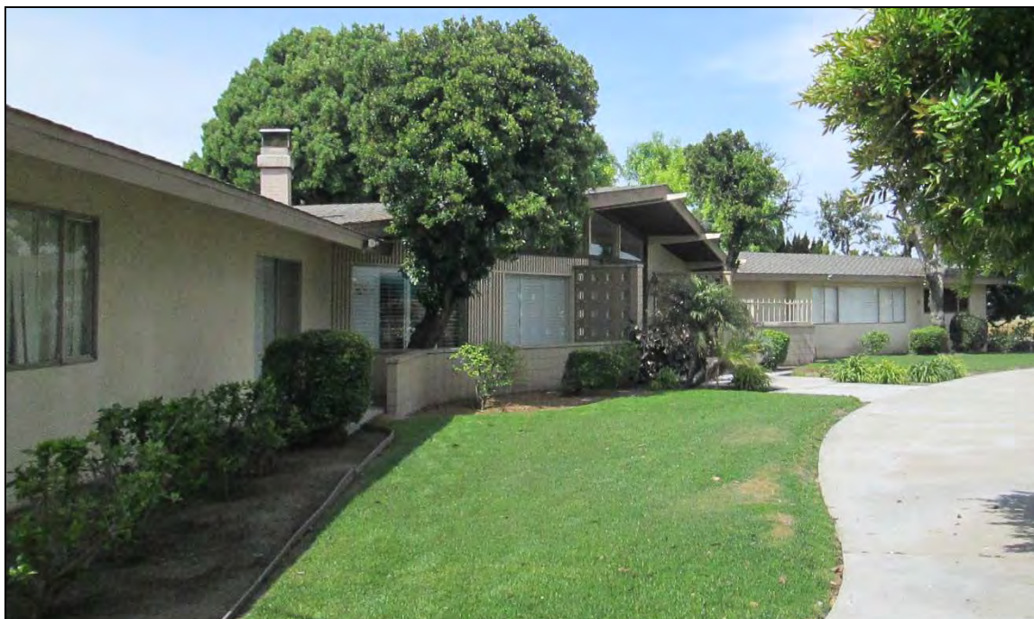
Borba Dairy Main House, front elevation. View looking west.
