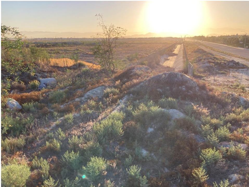
Photo 8: View of flood control channel located south of the Project Footprint, east of Haven Avenue; facing east. June 2022.
