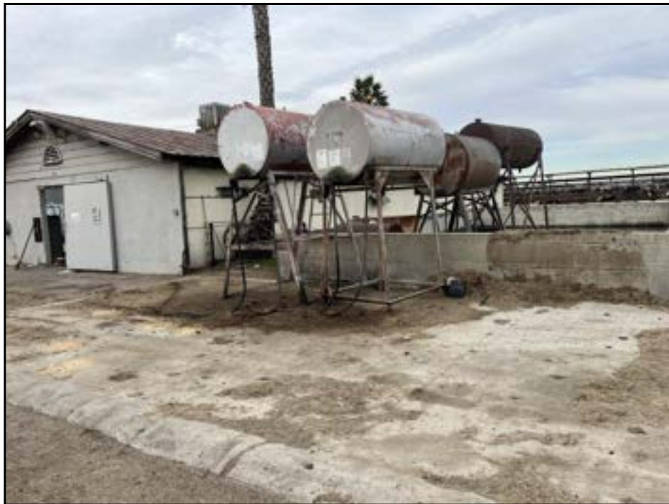
View of hazardous waste storage area in northeastern portion of Subject Property.
