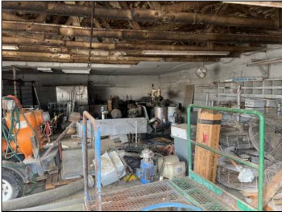
View of interior of maintenance/storage barn.
