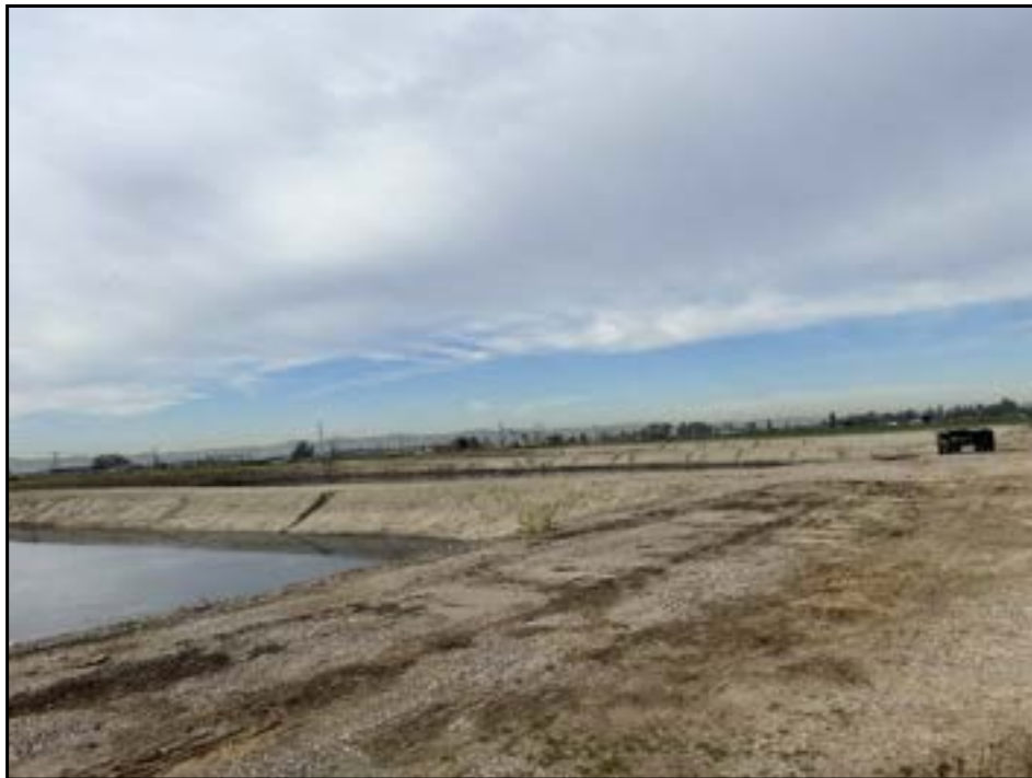
View of dairy ponds in southern portion of Subject Property.
