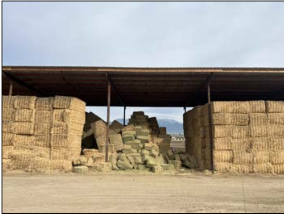
View of hay barn in northeastern portion of Subject Property.
