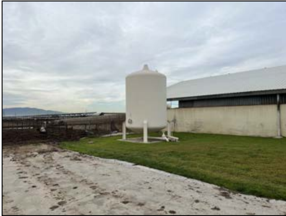
View of water holding tank adjacent to milk barn.
