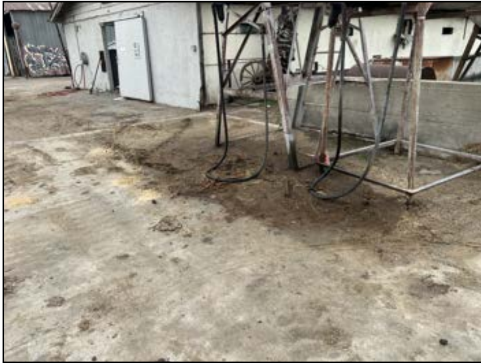
View of staining beneath ASTs adjacent to hazardous materials storage area.
