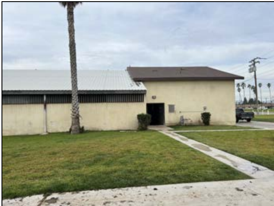
View of east side of milk barn (looking west).
