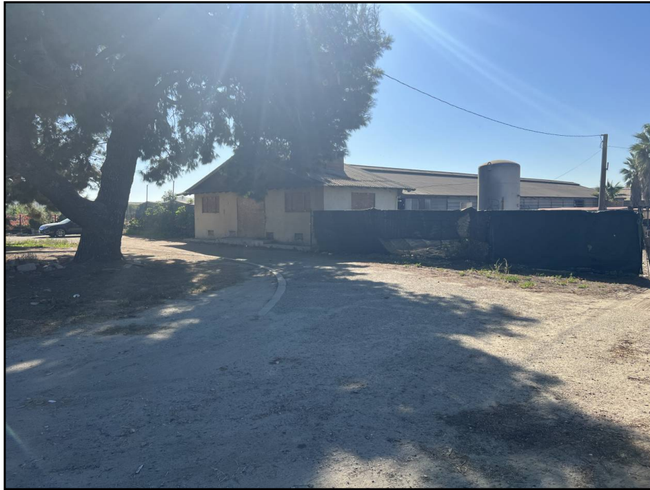
View of Subject Property (looking southeast) from East Riverside Drive.
