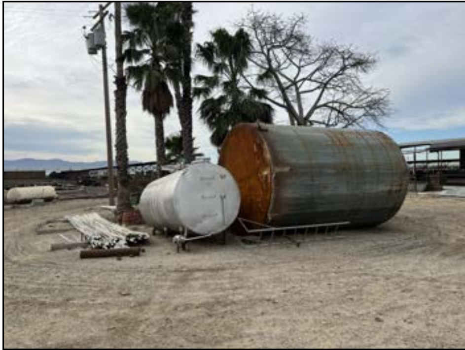
View of typical empty tanks observed on Subject Property.
