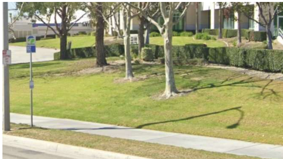
There is no landing pad or boarding area. No curb connection to the sidewalk.
