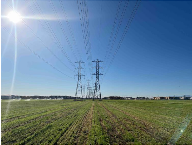
P-36-025440 Overview (View West)
