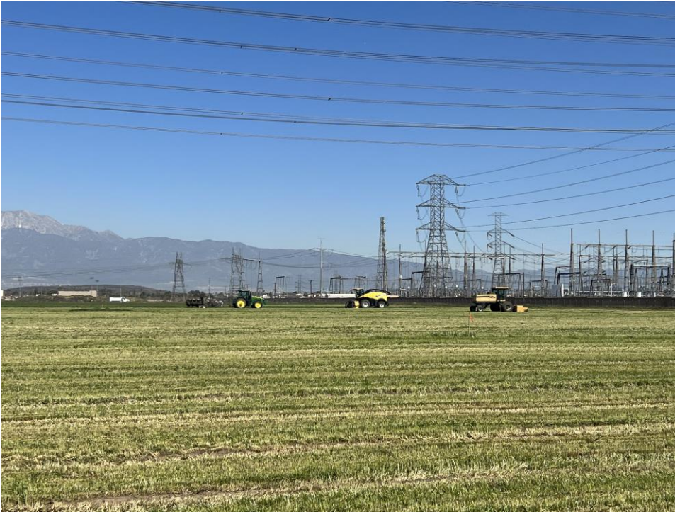
Photo 5: Southern Project Site Overview (View NE)
