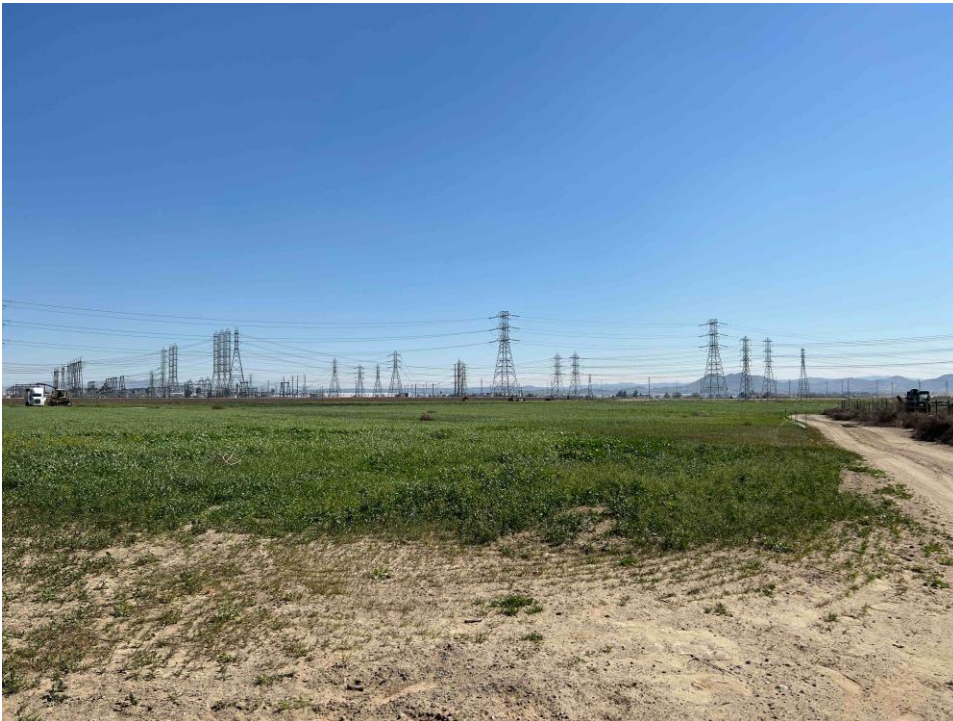
Photo 6: Northern Project Site Overview (View SE)
