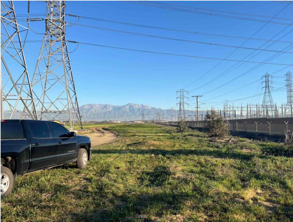
Photo 1: Southern Project Site Overview (View North)
