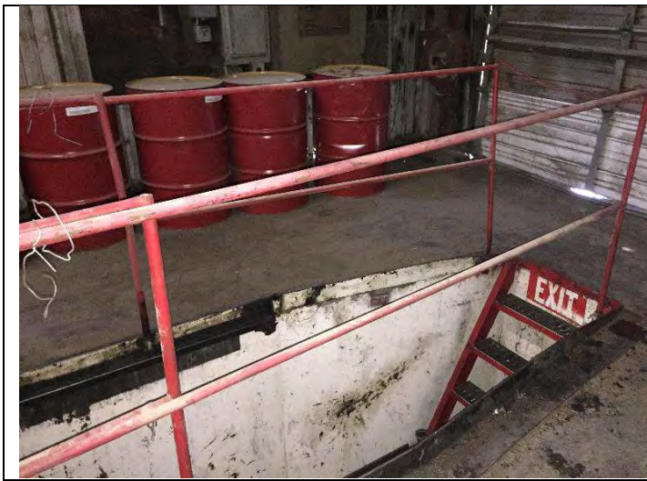
19. View of Service Pit within Building B
