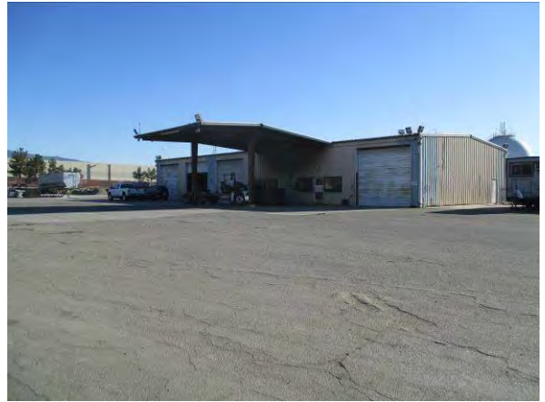
Photo #4 View of the truck repair shop building located on the eastern portion of the site.
