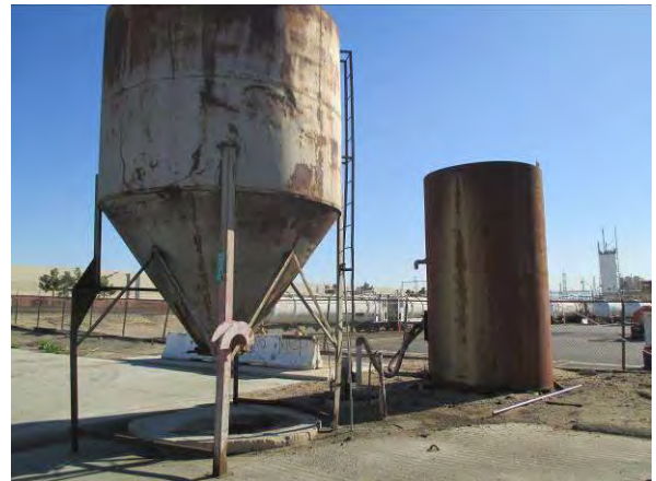
Photo #18 View of the sump and waste water storage for the former truck wash-down area.
