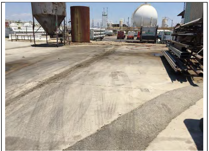
14. View of Former Vehicle Wash-Down Area
