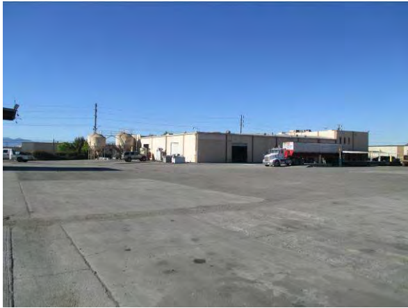
Photo #3 View of the office/warehouse building located on the southeastern portion of the site.
