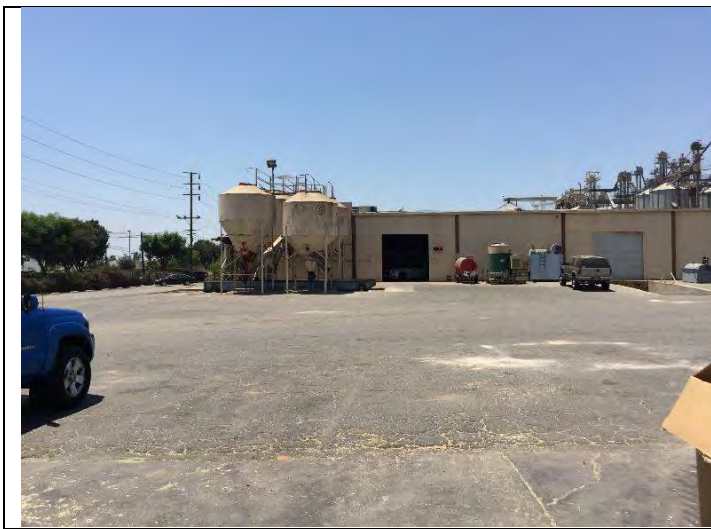
3. View of Main Building (Building A)
