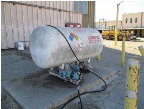
Photo #19 View of the propane AST located to the east of the mill.
