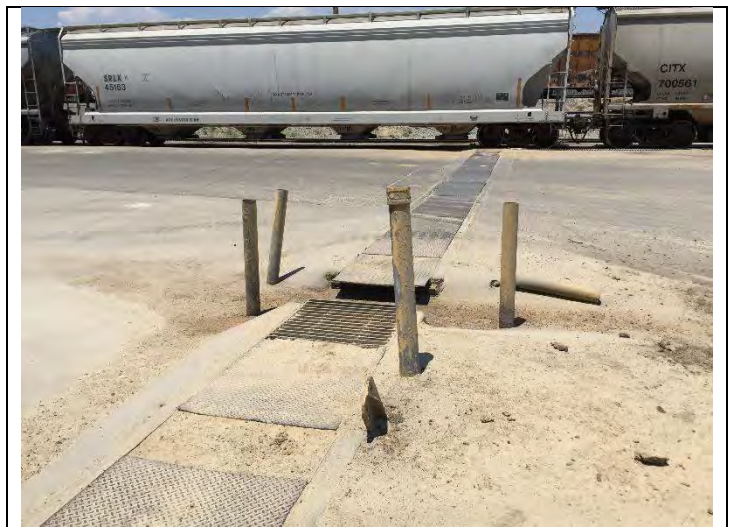
6. View of Grain Receiving Transfer Conveyor
