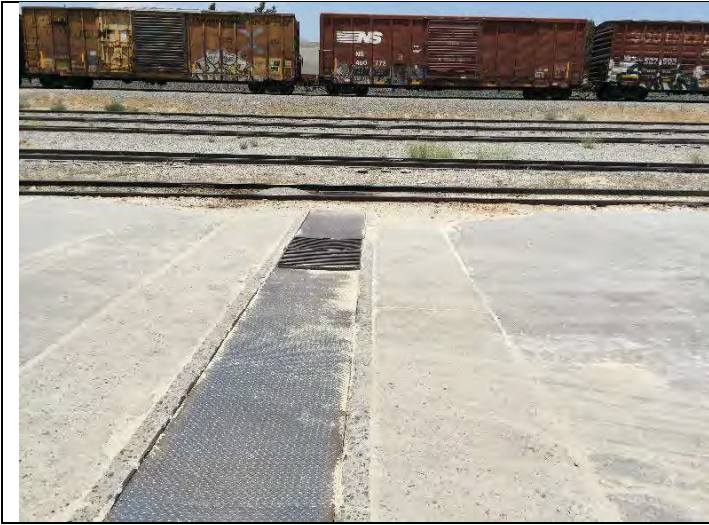
7. View of Grain Receiving Transfer Conveyor
