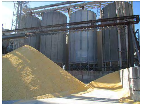
Photo #12 Typical view of the grain storage area.
