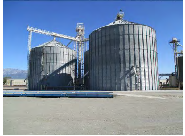
Photo #2 View of the large storage silos located on the western portion of the site.
