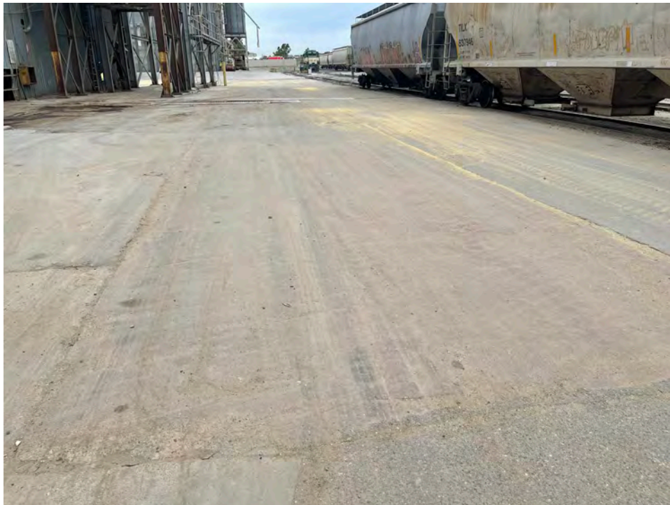
Photograph 8: Former underground storage tank area north of grain mill.
