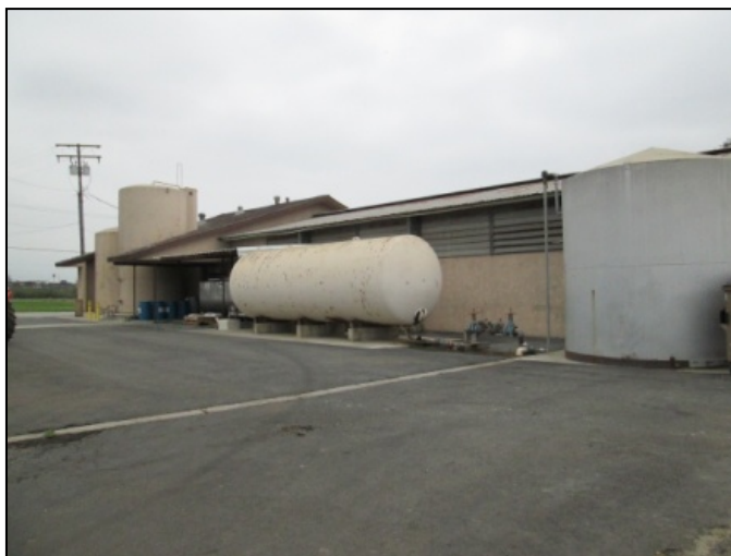
Dairy barn, west elevation. View looking northeast.
