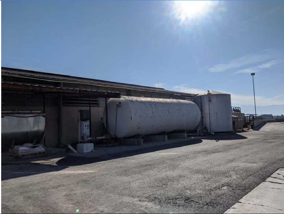
PHOTO 7: View of the water tanks, looking southeast.
