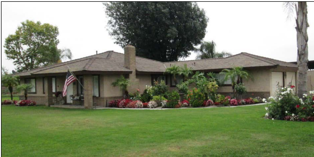
East House, north and west elevations. View looking southeast.
