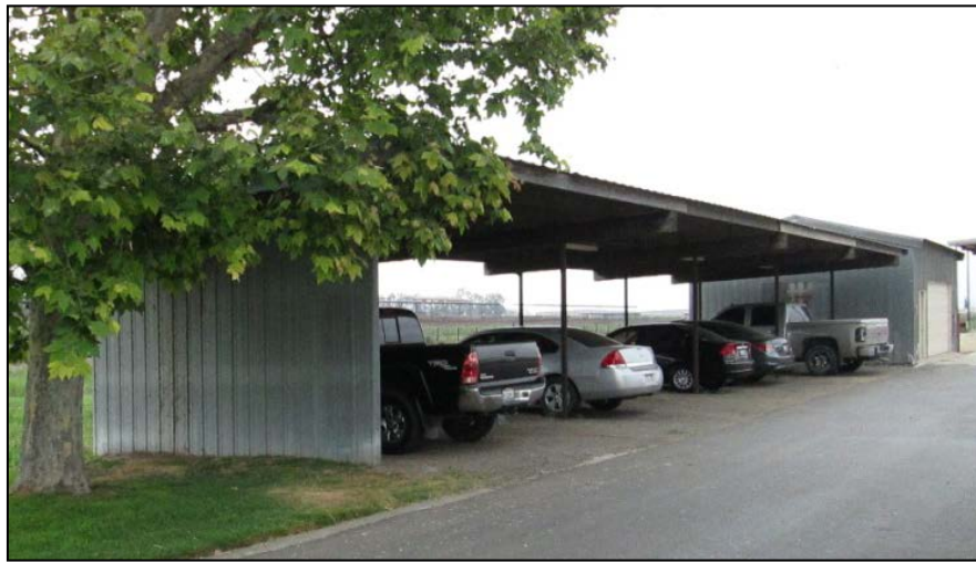
Covered carport. View looking southeast.
