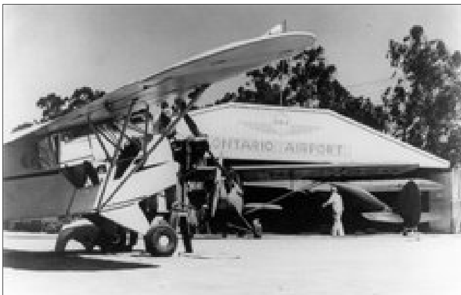
Figure 7. Ontario Airport, undated photo (City of Ontario 2018b)
