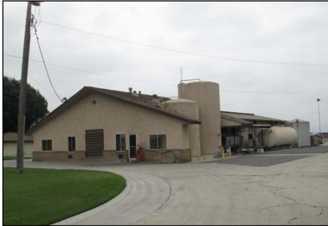
Dairy barn, north and west elevations. View looking south-southeast.
