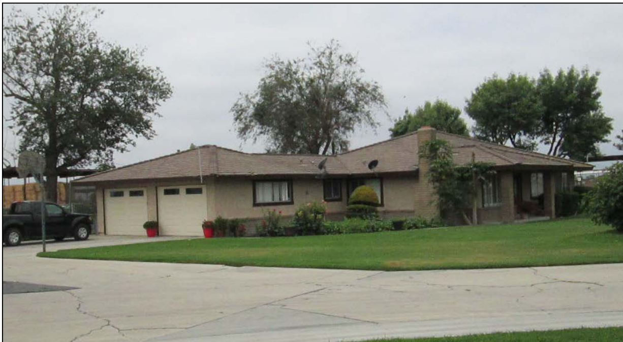
West House, north and east elevations. View looking southwest.
