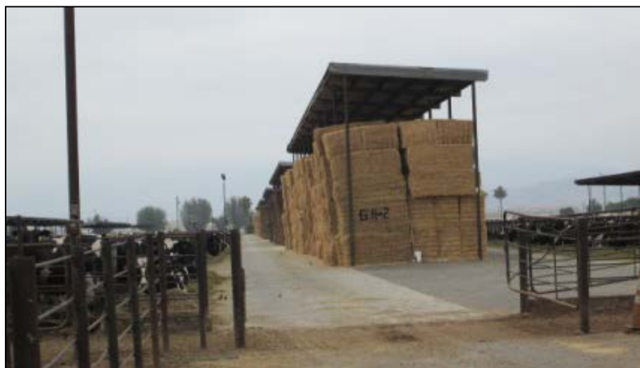
Hay storage sheds. View looking south.
