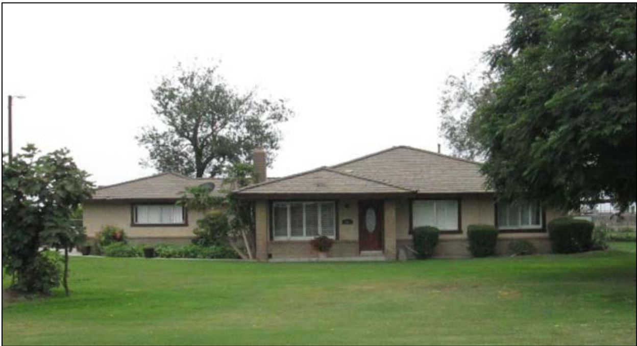
West House, front (north) elevation. View looking south.
