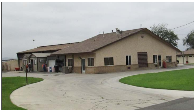
Dairy barn, north and east elevations. View looking southwest.
