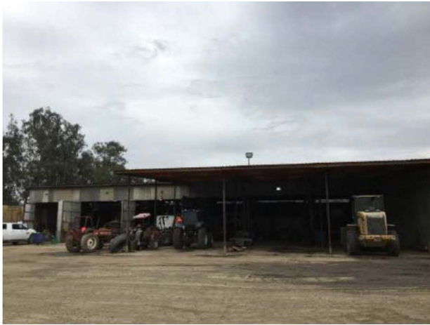
View of maintenance shop.
