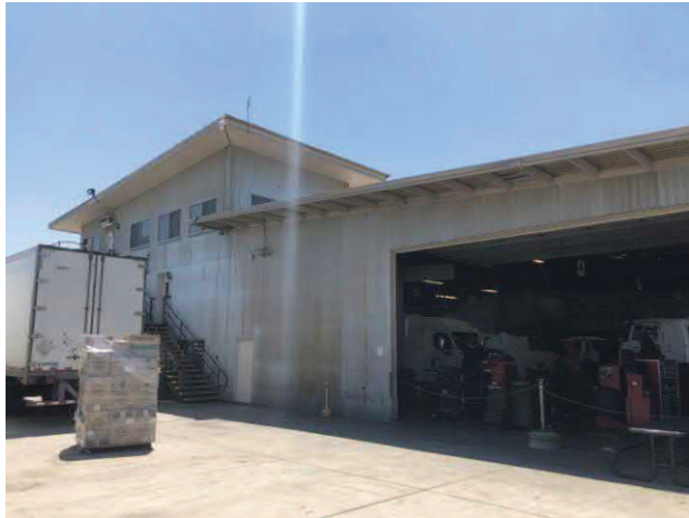
View of truck service building and office.
