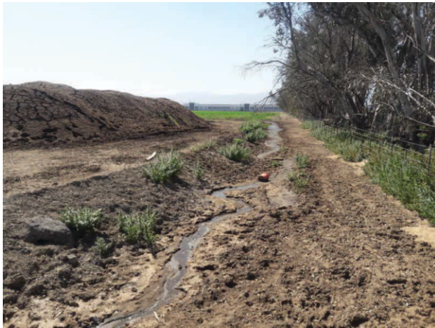
View of stormwater drainage swale.
