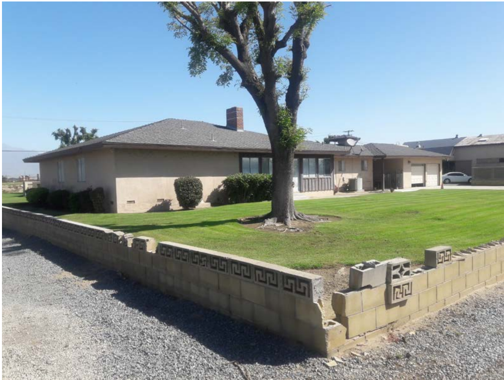
Photo #1: View of the residential structure located in the northern portion of the Subject Property.
