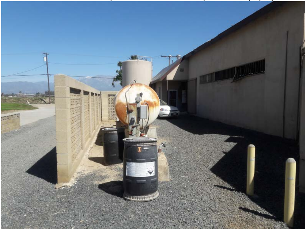
Photo #10: View of the well utilized for farming activities located on the western side of the northeastern milk barn and the diesel AST used for the water pump.
