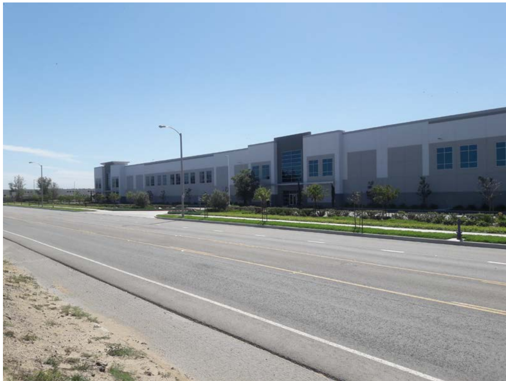
Photo #28: View of the adjoining property to the south.
