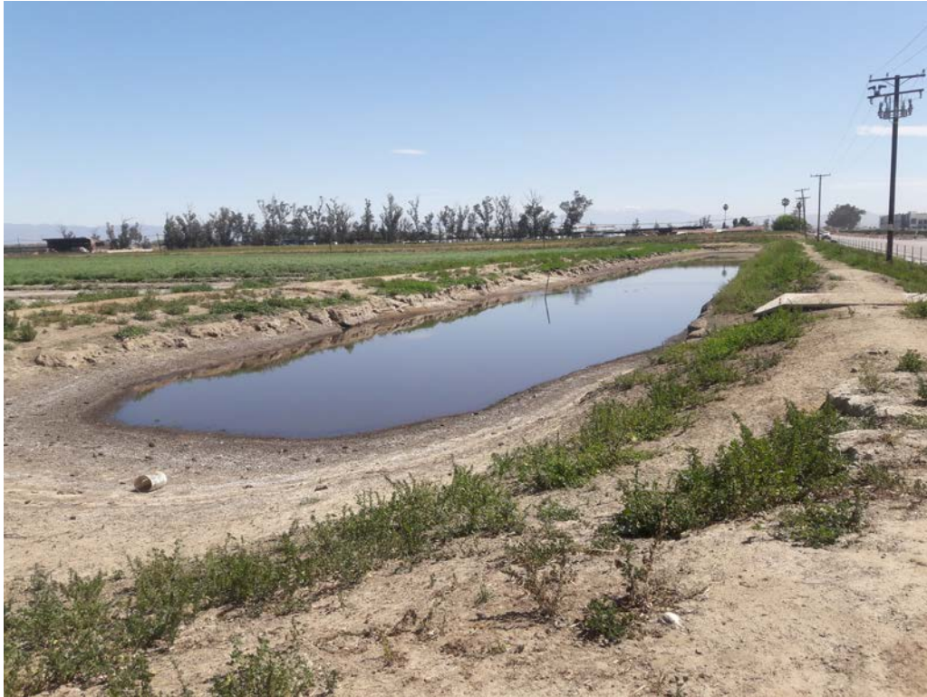
Photo #17: View of the wastewater lagoon located in the central portion of the Subject Property.
