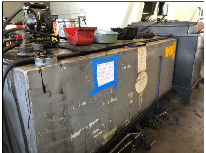
4. View of approximately 1,000-gallon waste oil AST.
