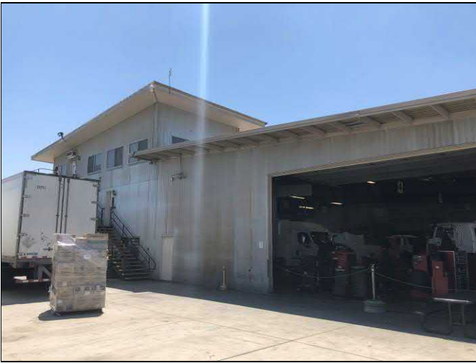
1. View of truck service building and office.
