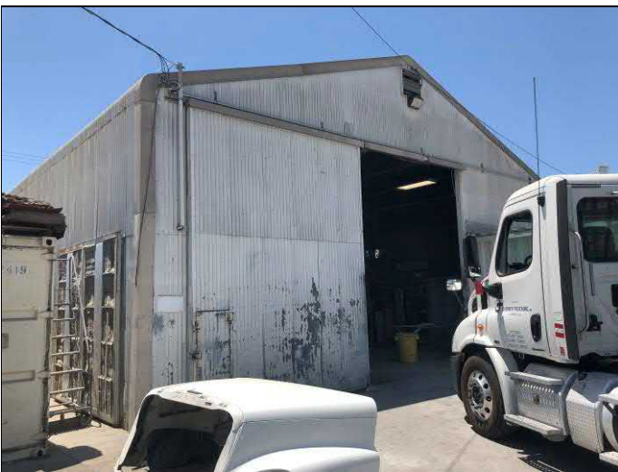
23. View of tool shop building.
