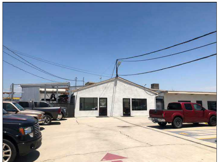
18. View of administrative building.
