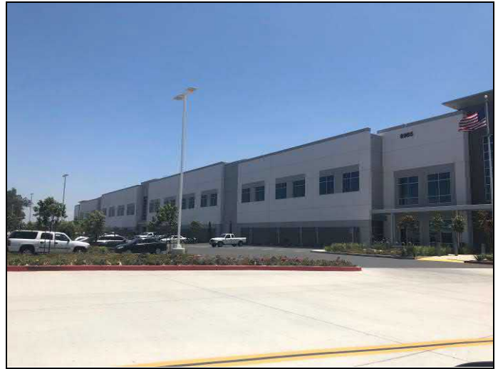
8. View of south-adjacent industrial warehouse (8985 Merrill Avenue).
