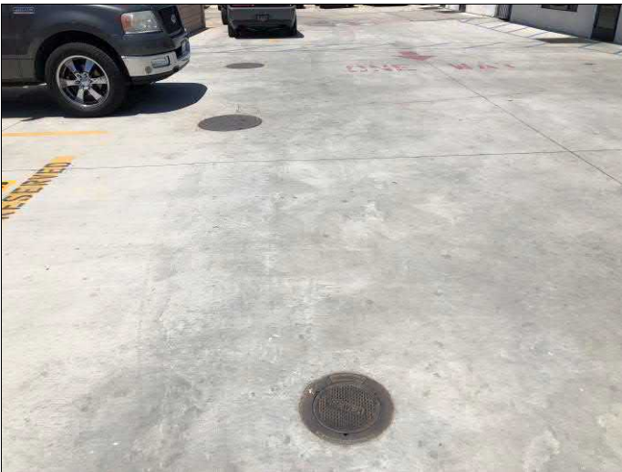
21. View of septic system by administrative building.
