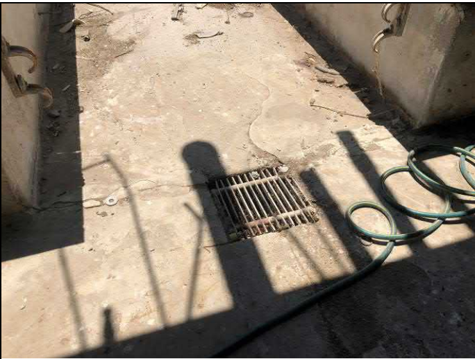
3. View of floor drain in former milking area.
