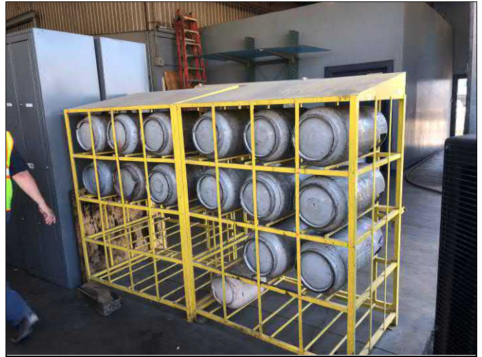
14. View of propane canisters for forklift operation.
