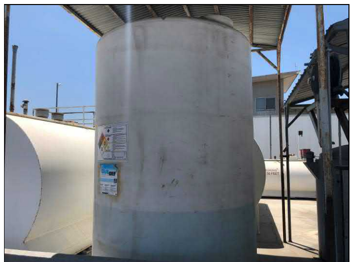
36. View of Blue Def silo AST (approximately 5,000-gallon).
