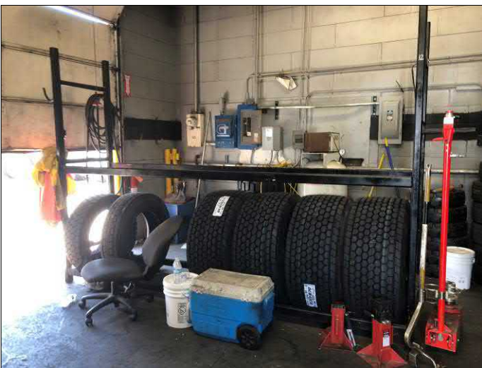
29. Additional tire shop interior view.
