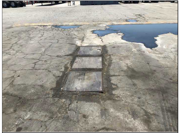
32. View of three-chamber clarifier in truck washing area.
