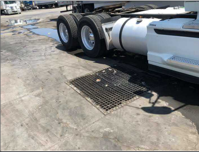
31. View of drain in truck washing area.
