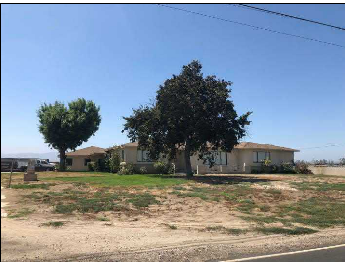
5. View of single-family residence on property.
