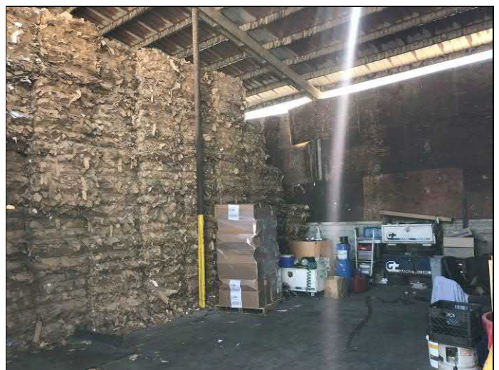
42. View of paper product storage shelter.
