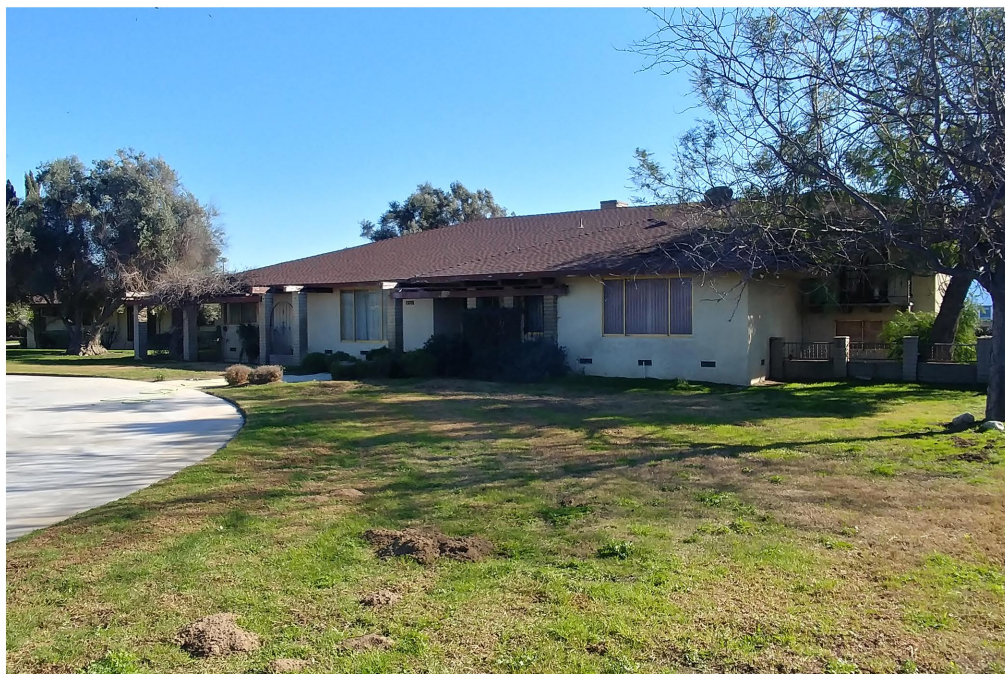
Plate 3.2–20: Overview of the Site Temp-6 residence at 8731 Eucalyptus Avenue, facing southeast.
