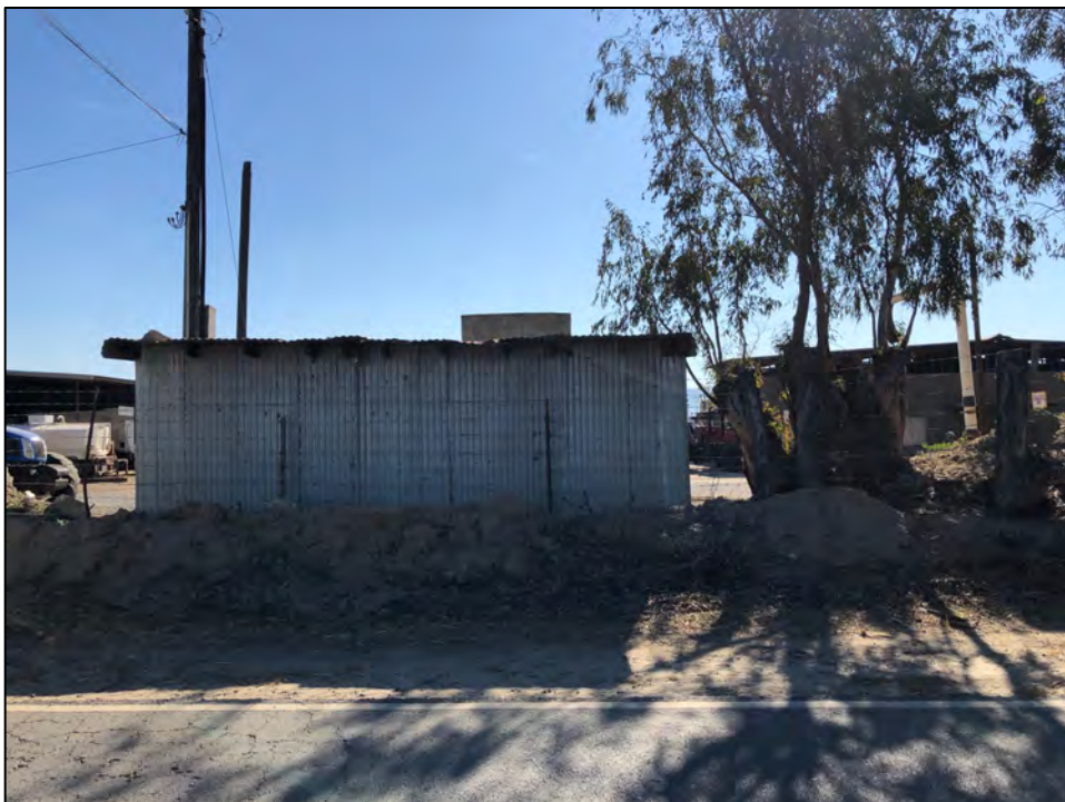
View south of ancillary shed at 8321 Eucalyptus Ave, with office on right, January 2020. Source: Urbana Preservation & Planning, LLC.
