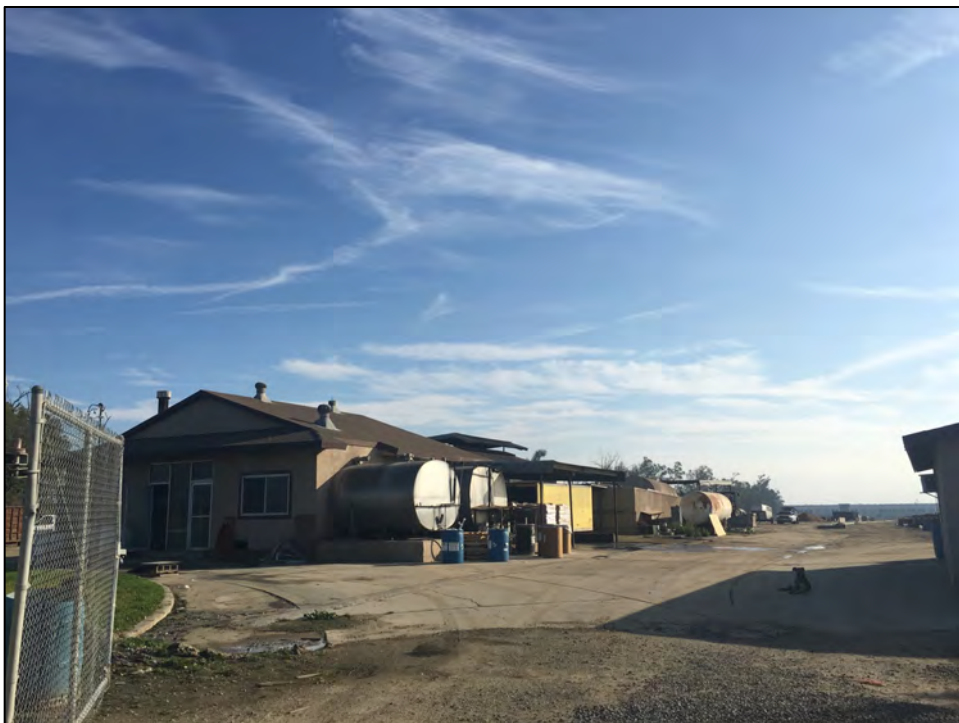
View southeast of Milking Parlor, with 8521 Eucalyptus Ave on right, January 2020 Source: Urbana Preservation & Planning, LLC.
