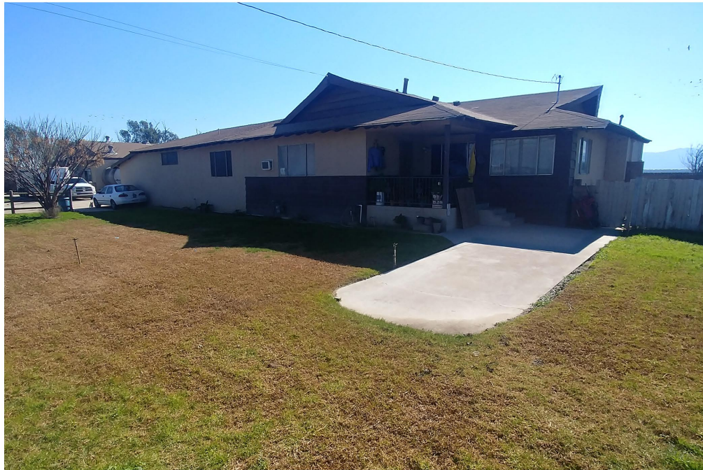
Plate 3.2–16: Overview of Site Temp-2 at 8521 Eucalyptus Avenue, facing southeast.
