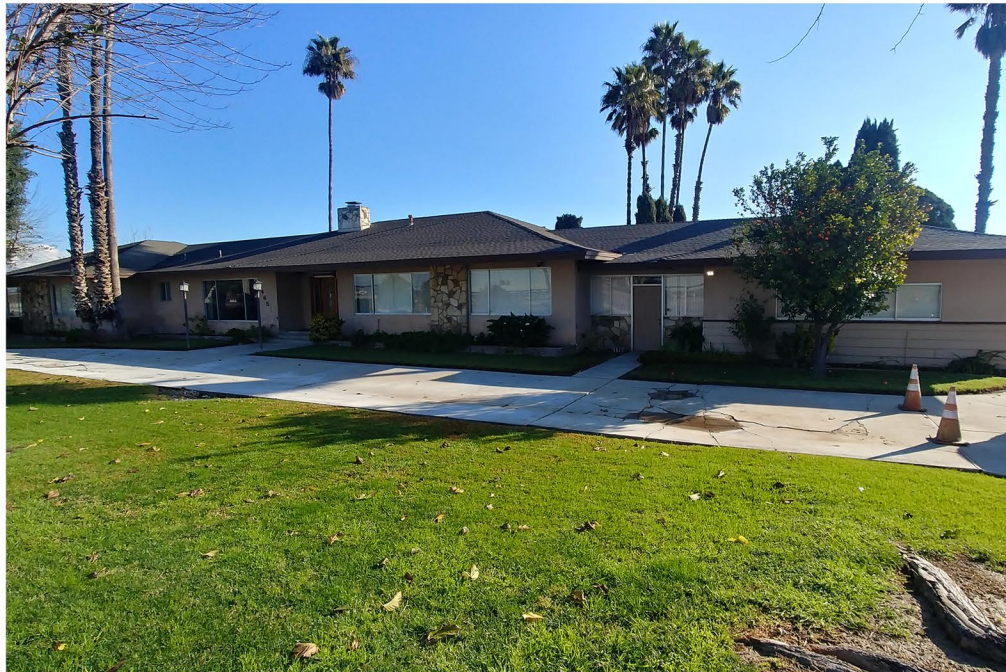
Plate 3.2-31: Overview of the Site Temp-15 residence at 14651 Grove Avenue, facing east.
