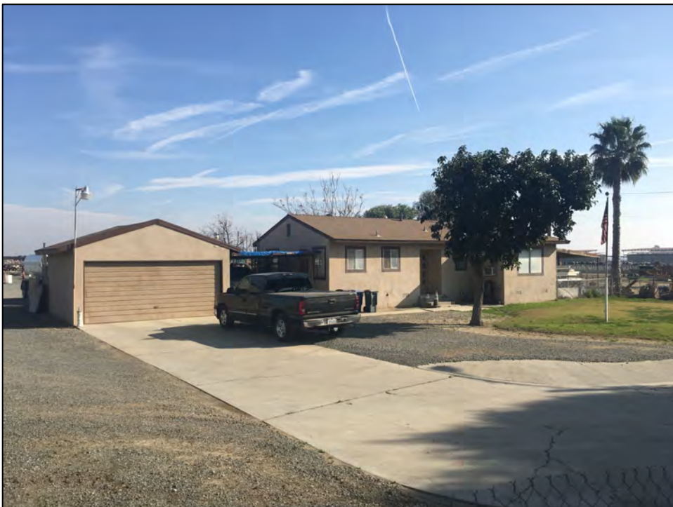
View southeast of 14525 Grove Avenue, single-family residence and garage, January 2020. Source: Urbana Preservation & Planning, LLC.
