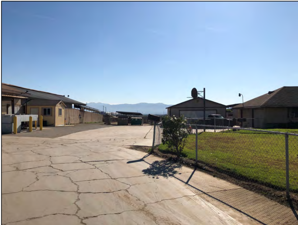
View south of parcel with pole structures in background, view between Milking Parlor (on left) and 8477 Eucalyptus Ave (on right), January 2020. Source: Urbana Preservation & Planning, LLC.
