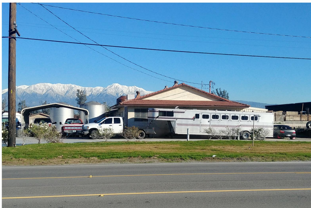
Plate 3.2–30: Overview of the Site Temp-14 milk barn at 8920 Merrill Avenue, facing north.
