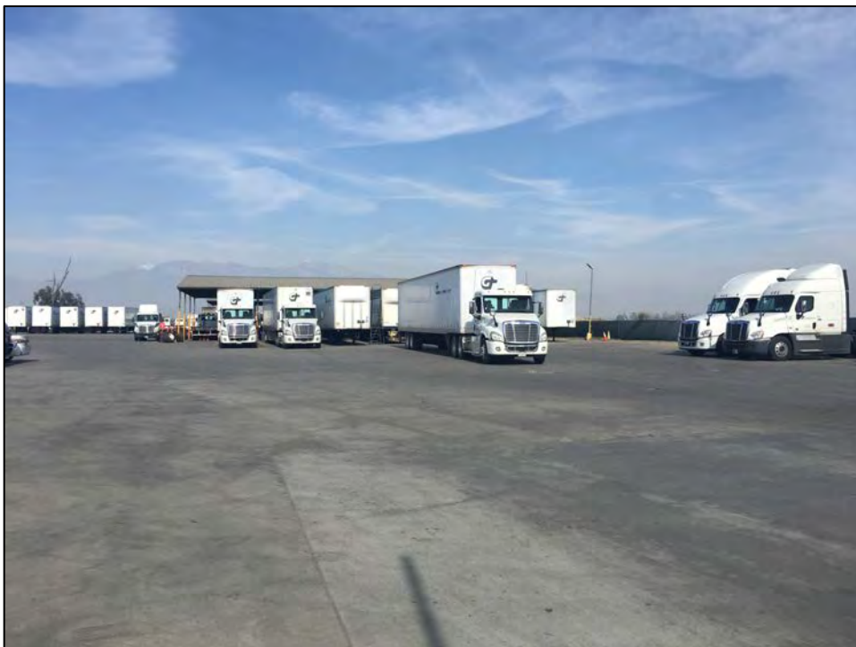
View north of Transportation Facility, including pole structure (in background), January 2020. Source: Urbana Preservation & Planning, LLC.
