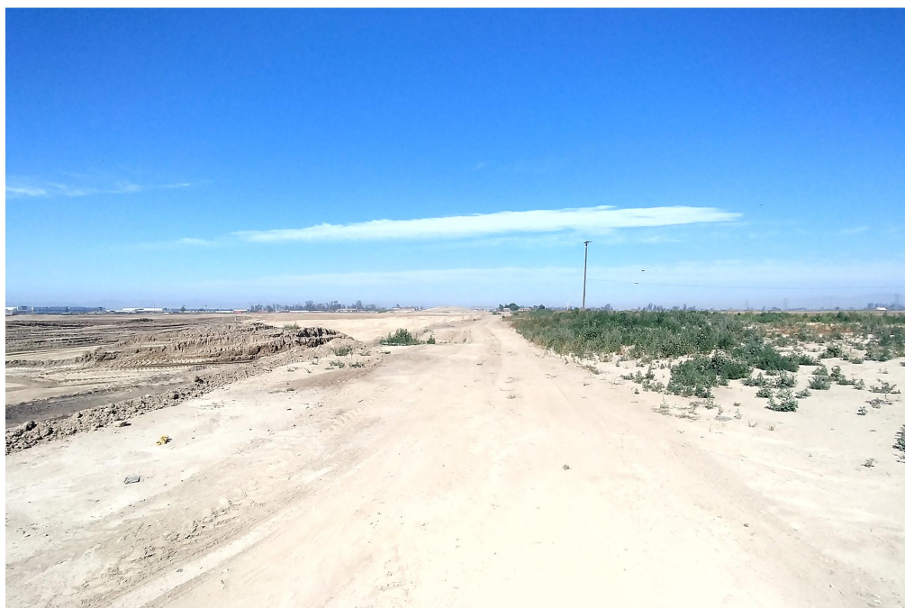
Plate 3.2-12: Overview of the off-site portion of Eucalyptus Avenue within the project, facing west.
