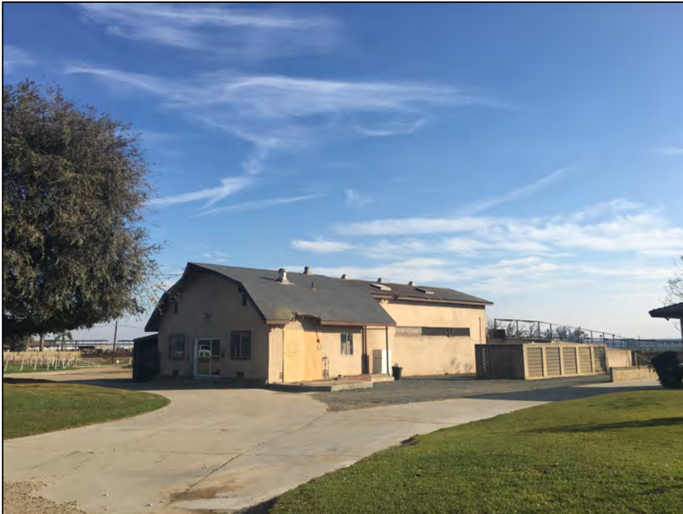
View southeast of Milking Parlor associated with 8643 Eucalyptus Ave, January 2020. Source: Urbana Preservation & Planning, LLC.
