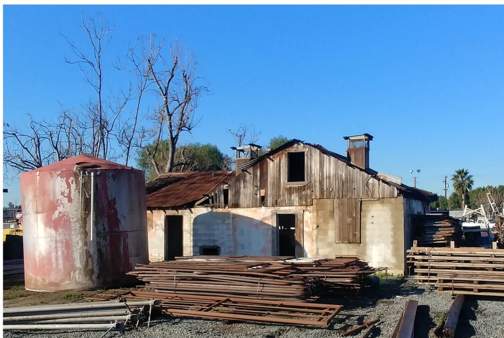
Plate 3.2–35: Overview of the Site Temp-17 barn at 14525 Grove Avenue, facing southwest.
