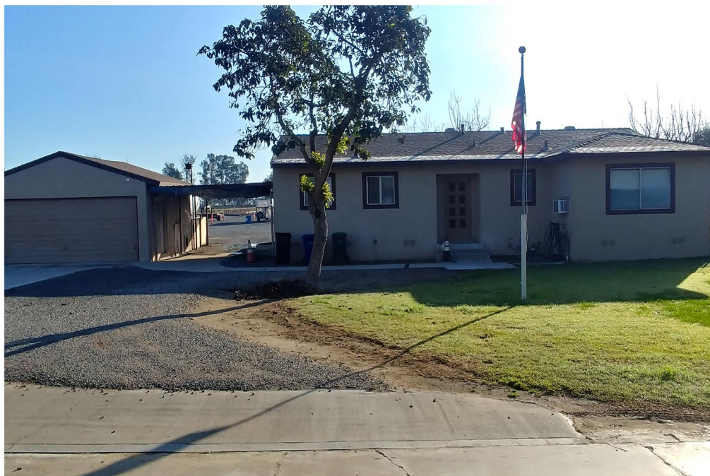
Plate 3.2–34: Overview of the Site Temp-17 residence at 14525 Grove Avenue, facing east.
