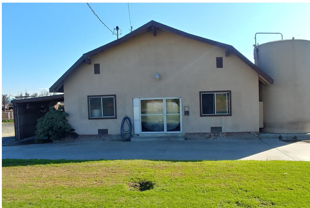
Plate 3.2–19: Overview of Site Temp-5 at 8643 Eucalyptus Avenue, facing south.
