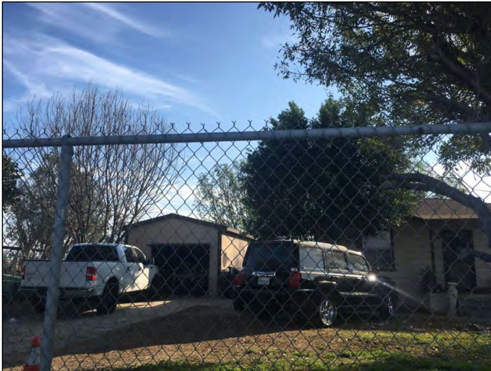
View southeast of 8551 Eucalyptus Avenue and garage, January 2020. Source: Urbana Preservation & Planning, LLC.
