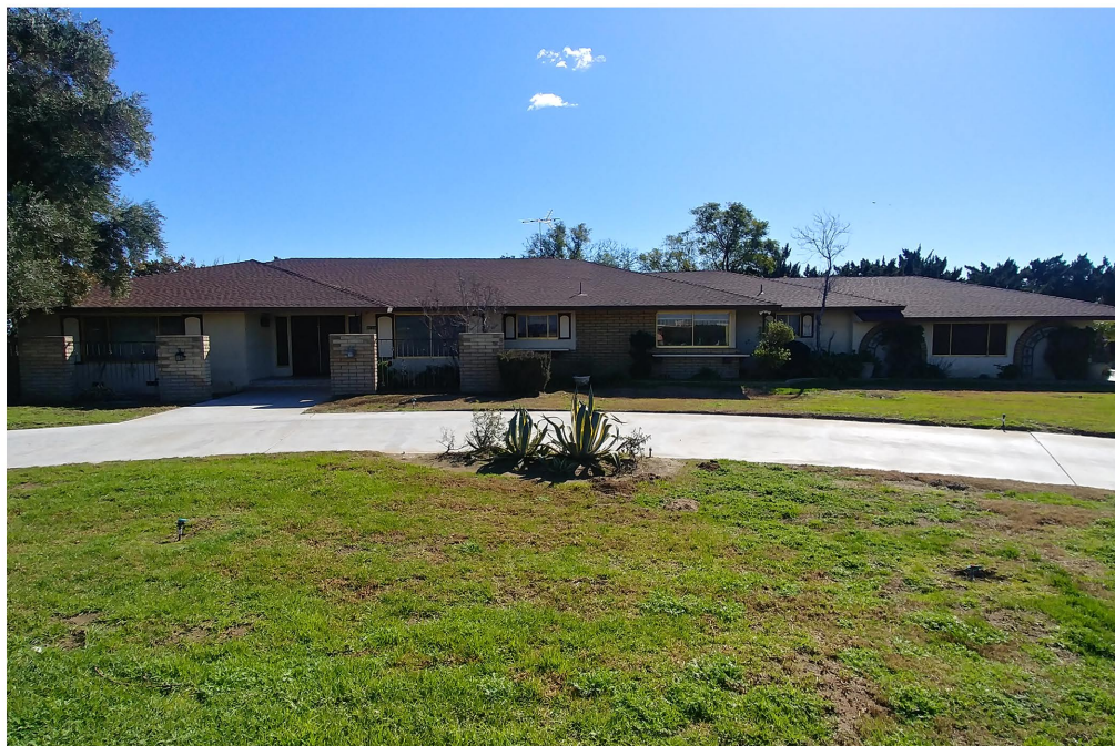
Plate 3.2–23: Overview of Site Temp-8 at 8888 Eucalyptus Avenue, facing south.
