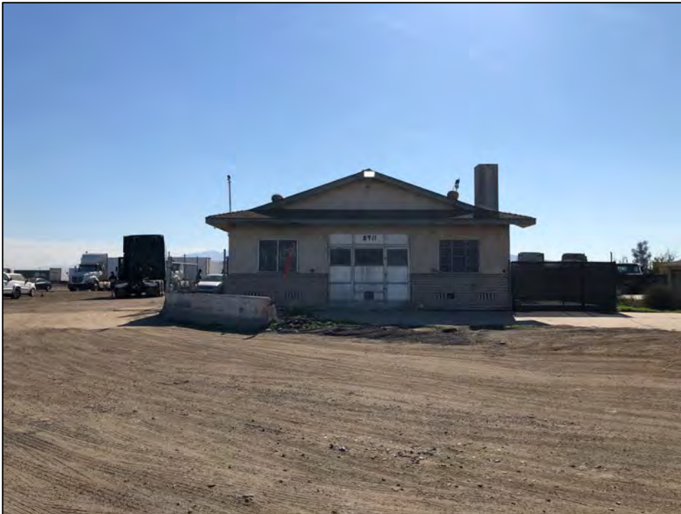
View south of Milking Parlor at 8911 Eucalyptus Ave, January 2020. Source: Urbana Preservation & Planning, LLC.
