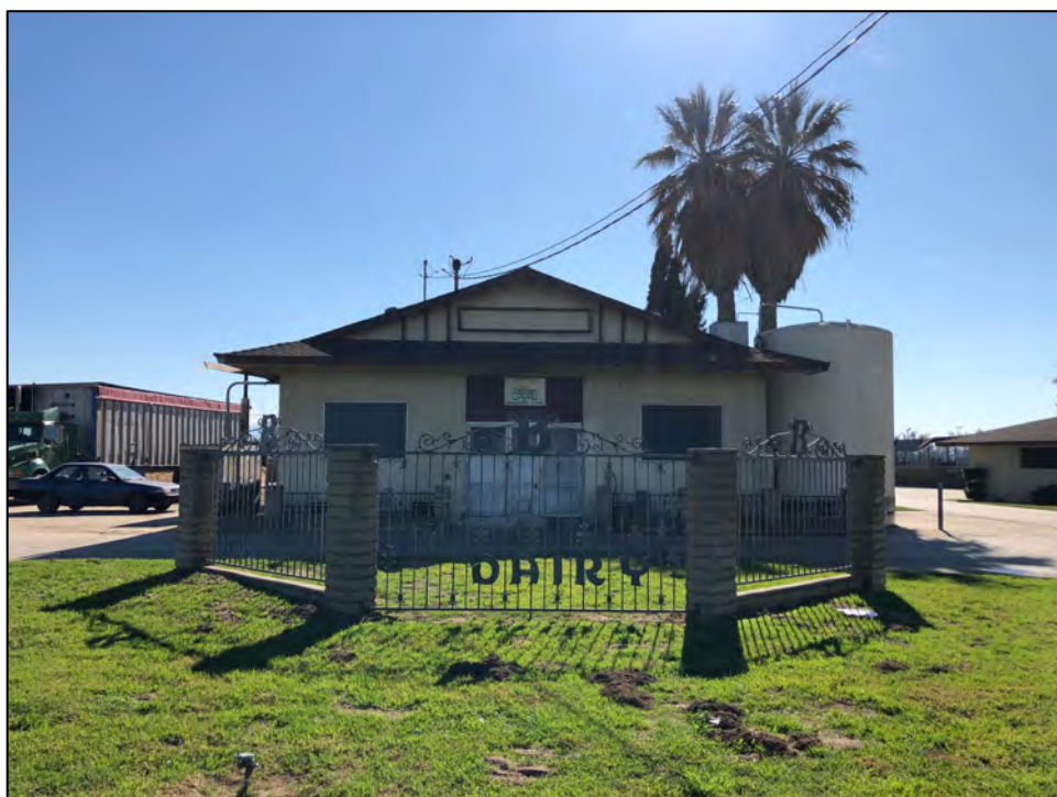
View south of Milking Parlor, January 2020. Source: Urbana Preservation & Planning, LLC.
