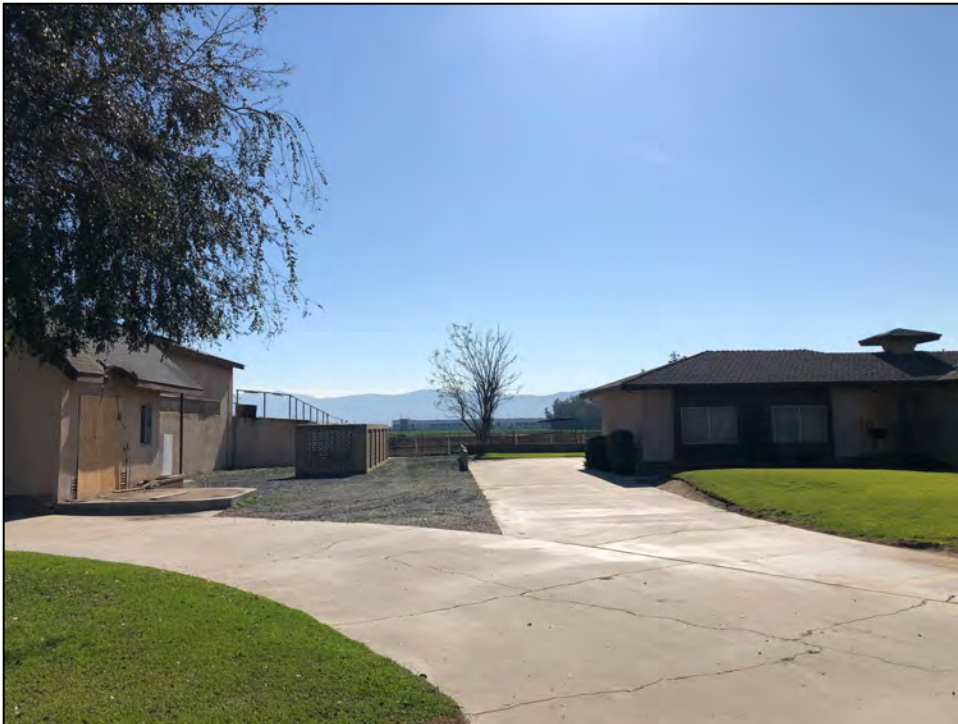
View south of parcel, view between 8643 Eucalyptus Ave (right) and its associated Milking Parlor (left). Source: Urbana Preservation & Planning, LLC.
