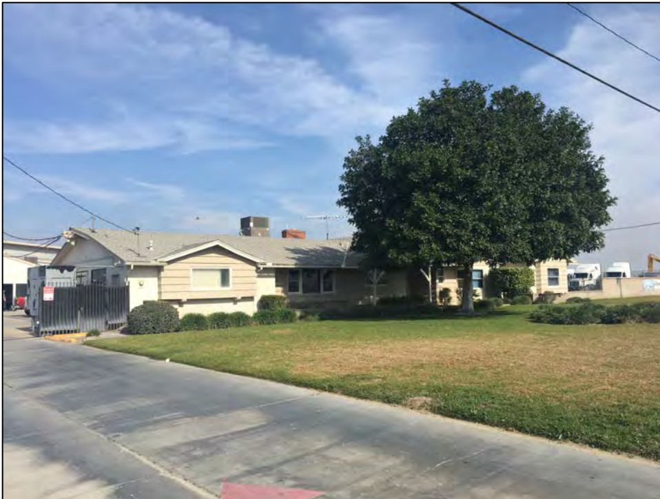
View northeast of 9032 Merrill Ave, January 2020. Source: Urbana Preservation & Planning, LLC.
