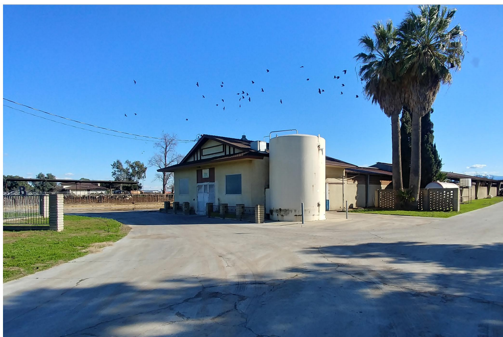
Plate 3.2–21: Overview of the Site Temp-6 milk barn at 8731 Eucalyptus Avenue, facing southeast.
