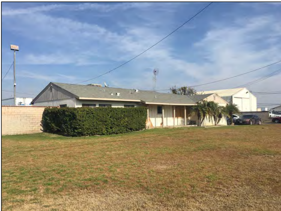
View northeast of 8966 Merrill Ave (south façade and east elevation), January 2020. Source: Urbana Preservation & Planning, LLC.
