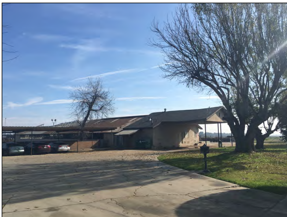
View southeast of Milking Parlor, January 2020. Source: Urbana Preservation & Planning, LLC.
