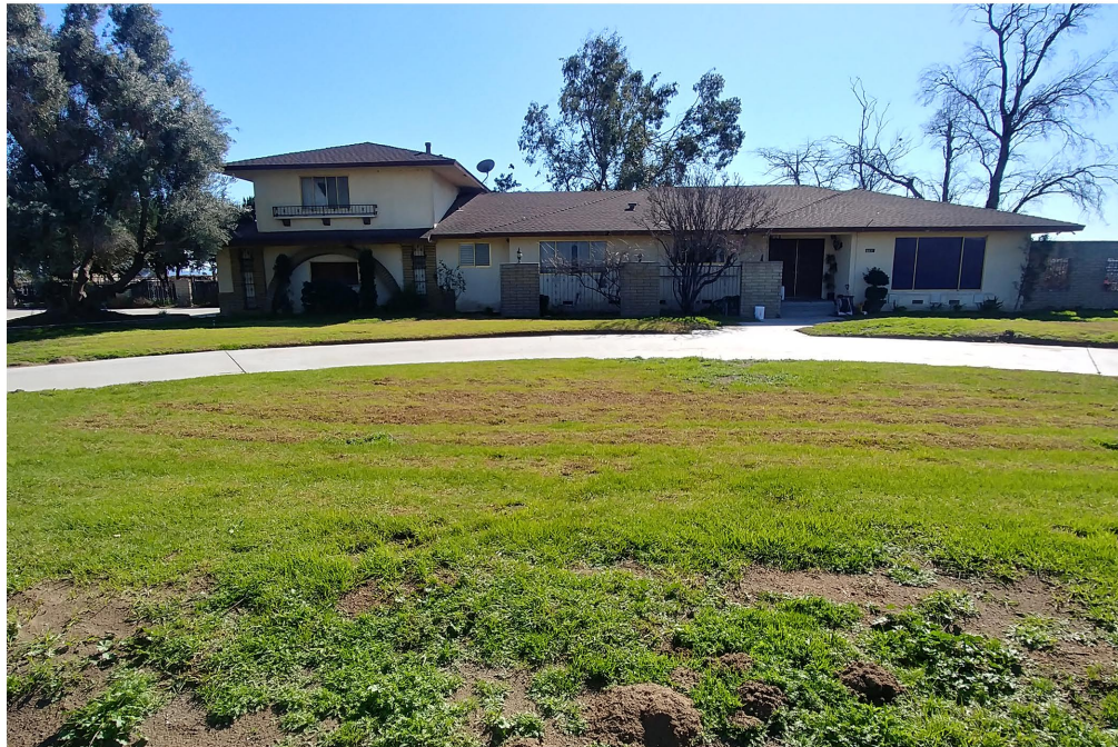
Plate 3.2–22: Overview of Site Temp-7 at 8831 Eucalyptus Avenue, facing south.
