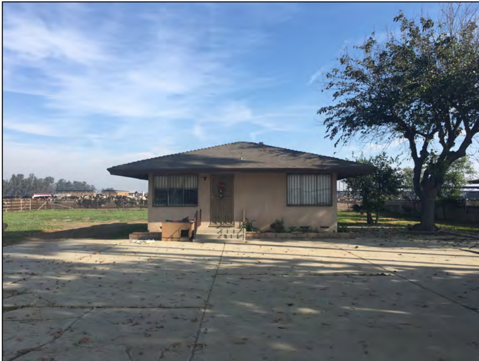
View east of 14545 Grove Avenue, January 2020. Source: Urbana Preservation & Planning, LLC.
