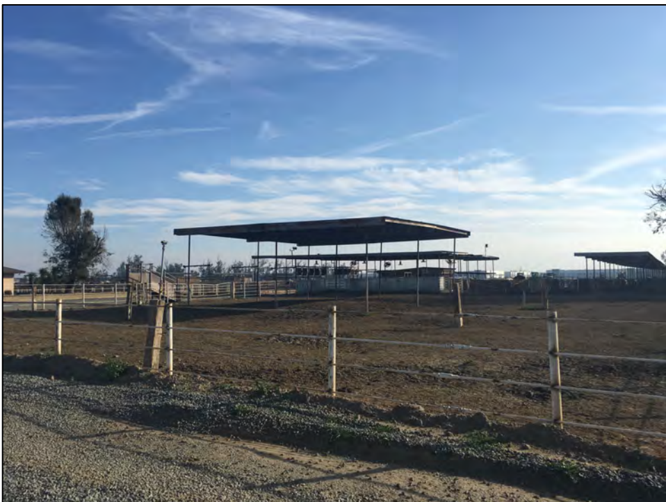
View southeast of pole structures, west of 8643 Eucalyptus Ave, January 2020. Source: Urbana Preservation & Planning, LLC.
