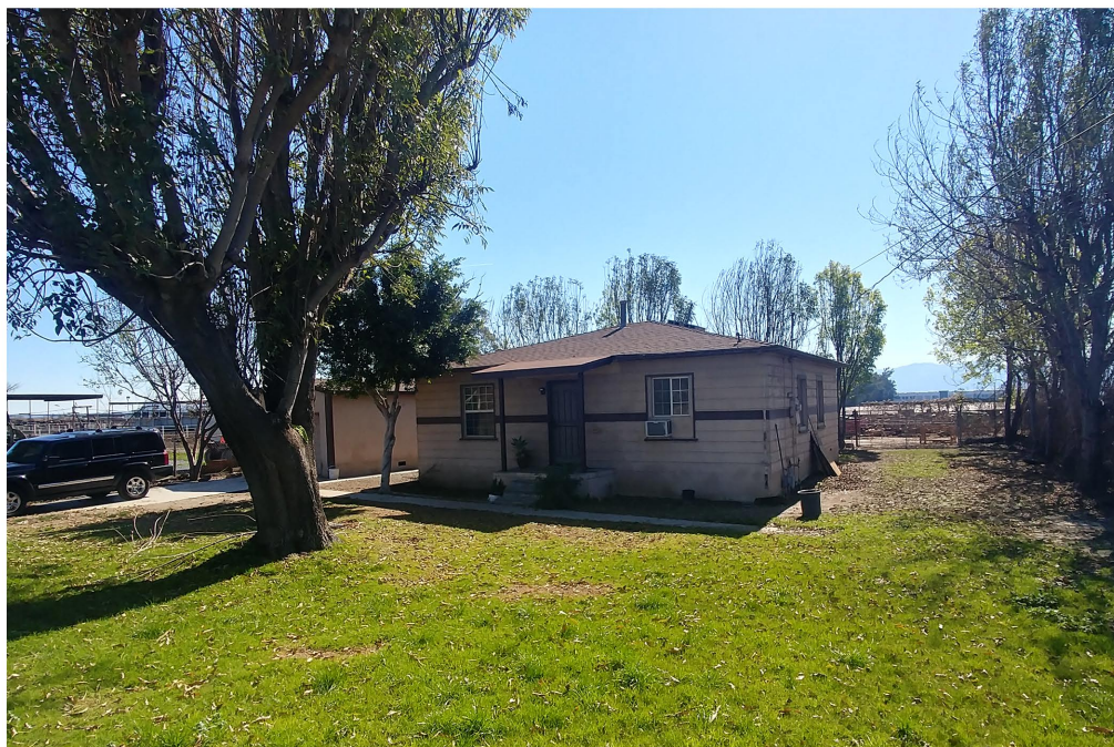
Plate 3.2–18: Overview of Site Temp-4 at 8551 Eucalyptus Avenue, facing southeast.
