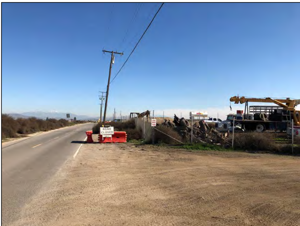
View east of Eucalyptus Ave road closure sign, with Trucking Facility on right, January 2020. Source: Urbana Preservation & Planning, LLC.
