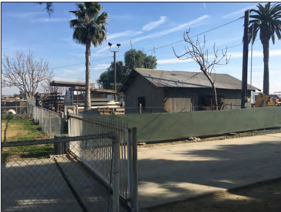
View southeast of ancillary shed, north and west facades, January 2020. Source: Urbana Preservation & Planning, LLC.
