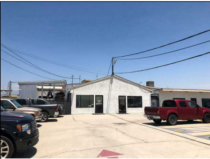
29. View of west-adjacent Gardner Trucking/Fleet Yards Inc. (9032 Merrill Avenue/8911 Eucalyptus)
