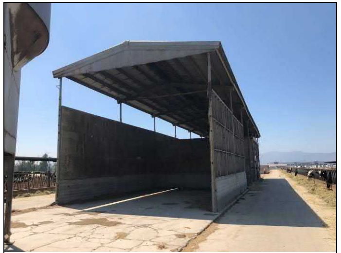
16. View of additional hay storage structure.
