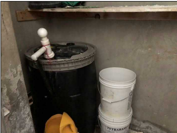
9. View of 55-gallon muriatic acid storage for line cleaning.
