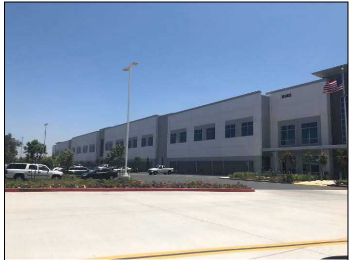
28. View of south-adjacent industrial warehouse (8985 Merrill Avenue).
