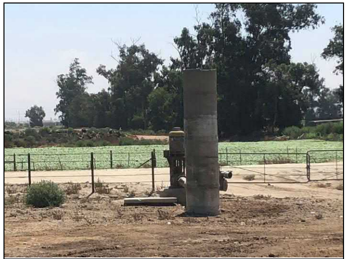
18. View of electric-powered irrigation well.
