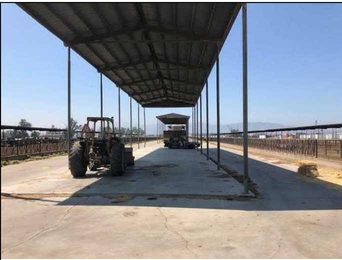
15. View of hay storage structure.
