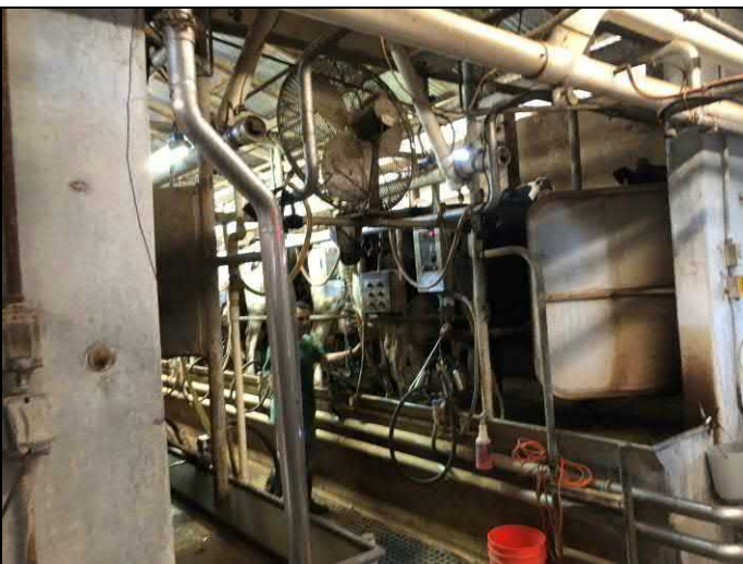
5. View of milking equipment.
