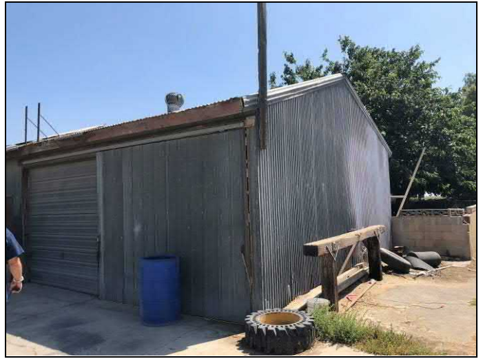
14. View of storage building.
